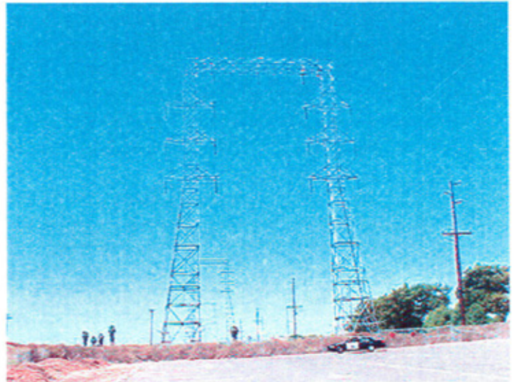
Photo 5: Tower 13, E Street and Bay Boulevard Looking North
