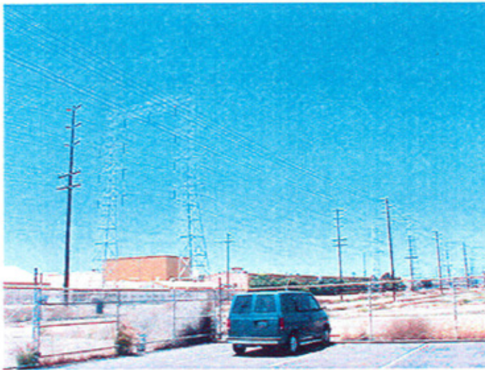
Photo 2: Tower 5, I Street and Bay Boulevard Looking Northwest
