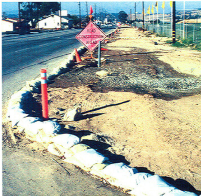
Sand bags used as perimeter control.
