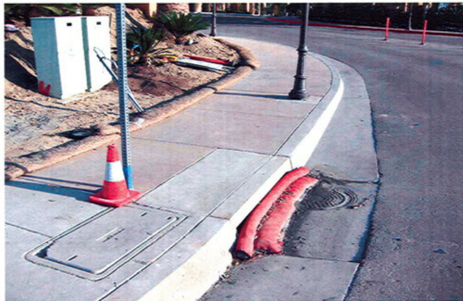
Inlet protection that blocks flow is good for preventing non-storm water discharges from entering the drain.
