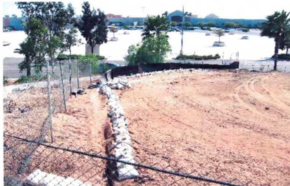
Gravel bags used as perimeter control.
