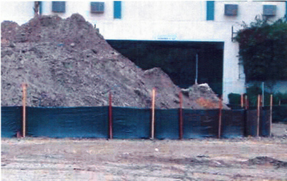
Silt fence used for stockpile perimeter control.
