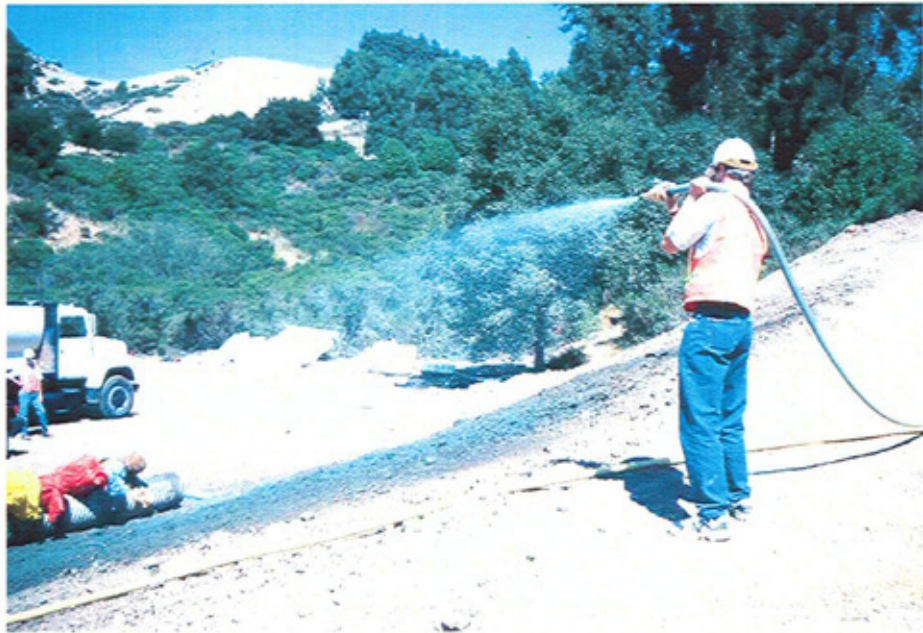
Applying hydroseed.
