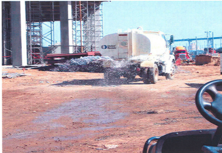
Water being applied for dust control.
