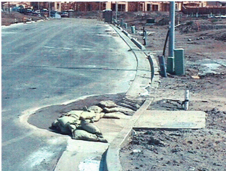
Gravel bag inlet protection.
