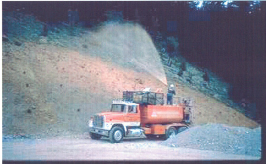
Applying hydraulic mulch.
