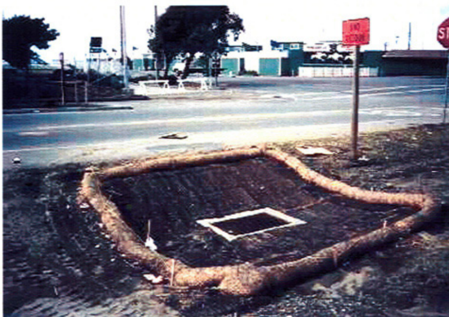
Inlet protection using fiber rolls and filter fabric.
