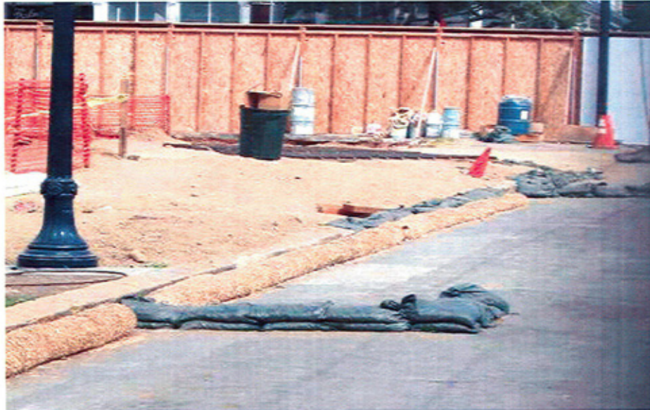
Gravel bags and fiber rolls used as a perimeter sediment control system.
