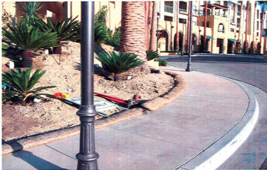
Fiber rolls as perimeter control
