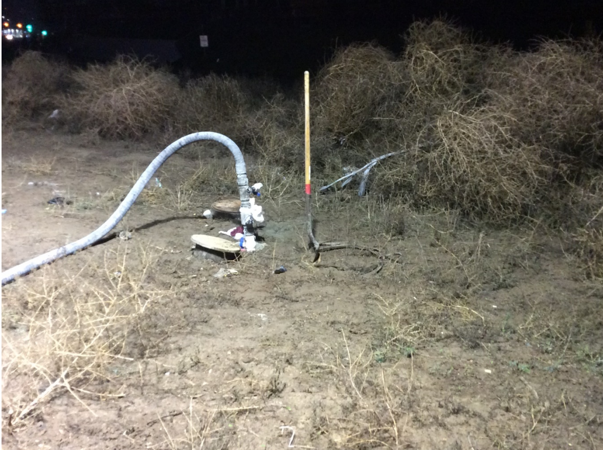
Figure 5: Grout Filling the Abandoned Pipeline
