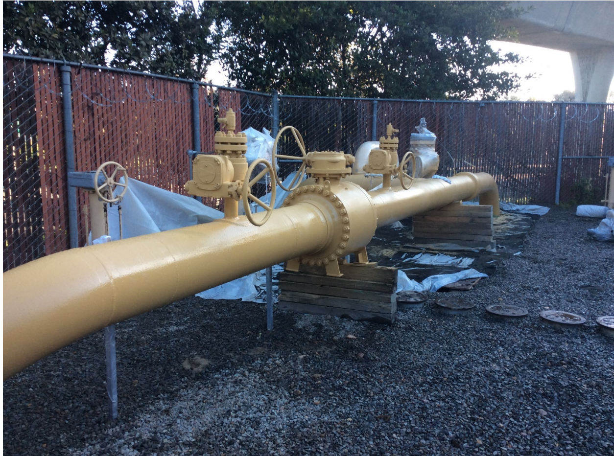
Figure 5: New Above Grade MLV
