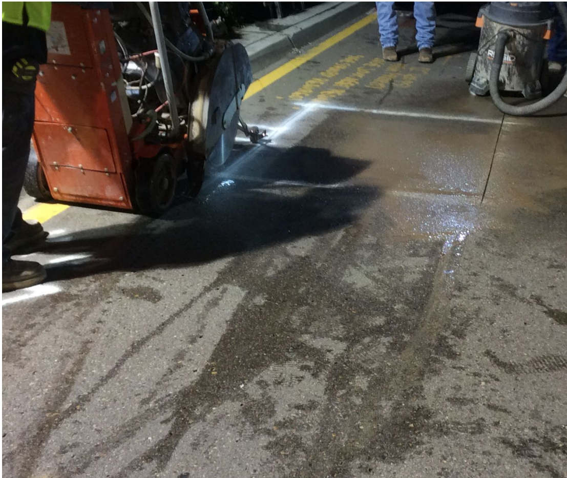
Figure 4: Sawcutting to Access the Abandoned Pipeline for Grout Fill
