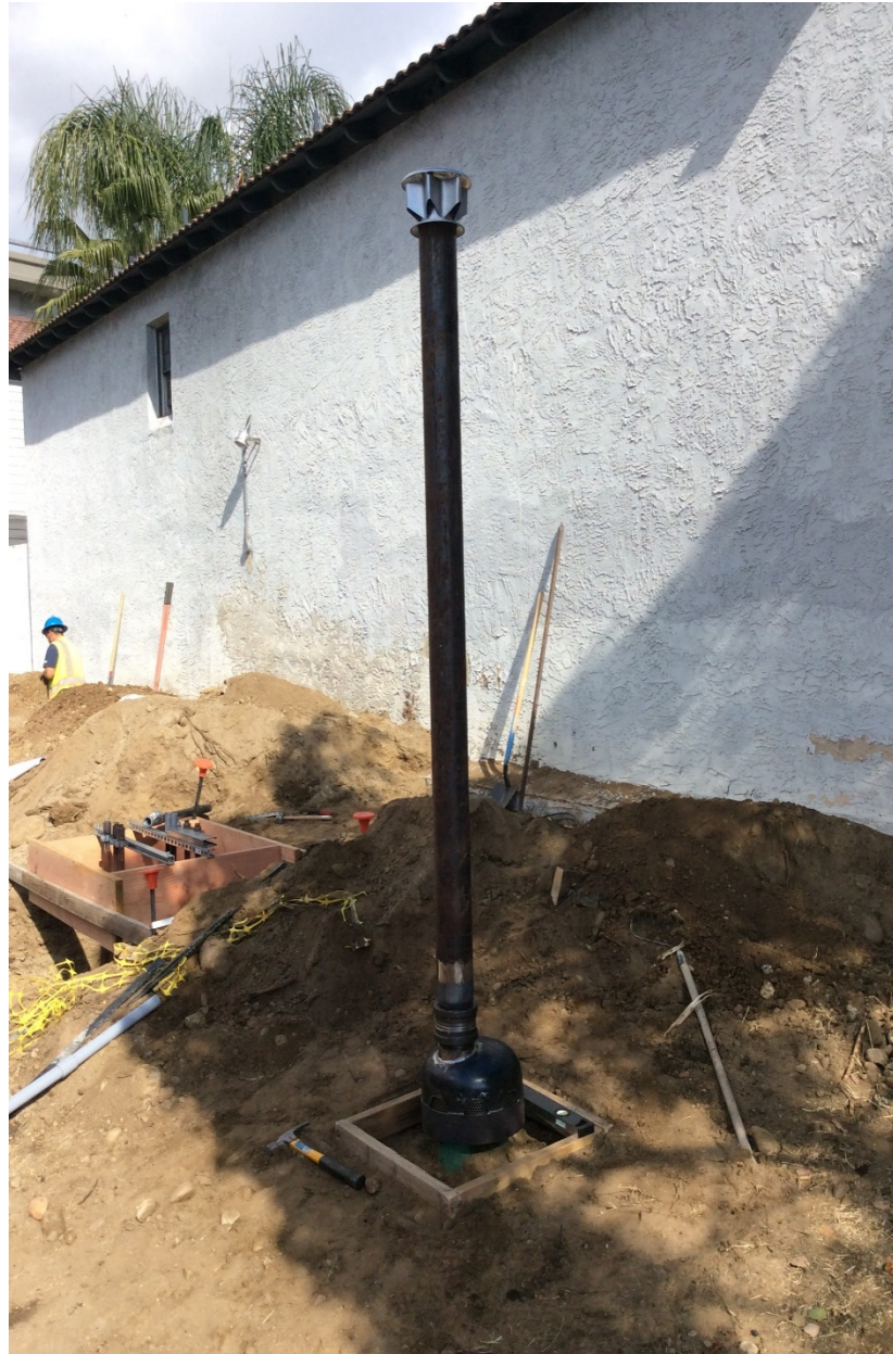
Figure 3: New Vault Vent
