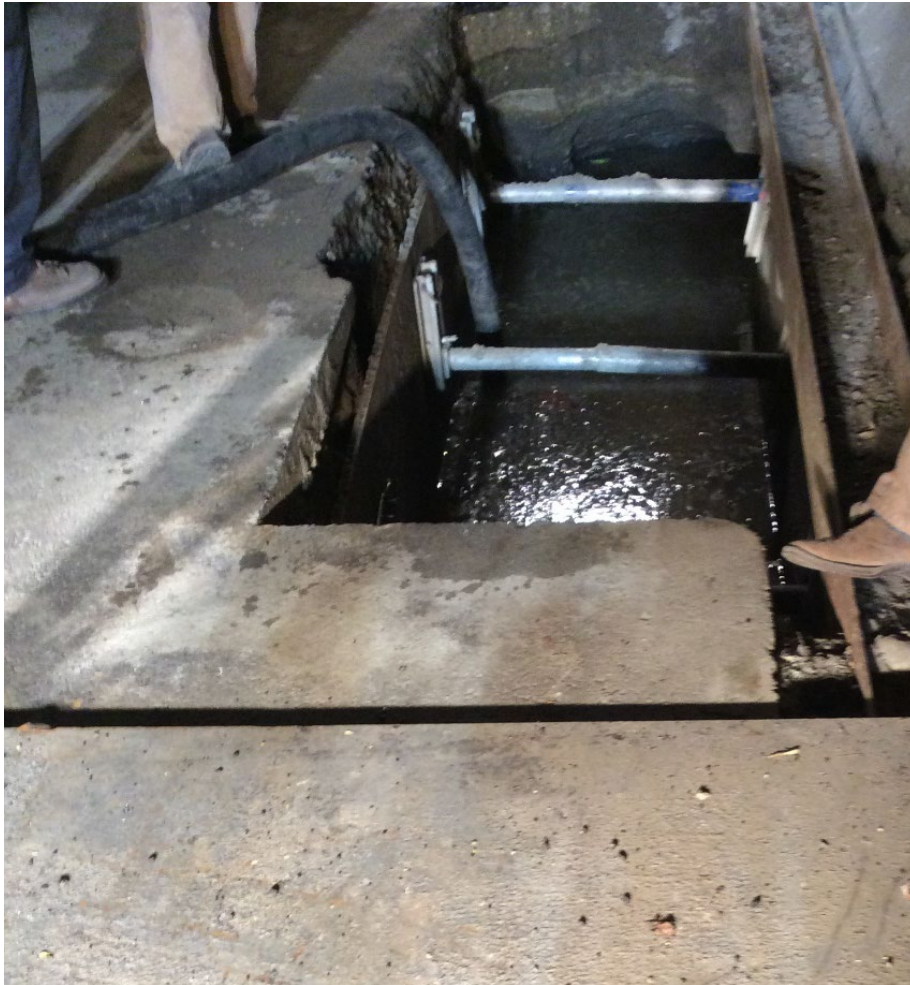
Figure 9: Groundwater Removal from Trench
