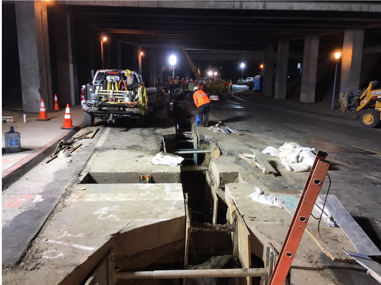
Figure 5: Nighttime Trenching Under the Interstate 8 Freeway
