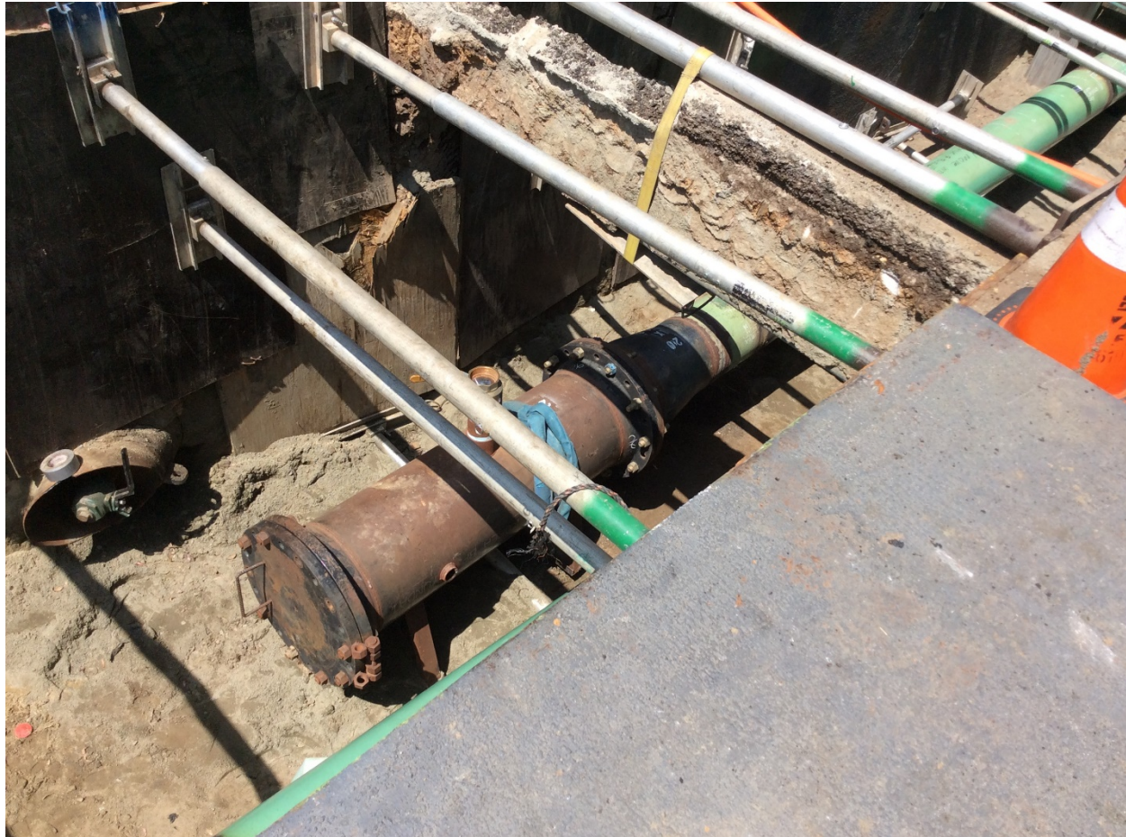
Figure 10: Pig Launcher for Post Completion Hydrotest
