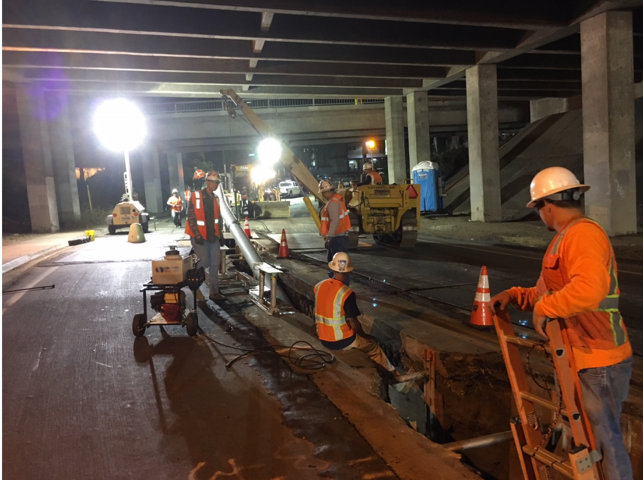
Figure 6: Nighttime Pipelay Under the Interstate 8 Freeway
