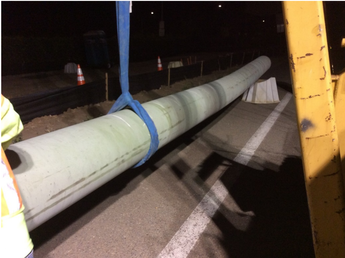
Figure 7: Pipe With Field Bend
