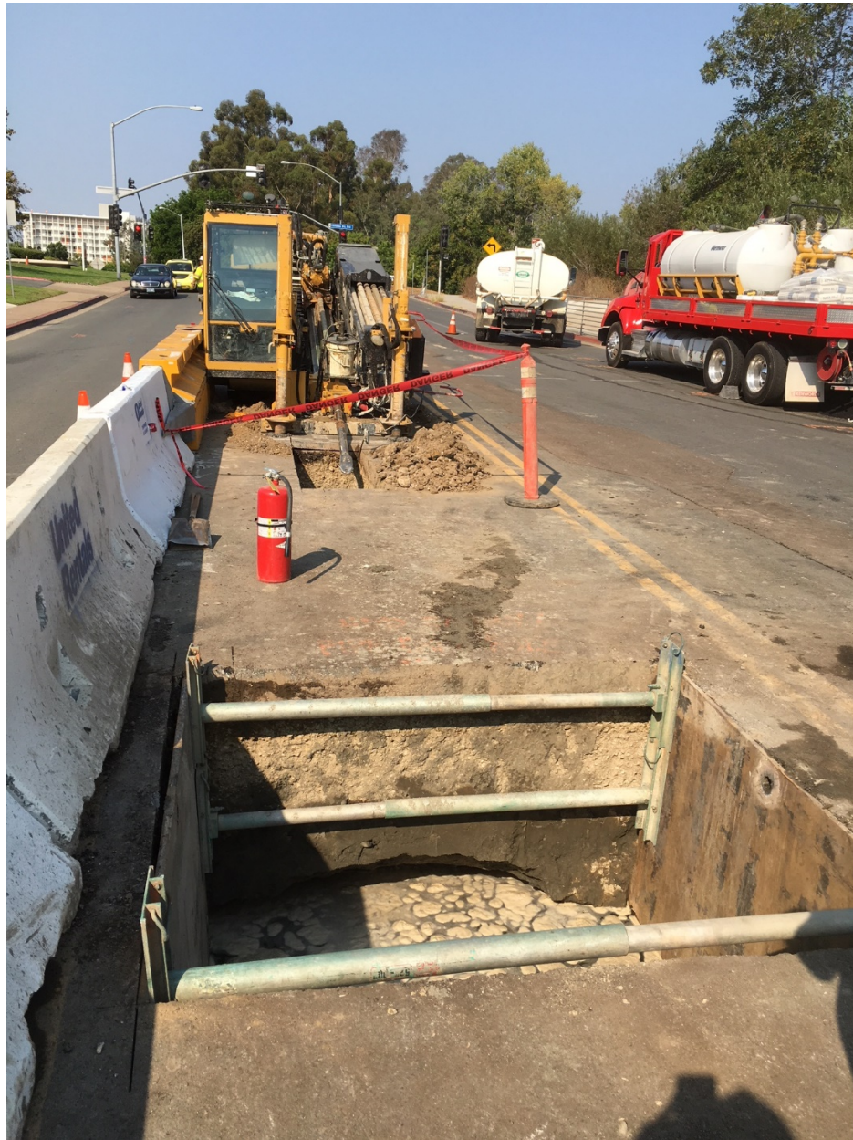
Figure 7: Highway 163 HDD Crossing
