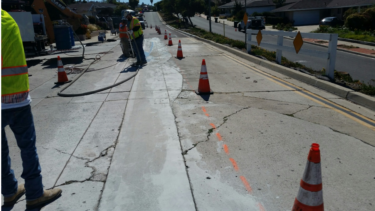
Figure 10: Saw Cutting Operations
