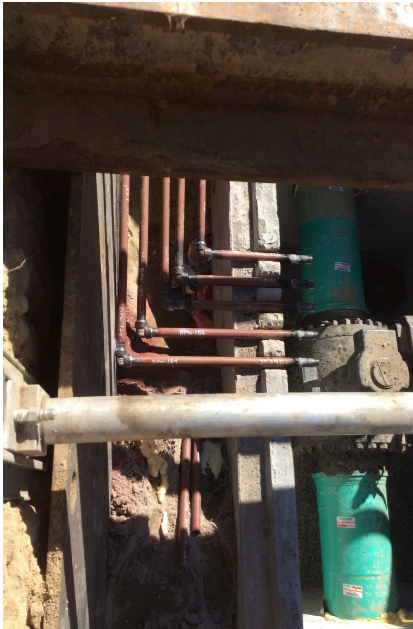
Figure 4: New Sensing Lines
