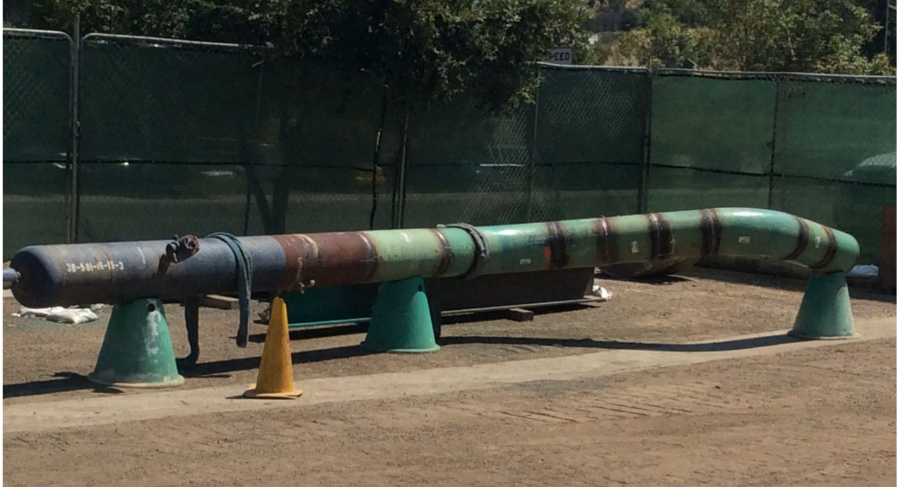
Figure 4: Section 4 Hydrotesting of a Prefabricated Installation
