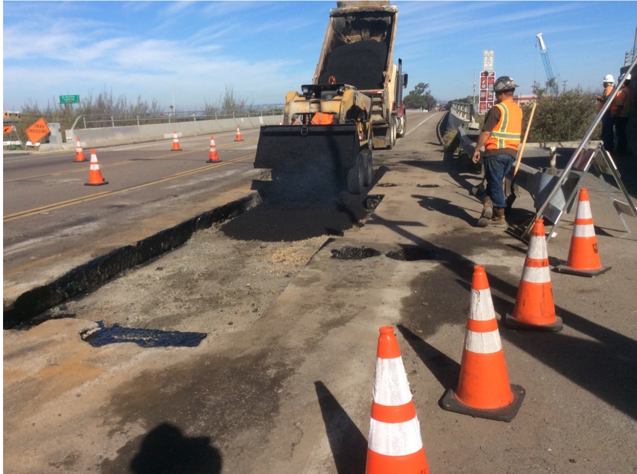
Figure 5: Bell Hole Paving
