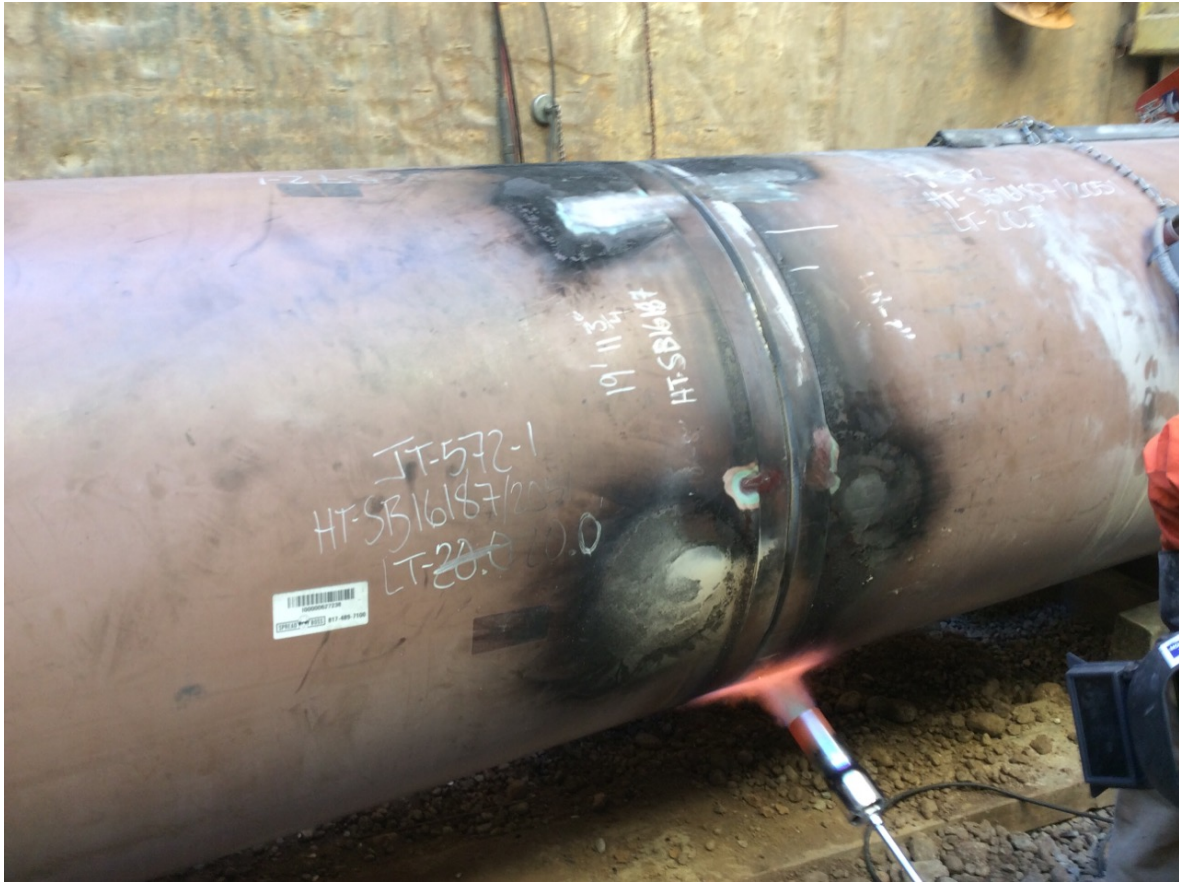
Figure 8: Preheating of Casing Pipe Between Welding Passes
