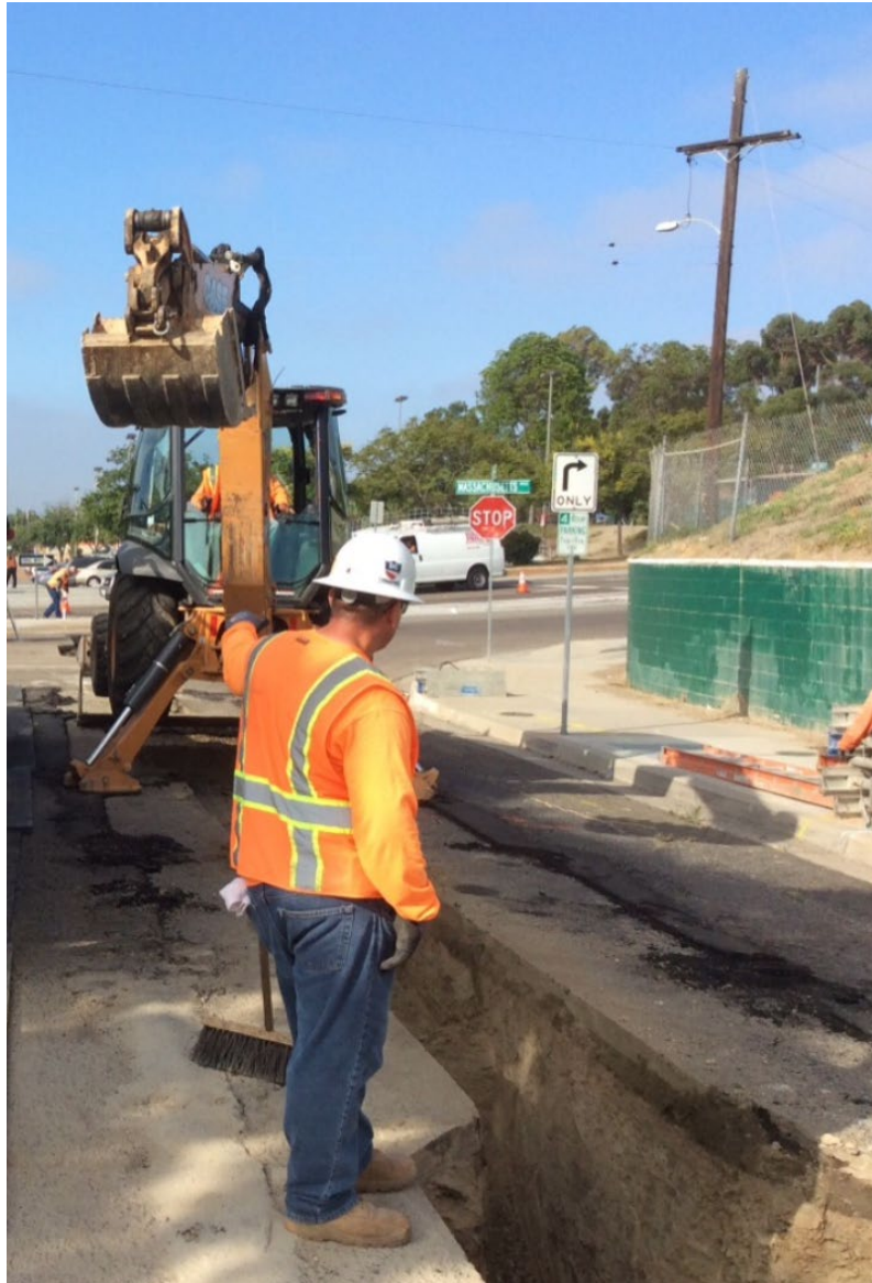
Figure 5: Section 4 Trenching near New MLV Location
