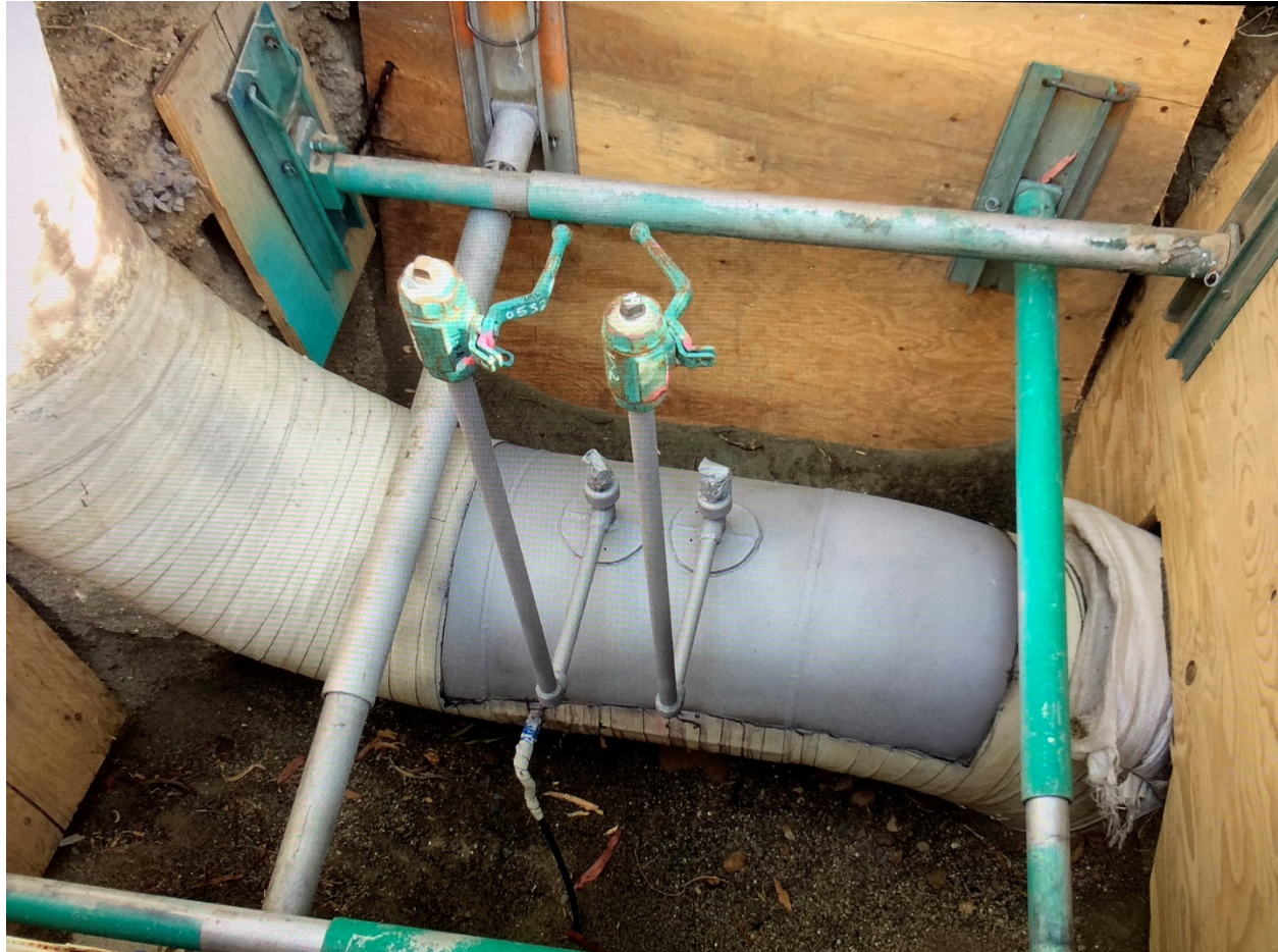
Figure 3: New Instrumentation Taps
