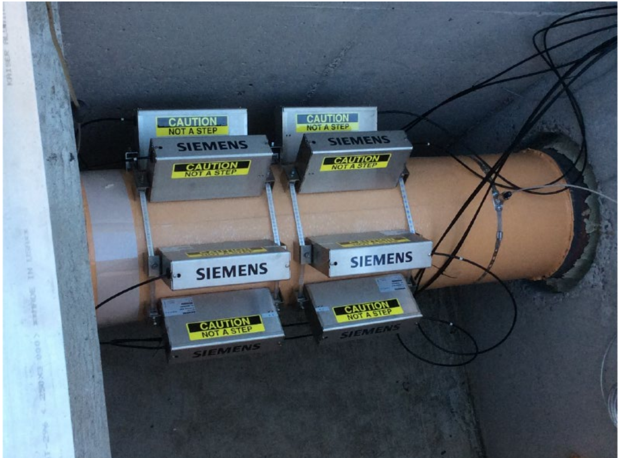
Figure 3: New Clamp On Flowmeter
