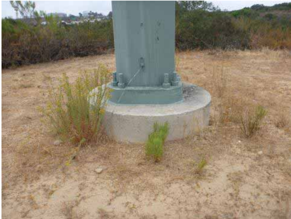
Photo 7. Northeast-facing view of Z479043.
