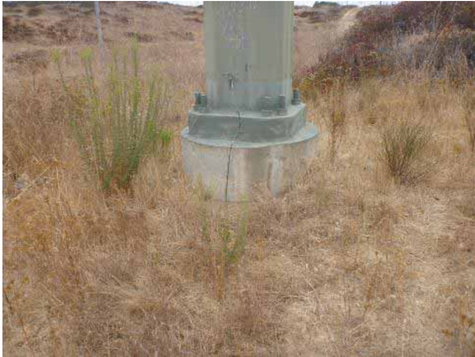
Photo 11. Northwest-facing view of Z479045.
