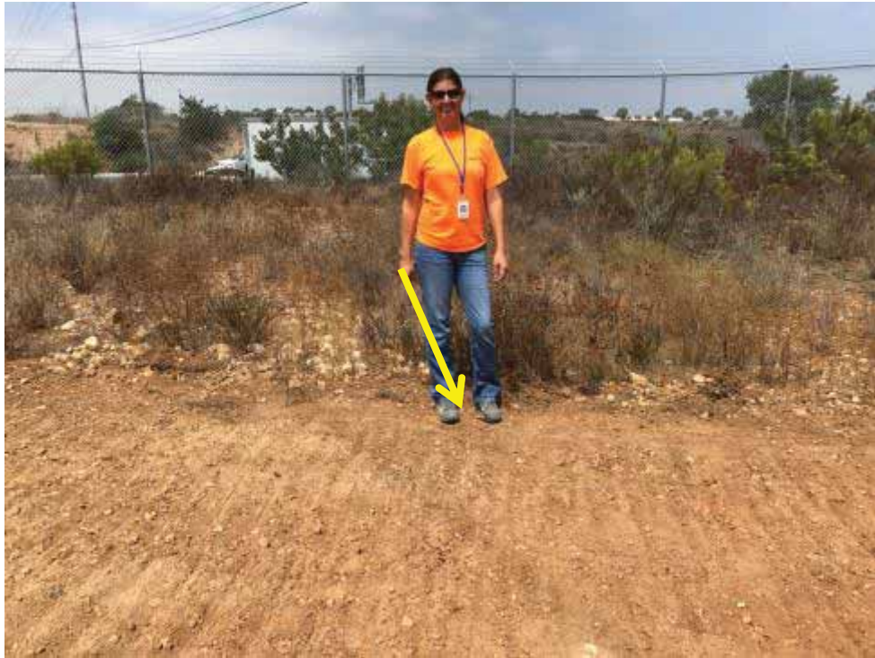
Photo 55. North-facing view of east pole location for GS-28.
