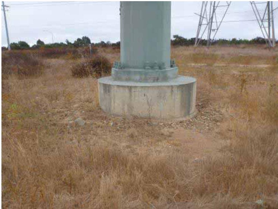
Photo 18. Southwest-facing view of Z479048.
