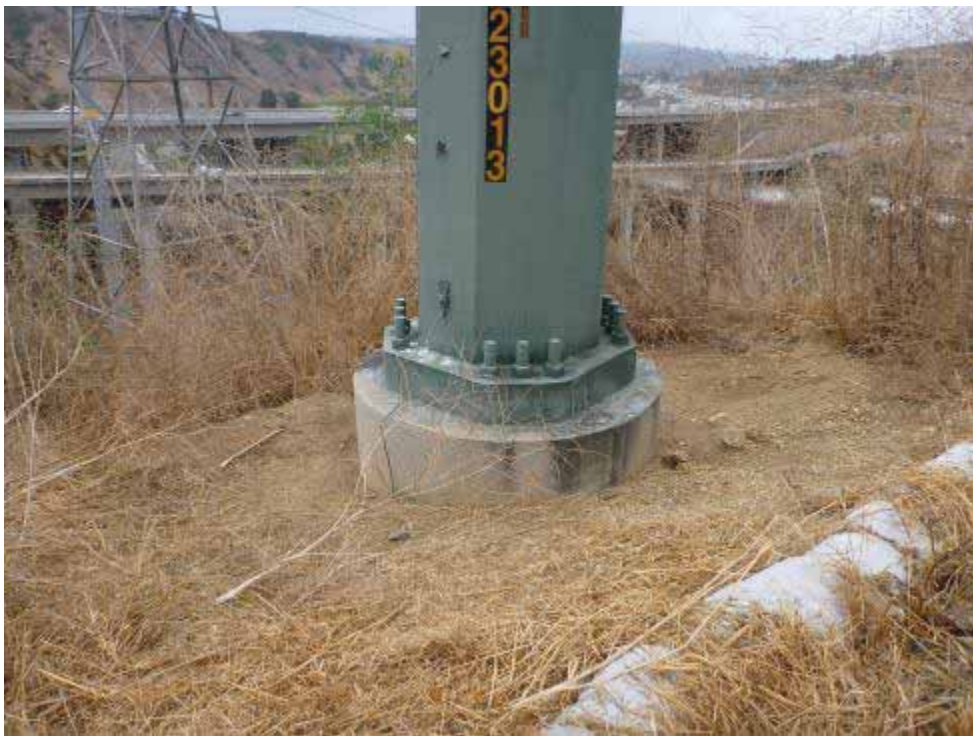
Photo 36. Northwest-facing view of Z479055.
