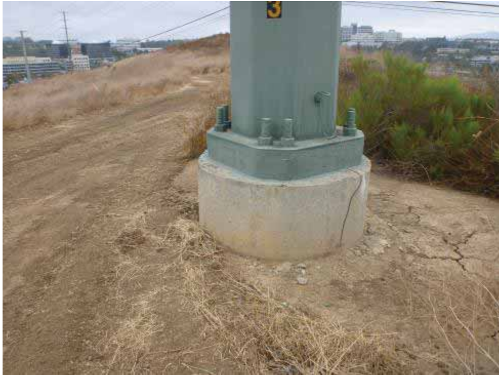
Photo 33. Northeast-facing view of Z479054.
