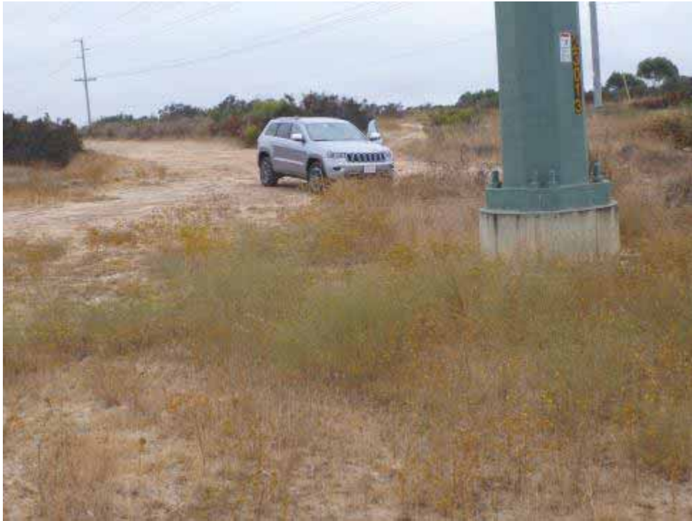
Photo 16. Southwest-facing view of Z479047.
