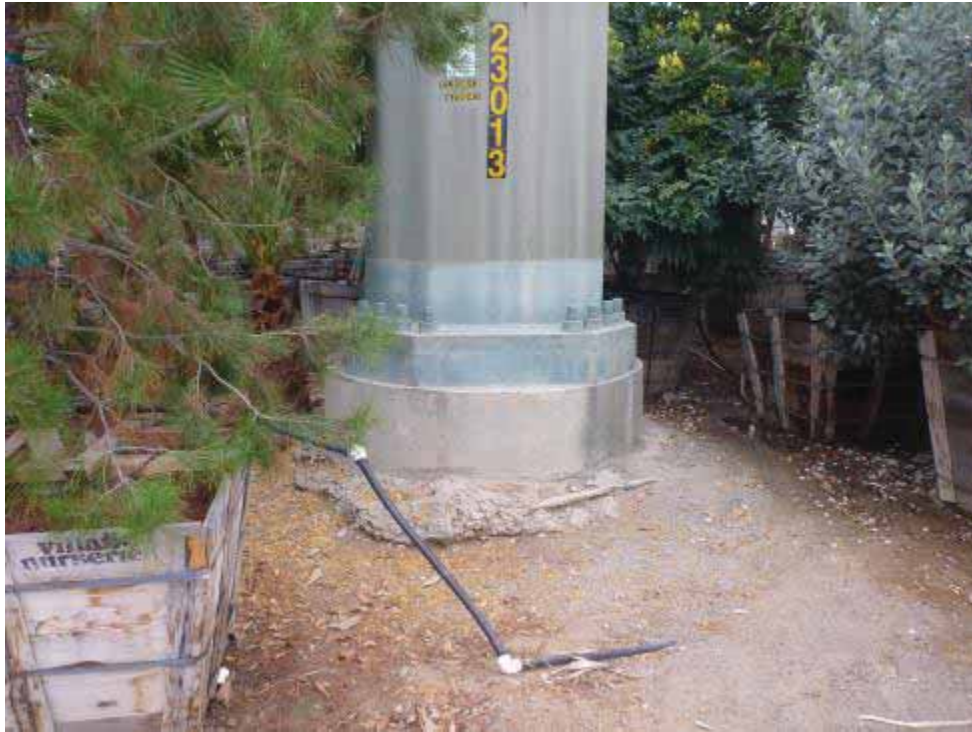
Photo 3. North-facing view of Z479041.
