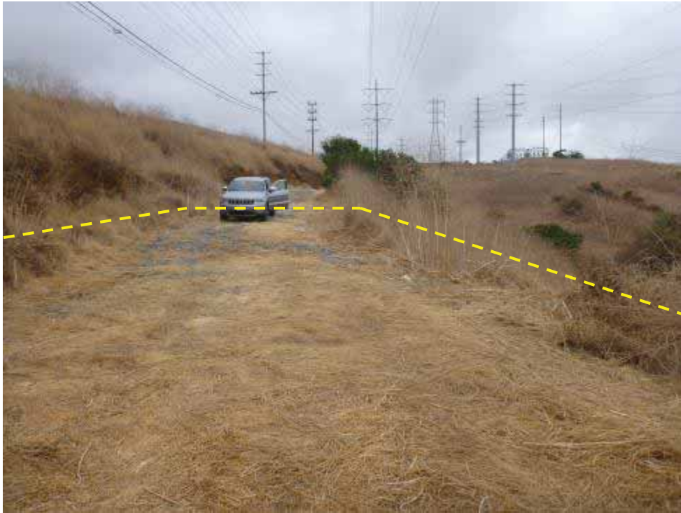
Photo 37. South-facing view of dirt access road off of Eastgate Mall Road to Z479055 and a portion of the work area at Z479055.
