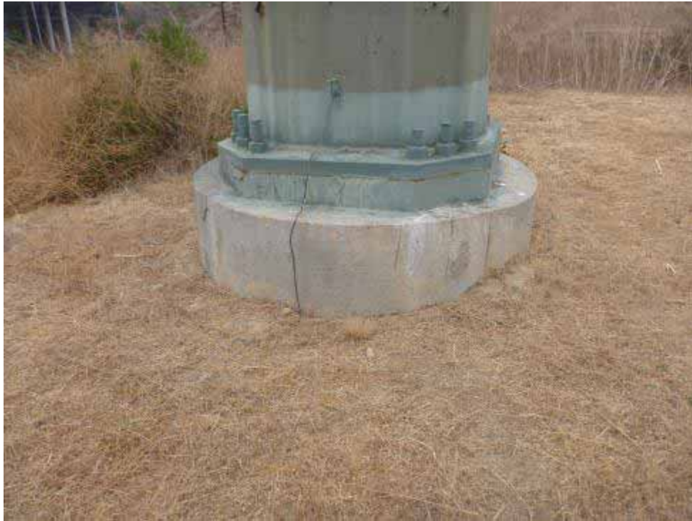
Photo 9. North-facing view of Z479044.
