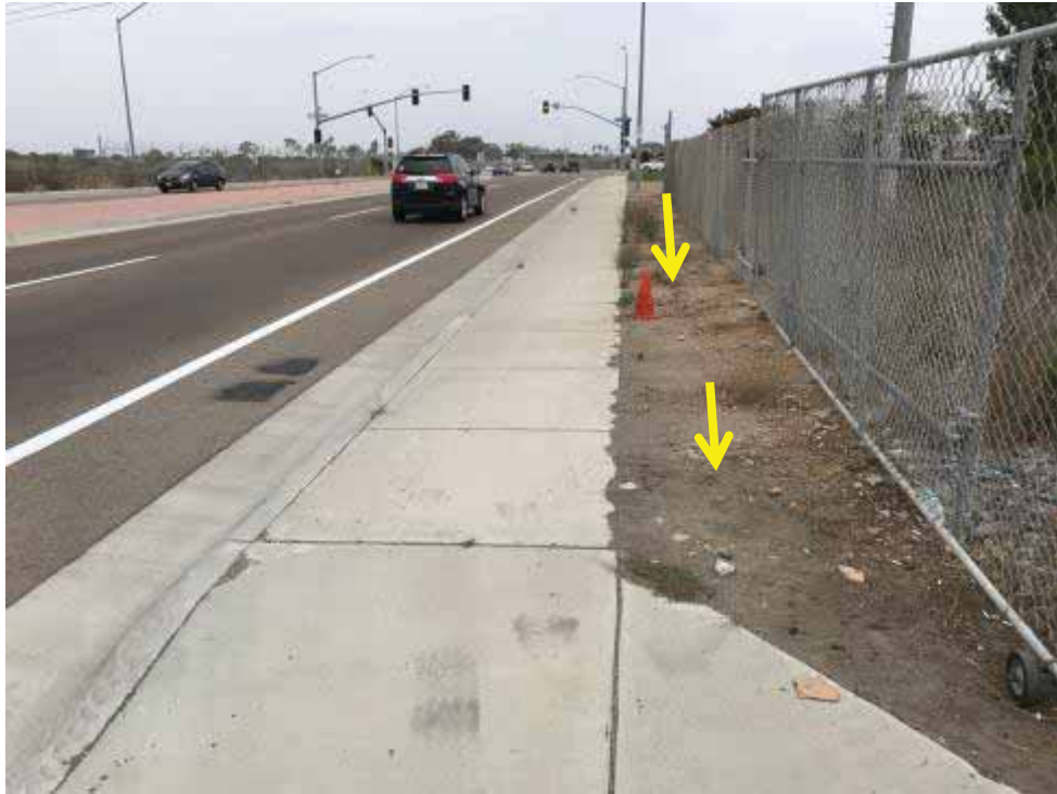
Photo 51. East-facing view of GS-26 (yellow arrows indicate pole locations).
