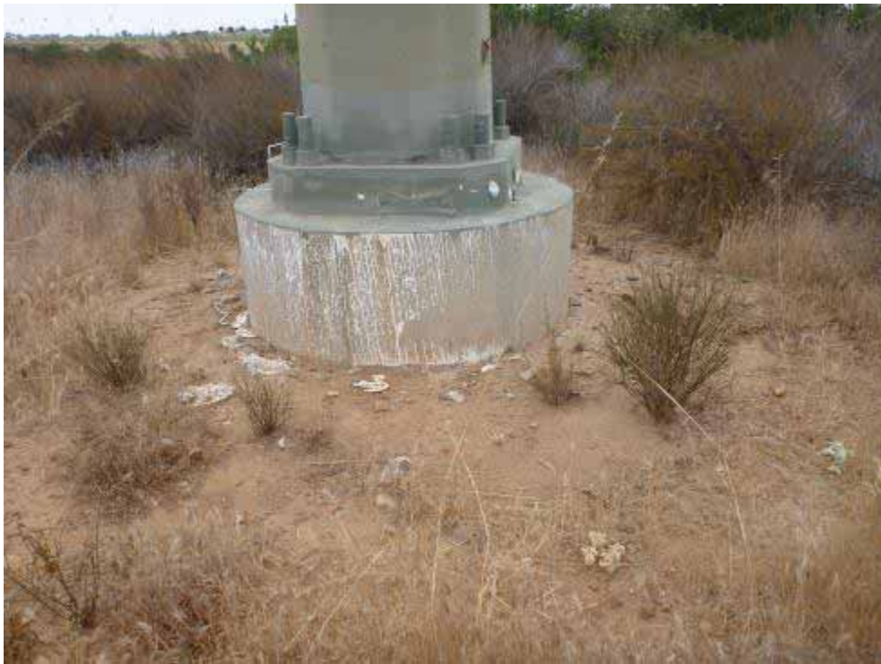
Photo 14. East-facing view of Z479046.
