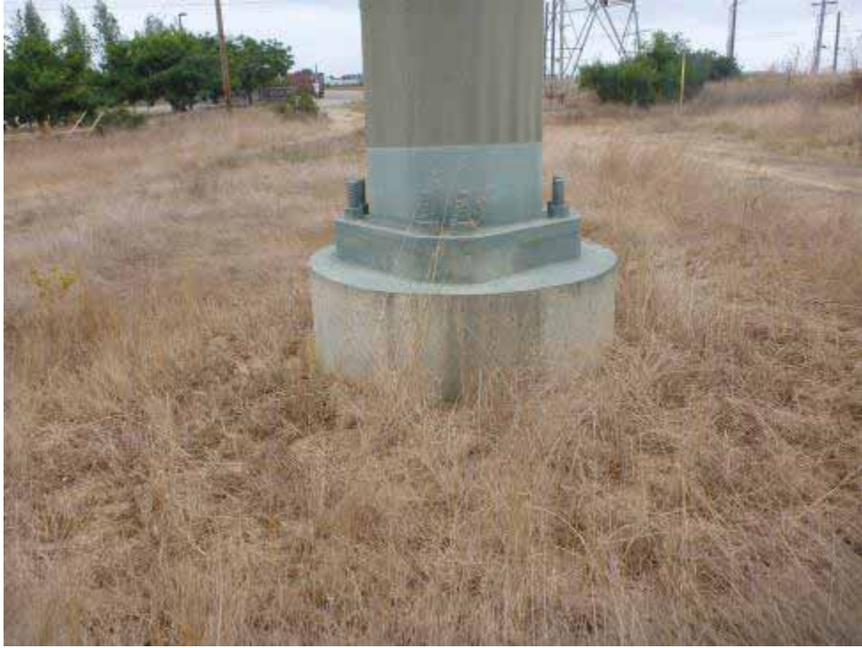
Photo 29. Northwest-facing view of Z479052.
