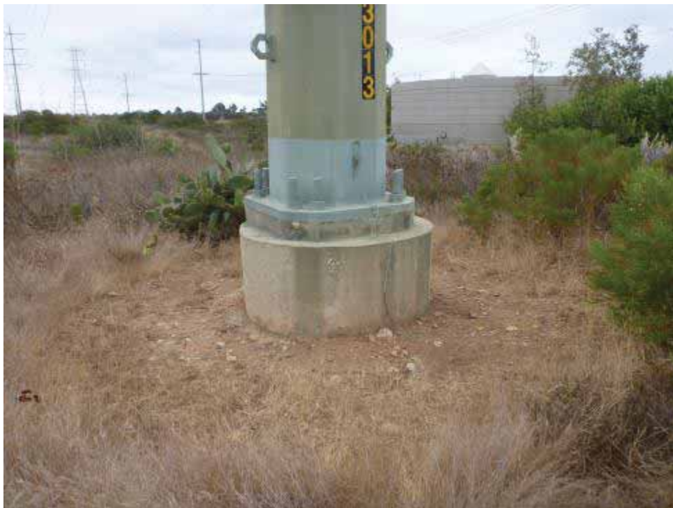
Photo 24. Southwest-facing view of Z479050.
