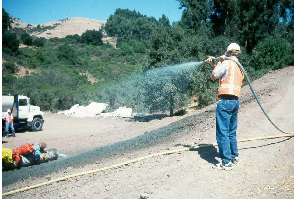
Applying hydroseed.
