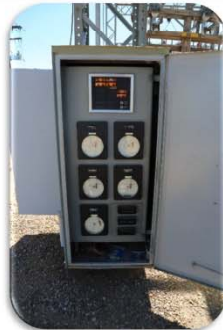
Analog Relay Equipment
