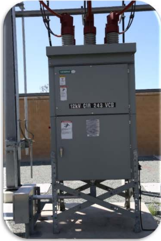
Vacuum Circuit Breakers
