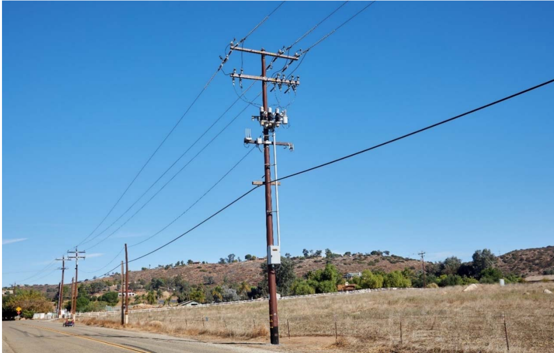
Figure 2 Completed Covered Conductor Project
