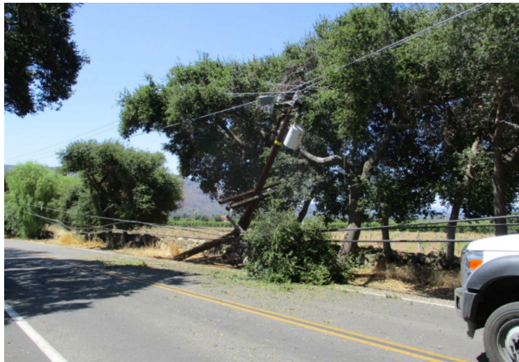
Figure 9: Covered Conductor Contact with Vegetation After Car-Hit-Pole Ojai, California – July 24, 2020
