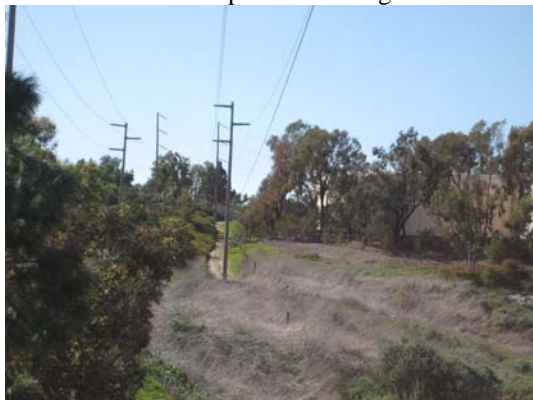
Example: 138 kV poles located on the edge of very flammable canyon.
