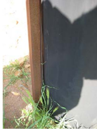
Example: The ground wire cover does not completely cover the copper wire creating a fire hazard. These poles will require brushing.
