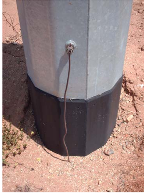
Example: Above grade ground wires without the cover. These poles require brushing.
