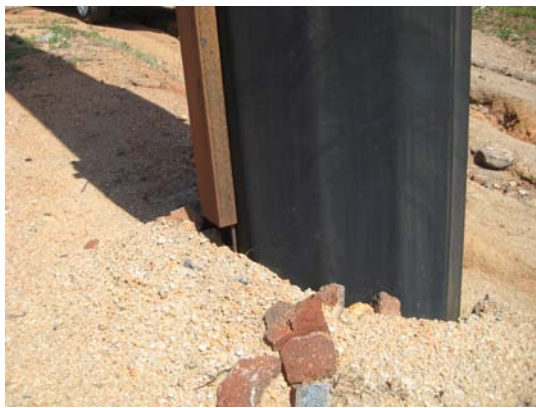
Example: The ground wire cover does not completely cover the copper wire creating a fire hazard. These poles will require brushing.
