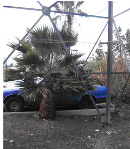
Example: The palm requires removal. It provides access to the climbing guard
