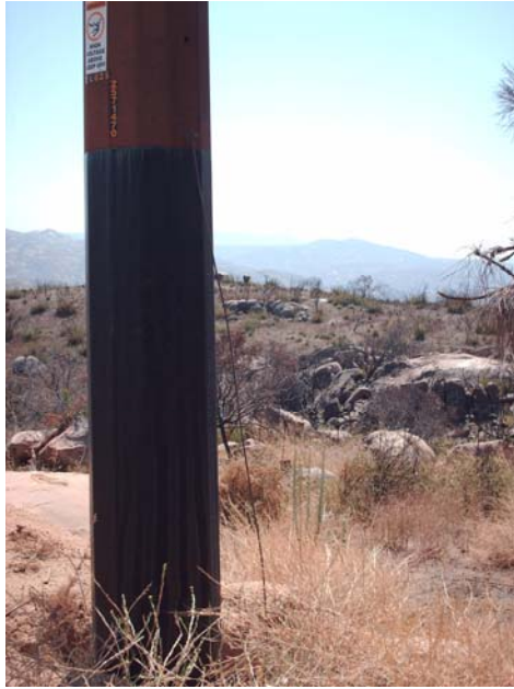
Example: Above grade ground wires without the cover. These poles require brushing.
