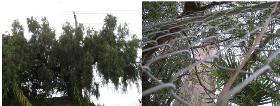
Example: Pole requiring climbing space. It is located in a backyard butting up to a canyon. There is no bucket truck access and the pepper tree in growing too close to the pole.
