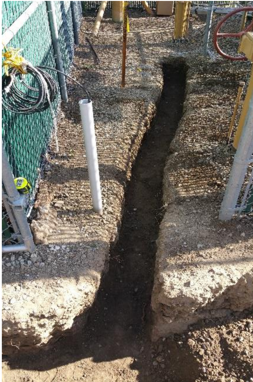
Figure 7: Conduit Trenching at Sexton Canyon
