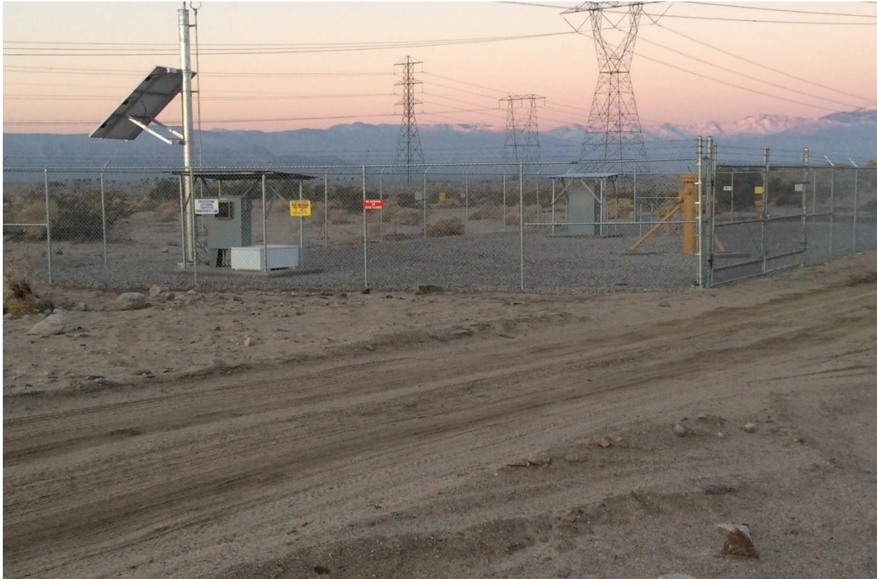
Figure 6: Fargo Canyon – Project Site Post Construction
