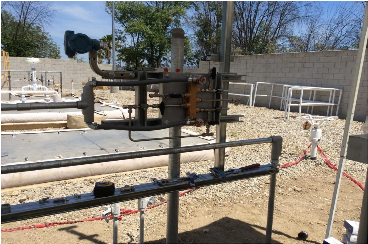
Figure 9: RCV at Westside Station
