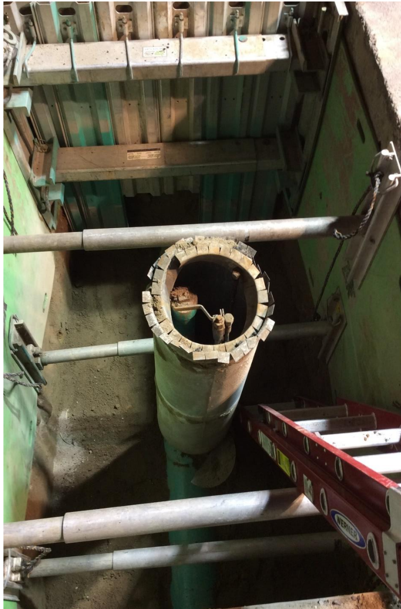
Figure 3: Valve Extension
