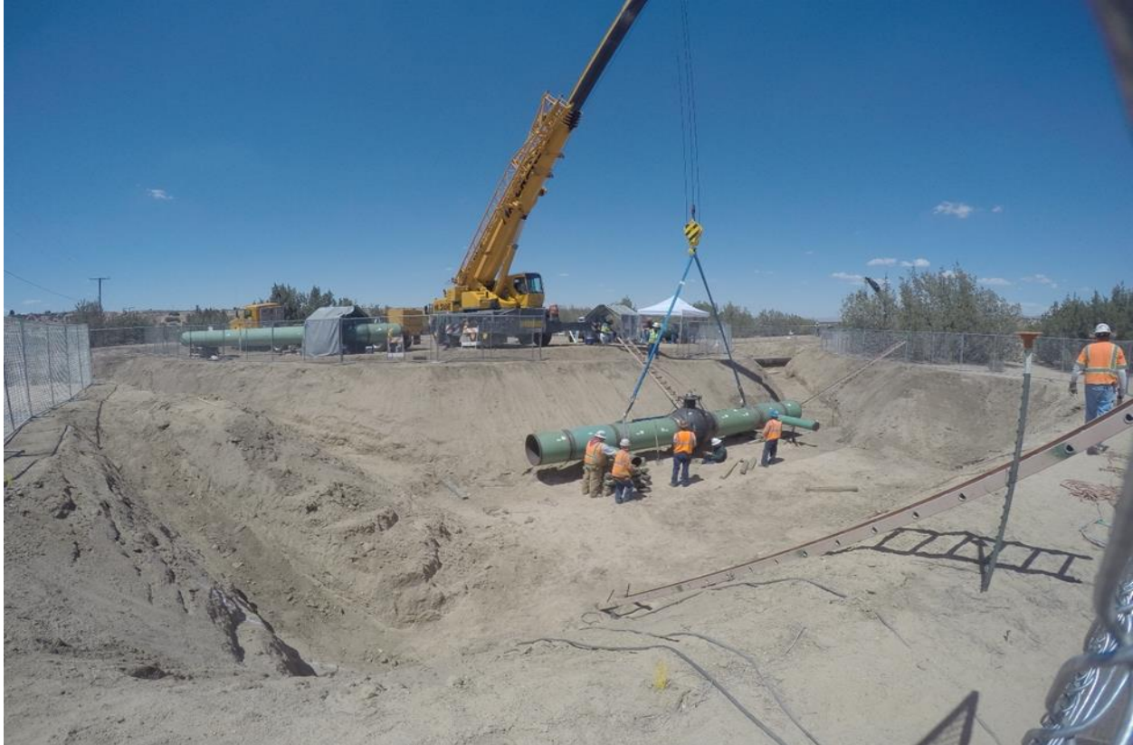
Figure 3: Placement of the New Mainline Valve Assembly
