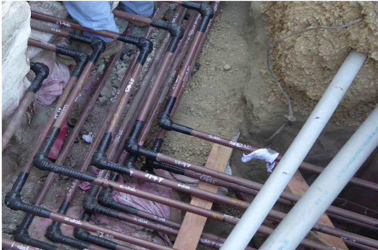
Figure 9: Typical Sense Line Piping
