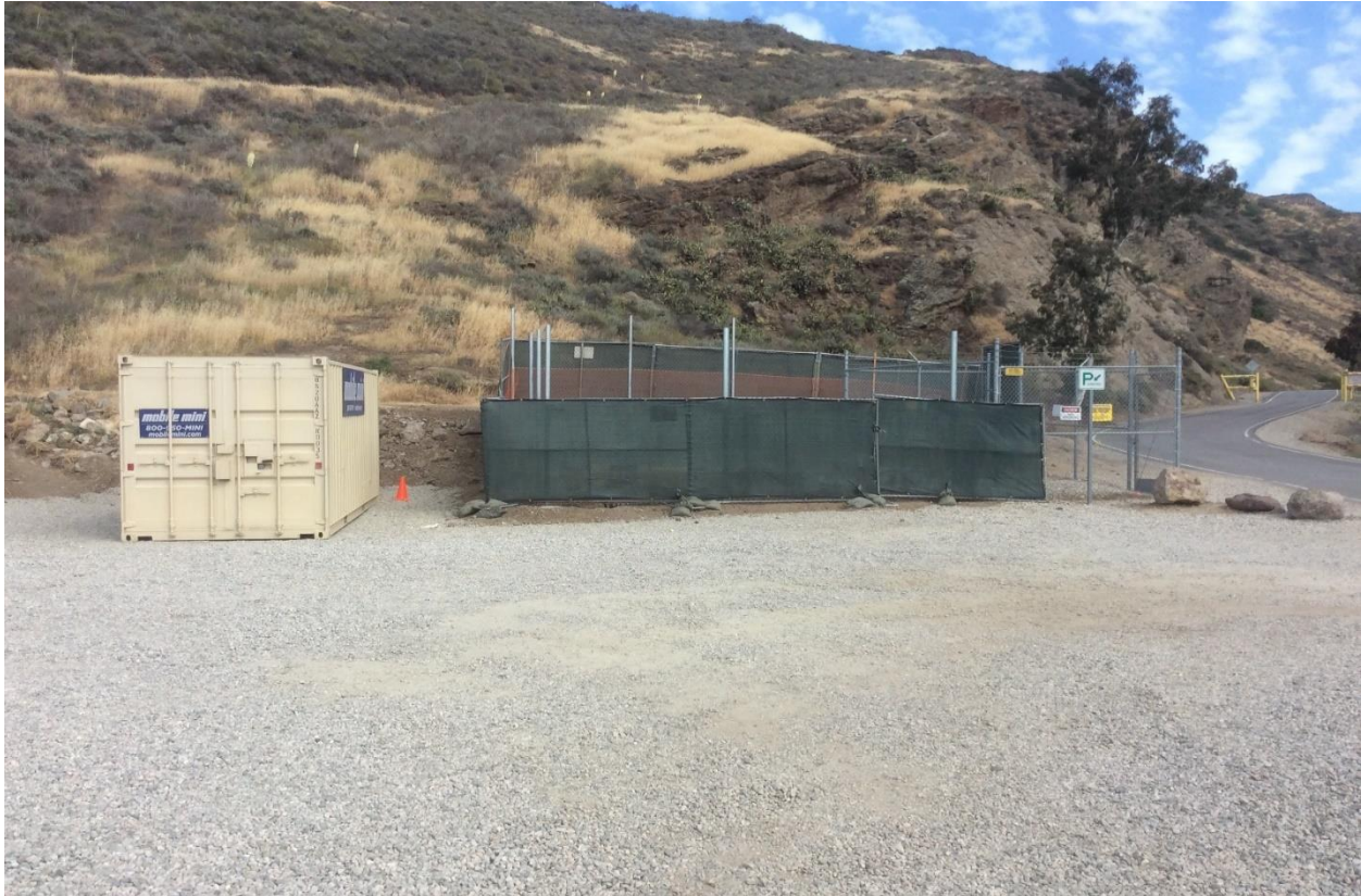
Figure 8: Equipment at Hill Canyon
