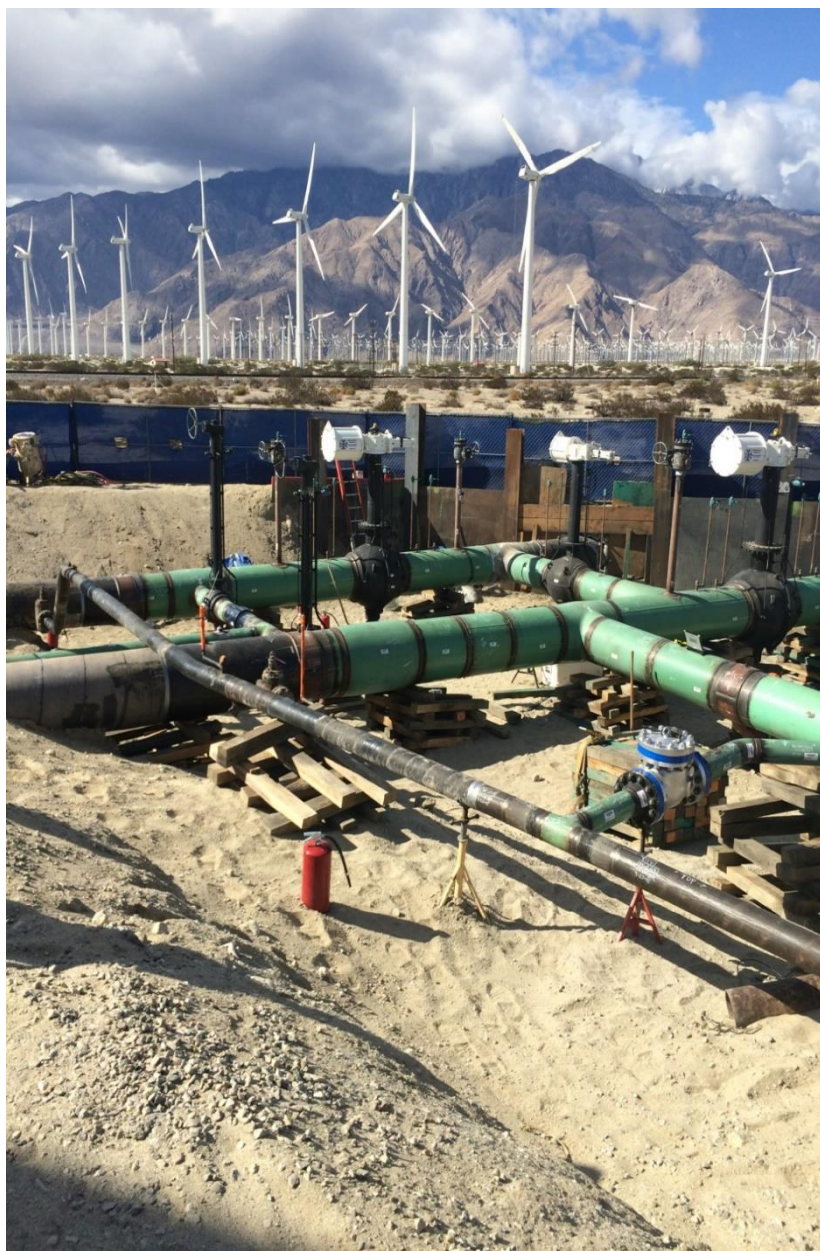
Figure 5: Garnet Station – New Piping Assembly After Installation
