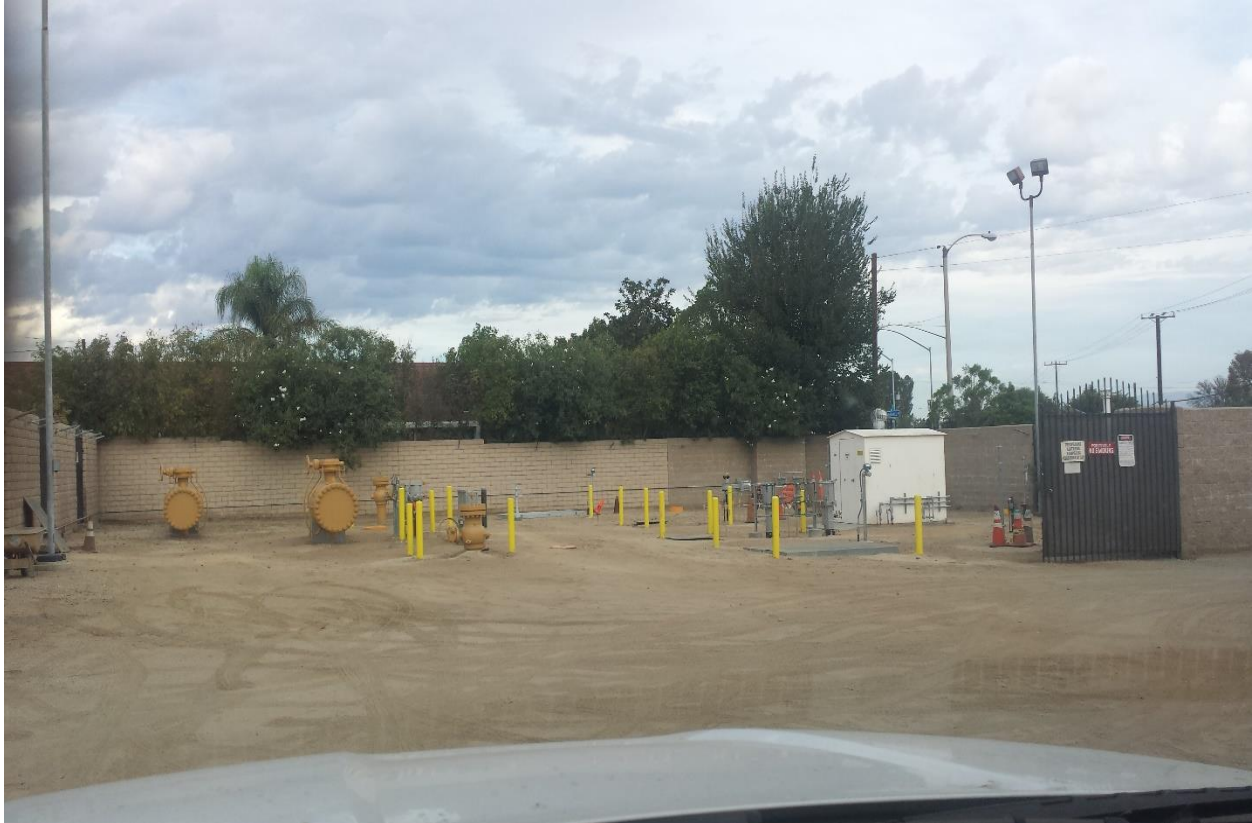
Figure 7 – Newhall Station – Newhall Station Post Construction
