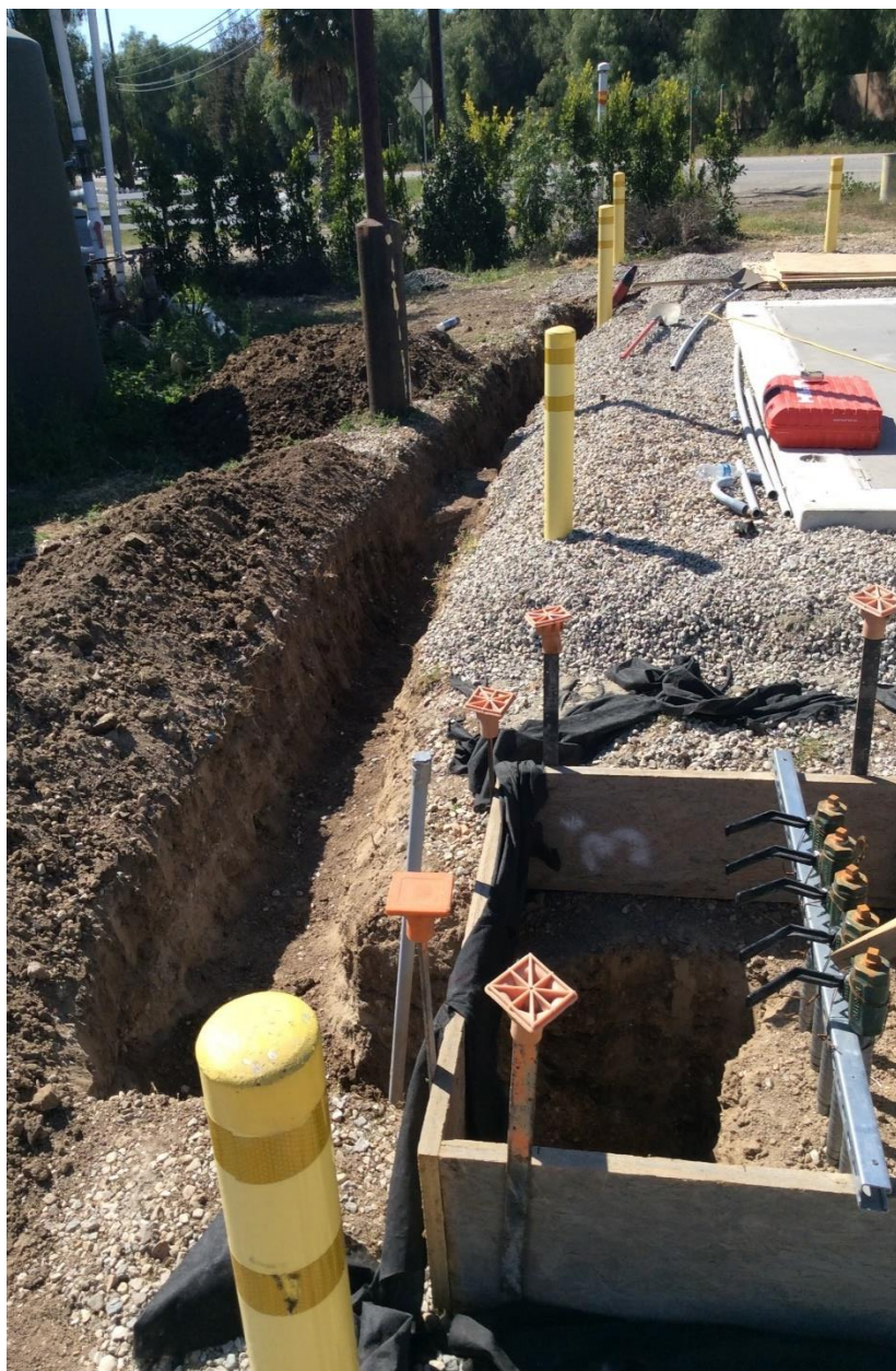
Figure 8: Trenching at Santa Rosa Road
