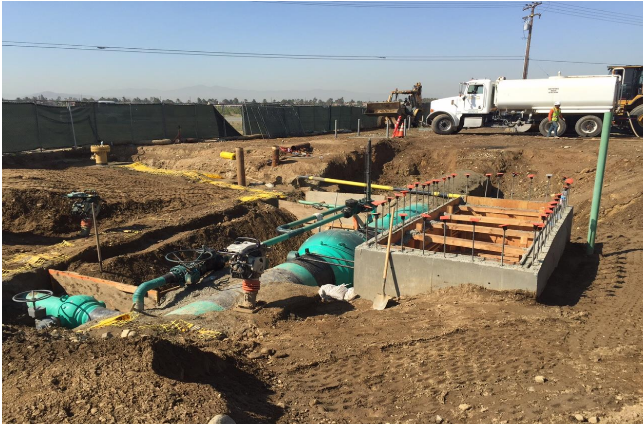
Figure 3: New Mainline Valve and Bottom Section of the New Vault
