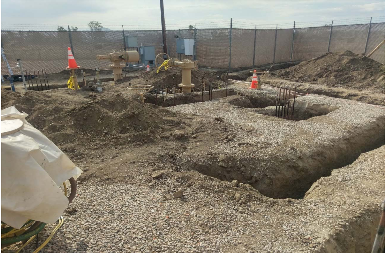
Figure 7: Rainbow Valve Enhancement Project Bundle, Briggs & Marino Site – Conduit Trench Excavation
