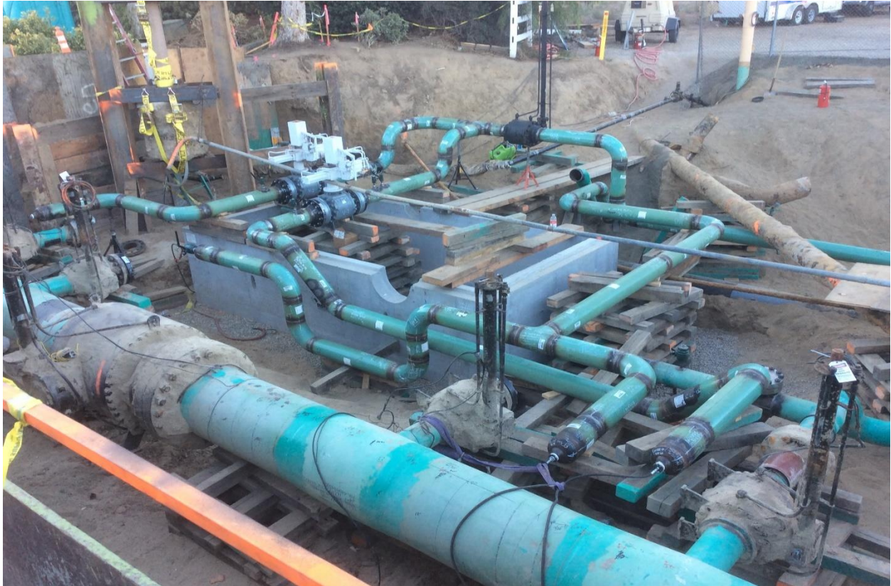
Figure 6: Castaic Junction – New Piping Assembly Prior to Tie-in
