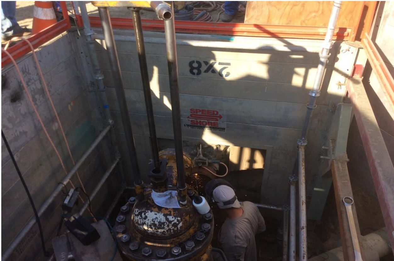
Figure 7: Welding Plate on Abandoned [REDACTED] Line
