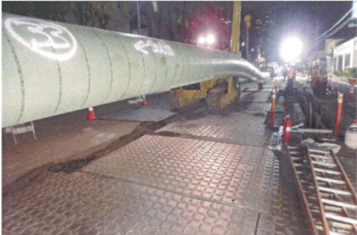
Figure 7: Preparing Pipe String for Installation in Trench
