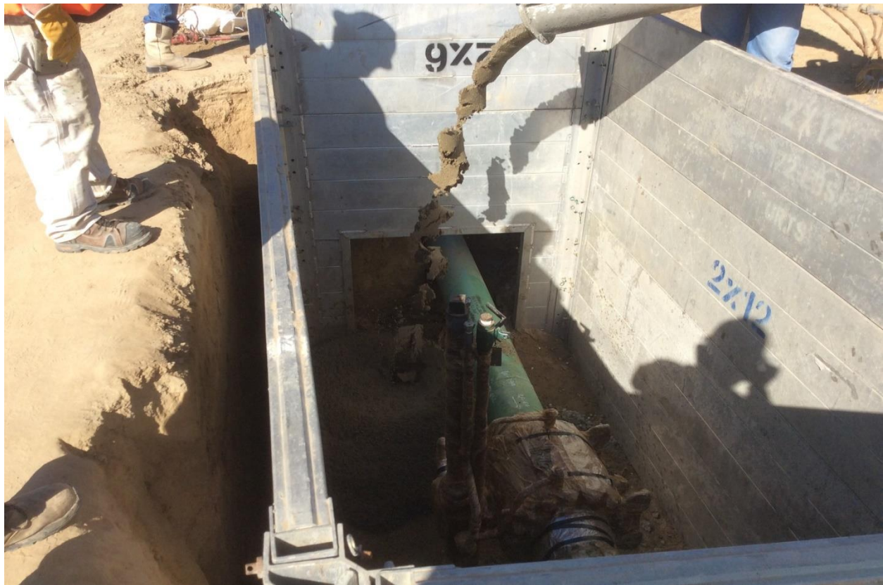
Figure 10: Slurry Backfill
