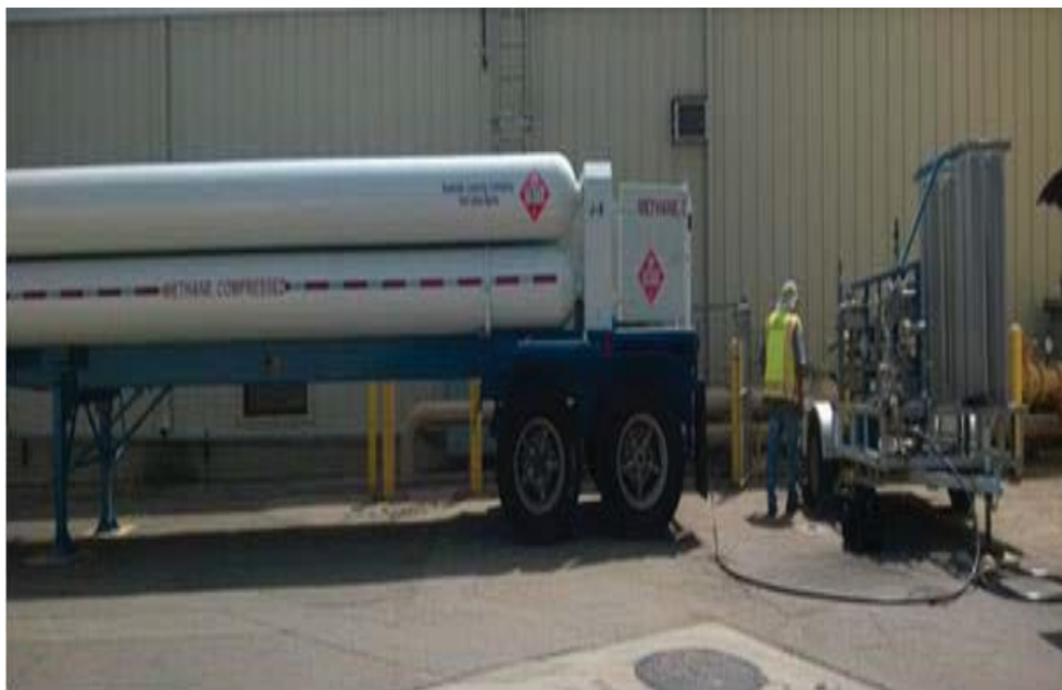
Figure 16: CNG for Temporary Bypass
