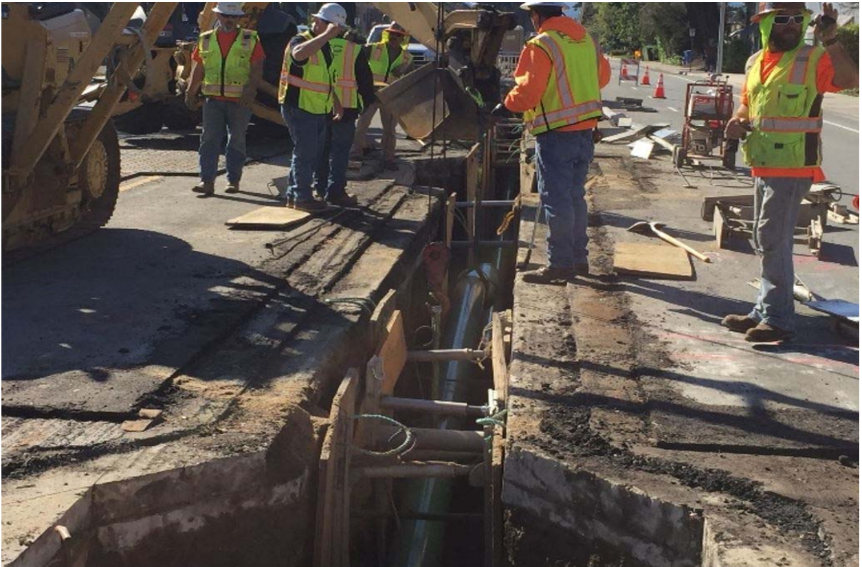
Figure 4: Installation of Pipe along South Higuera Street
