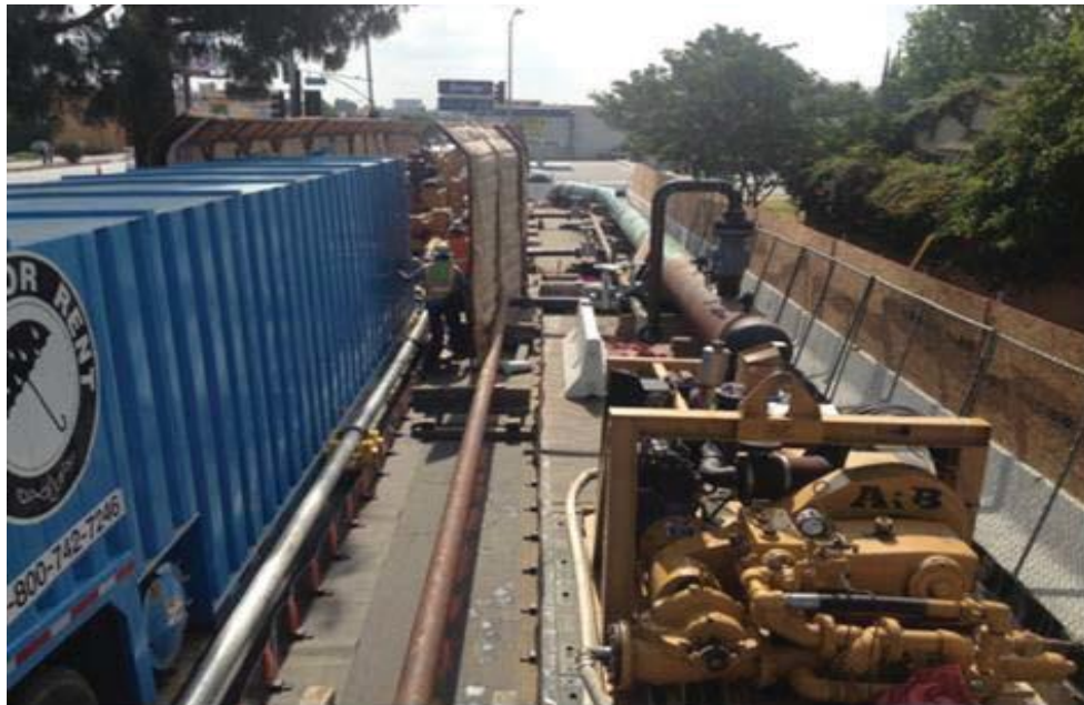
Figure 12: Hydrotest Set Up with Sound Proofing to Minimize Noise Complaints (located behind Baker tank)
