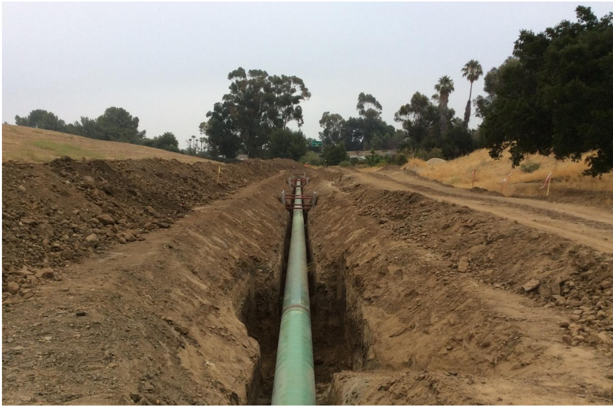
Figure 5: Open Trench Installation of Replacement Pipeline
