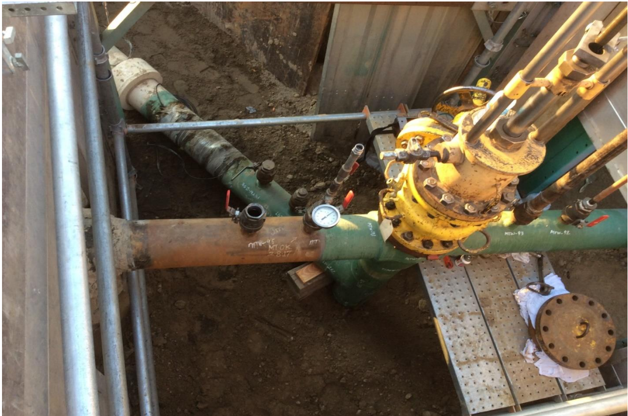
Figure 8: [REDACTED] Line Prior to Cut and Cap
