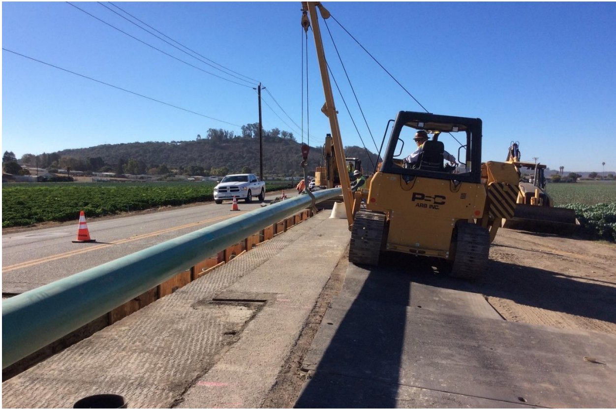
Figure 11: Section 7A - Side Booms to Move Welded Pipe into the Trench
