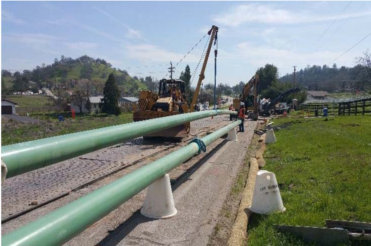
Figure 6: Laying Double Joints in Narrow Right-of-Way
