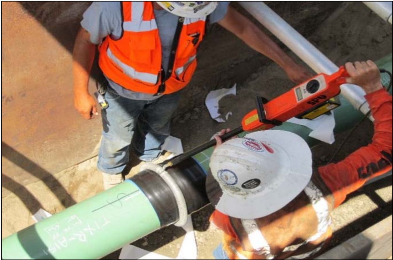
Figure 8: Section 2 – Checking Integrity of Coating
