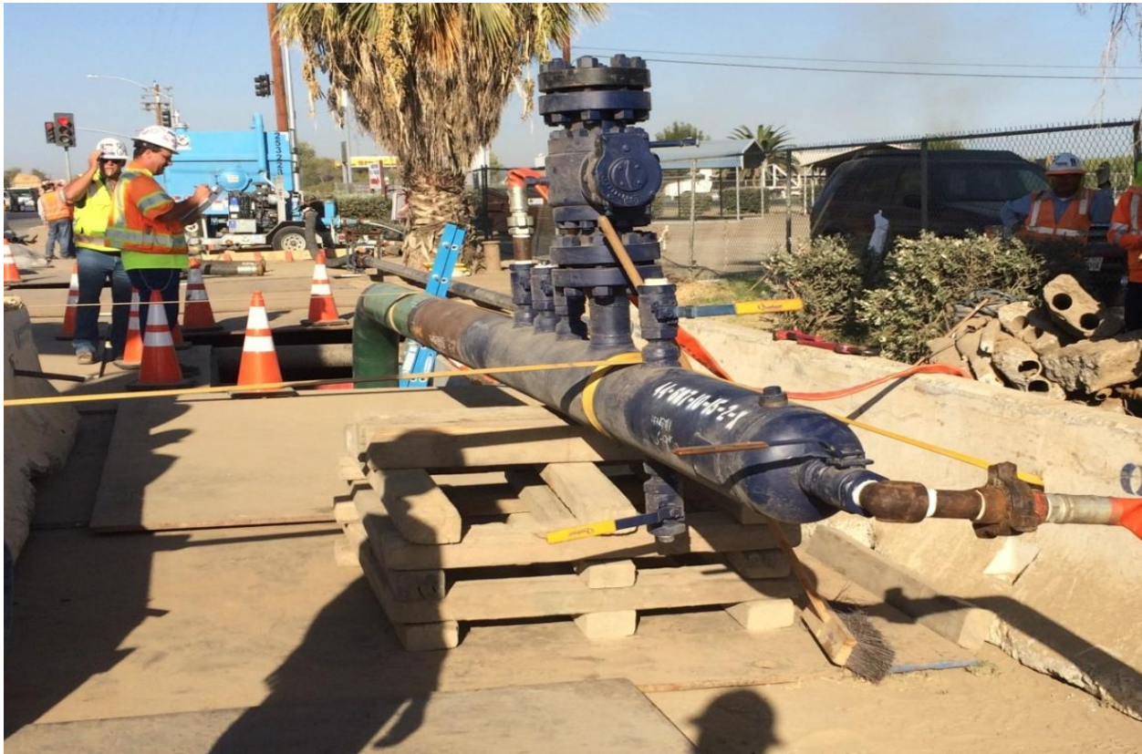
Figure 4: Test Head Assembly During Hydrotest Operations
