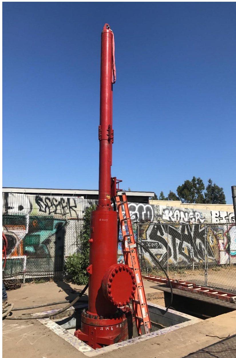
Figure 6: Pressure Control Fitting Isolation Machine
