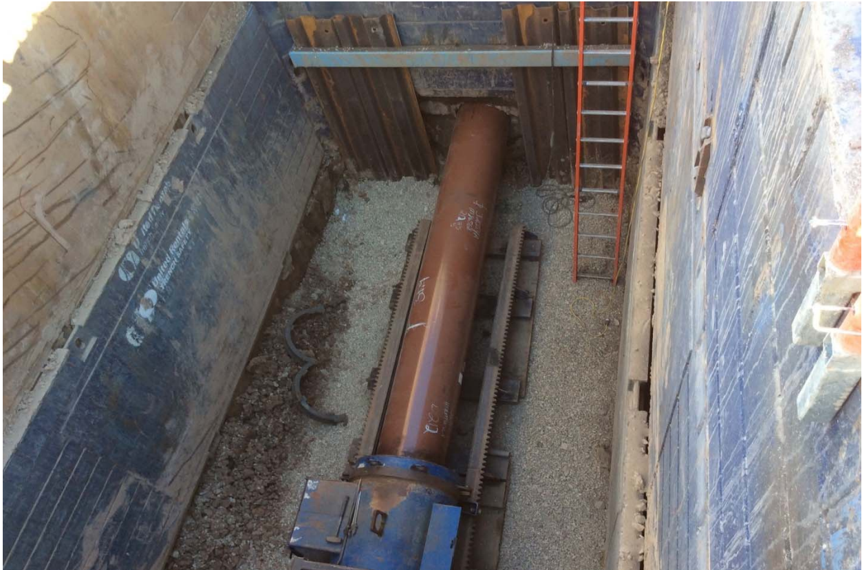
Figure 6: Boring Machine Pushing [REDACTED] Abrasive Resistance Overcoat Pipe
