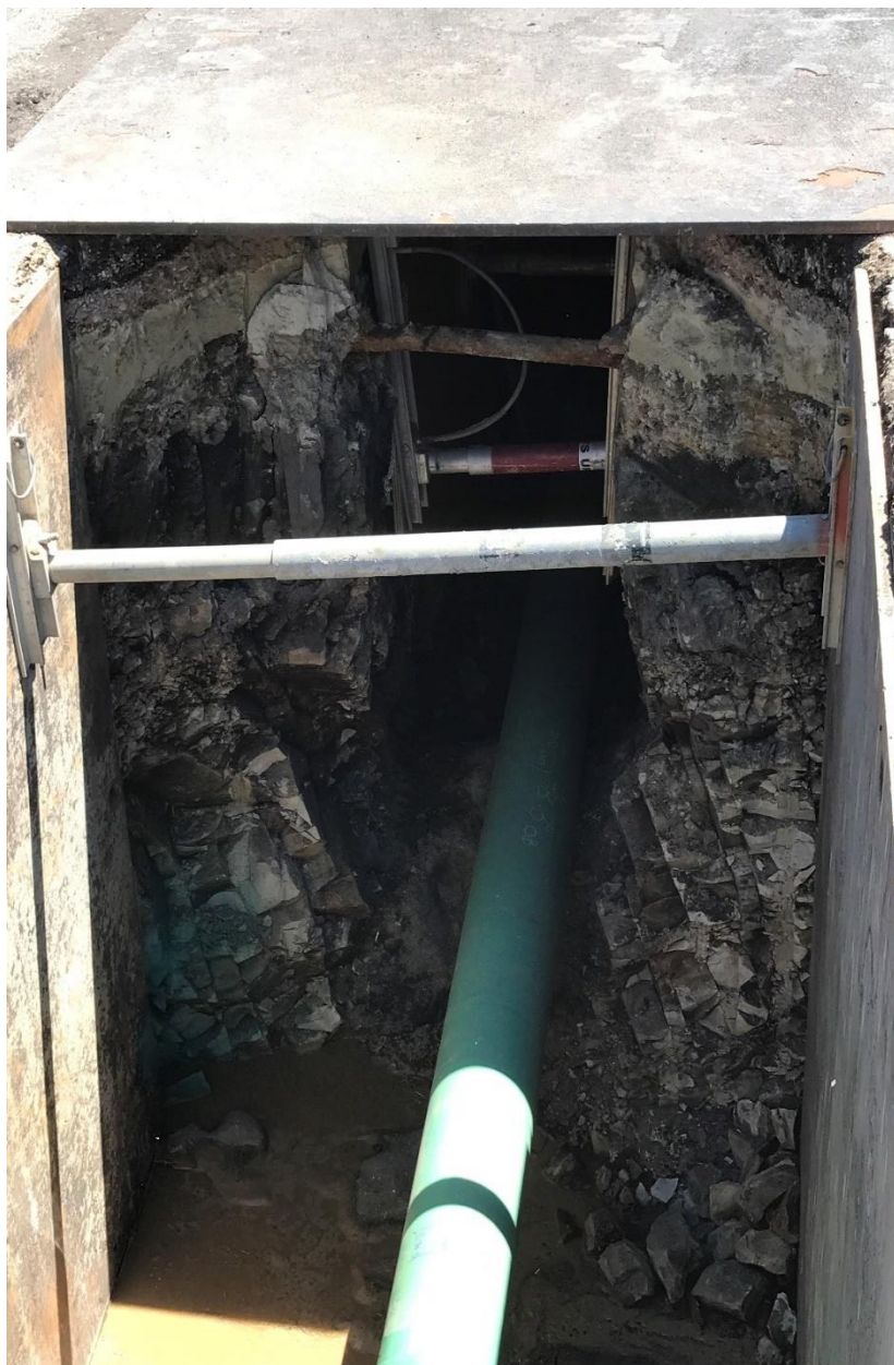
Figure 8: New Pipe Installation in Rocky Conditions
