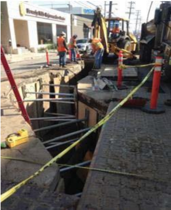
Figure2: Lowering Pipe in Congested City Area
