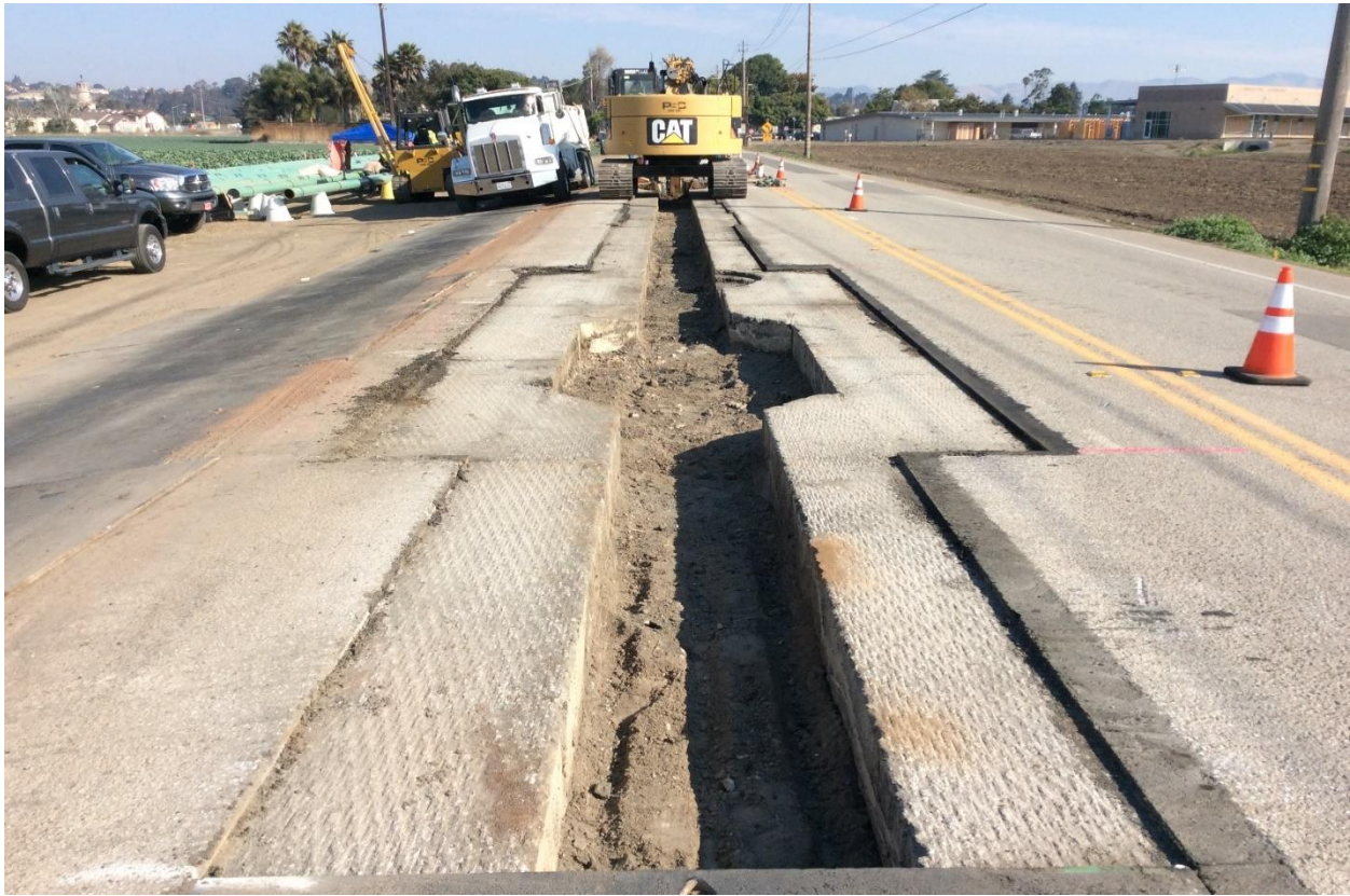
Figure 10: Section 7A - Stripping and Excavating a Trench Near the Valve Assembly
