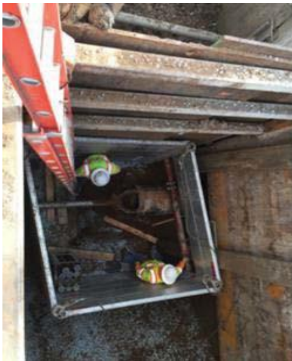
Figure 8: Jack and Bore Operation
