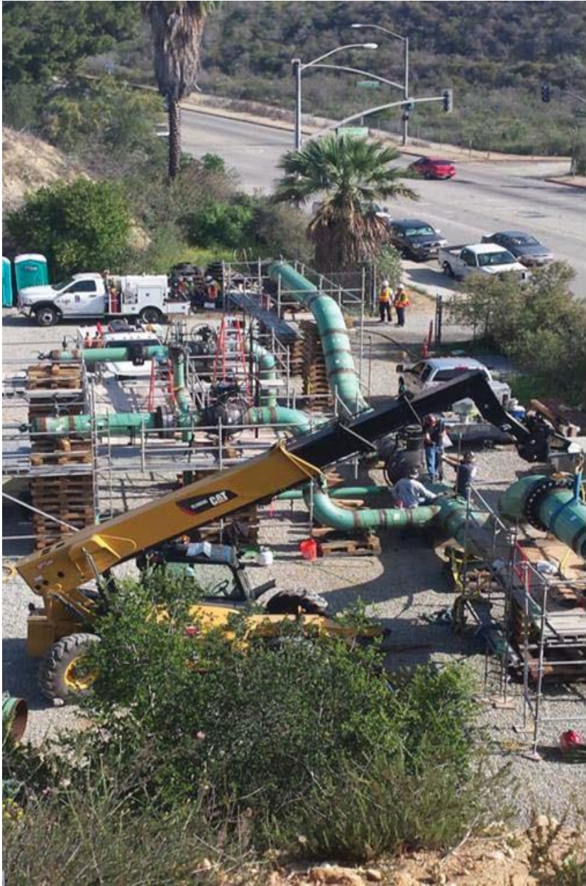
Figure 10: Above-Ground Pre-Fabrication of Valve Assembly
