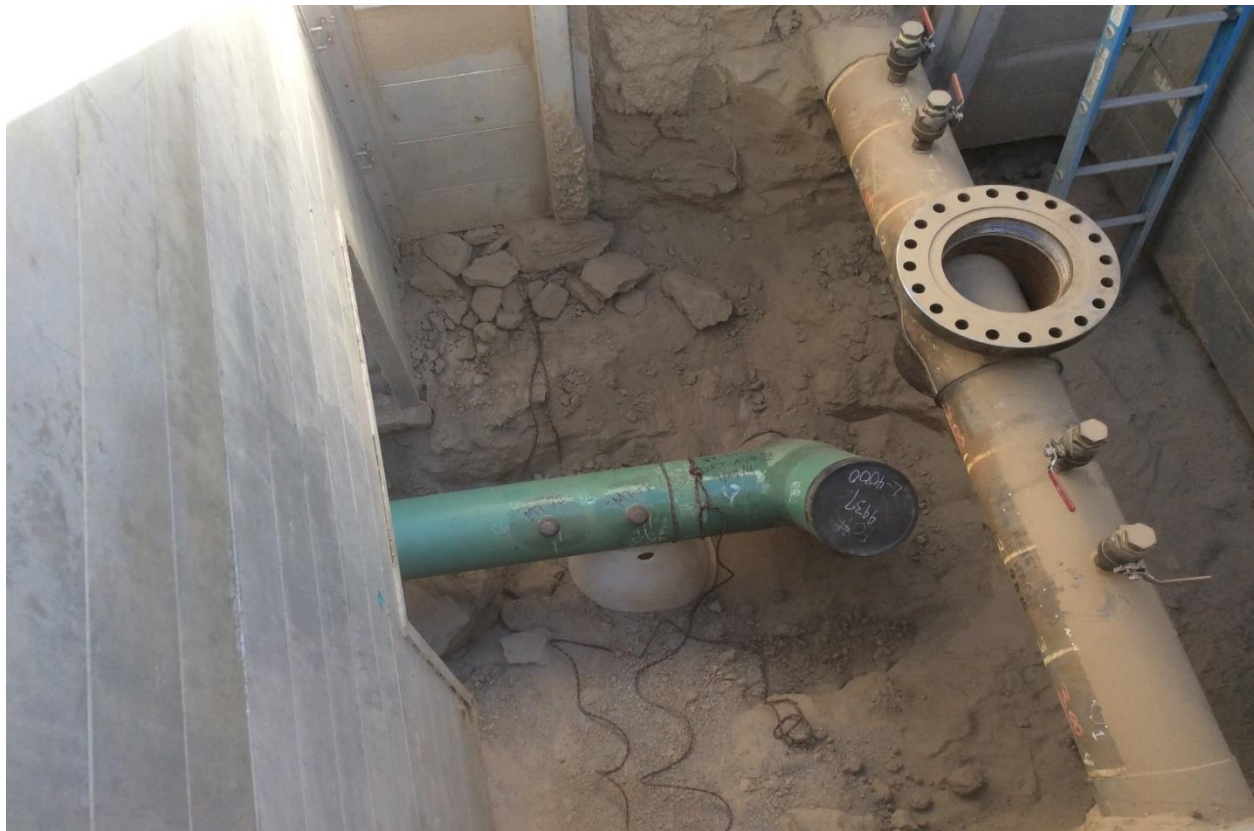
Figure 3: Fit Up in Process to [REDACTED] Bottom Out Stopple Fitting
