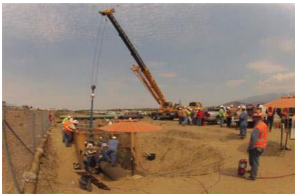
Figure 14: L-2000 Tie-In Construction
