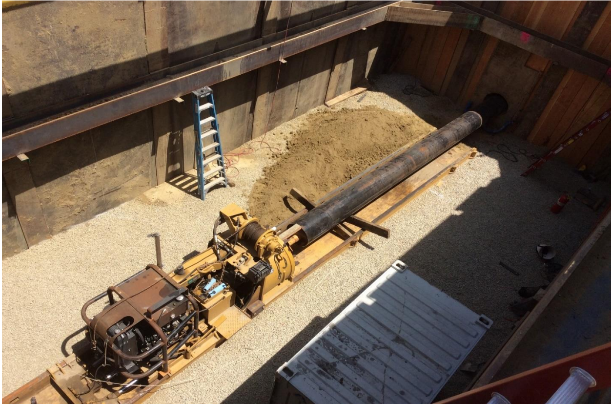
Figure 6: Jack-and-Bore Construction Set Up
