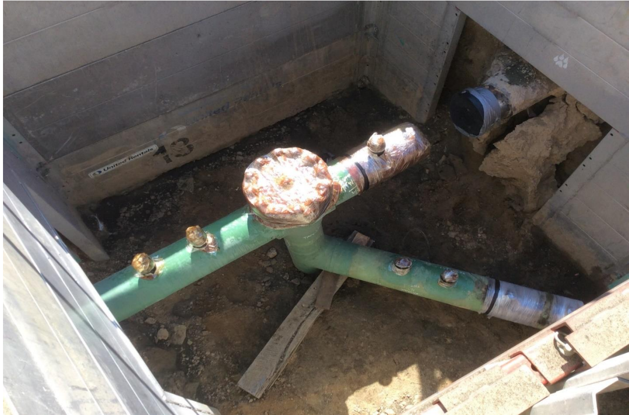
Figure 9: Fittings Wrapped
