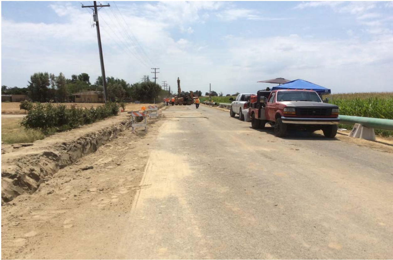
Figure 10: Elm Avenue During Construction
