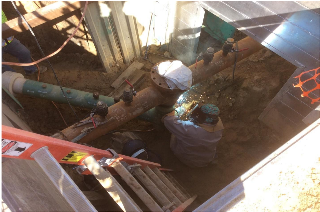
Figure 5: Tie-In to Existing [REDACTED] Line
