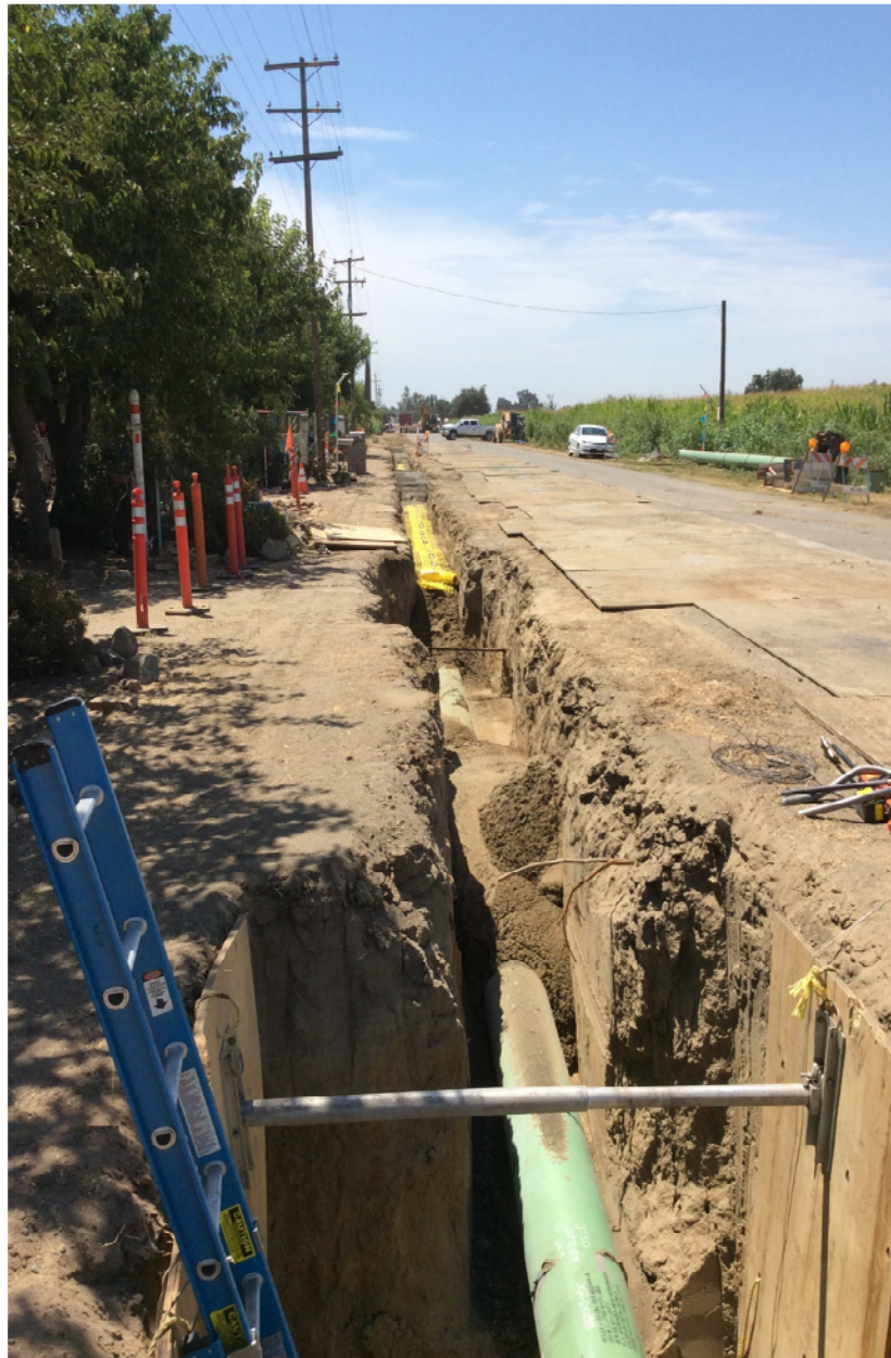
Figure 11: Backfilling the Pipeline Trench
