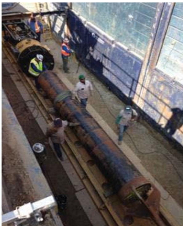
Figure 8: Jack and Bore Operation
