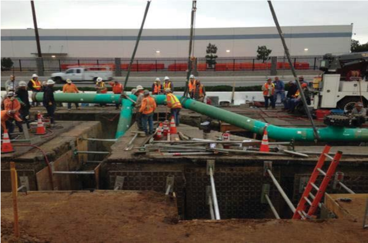
Figure 9: Lowering Section of Pipe into Trench
