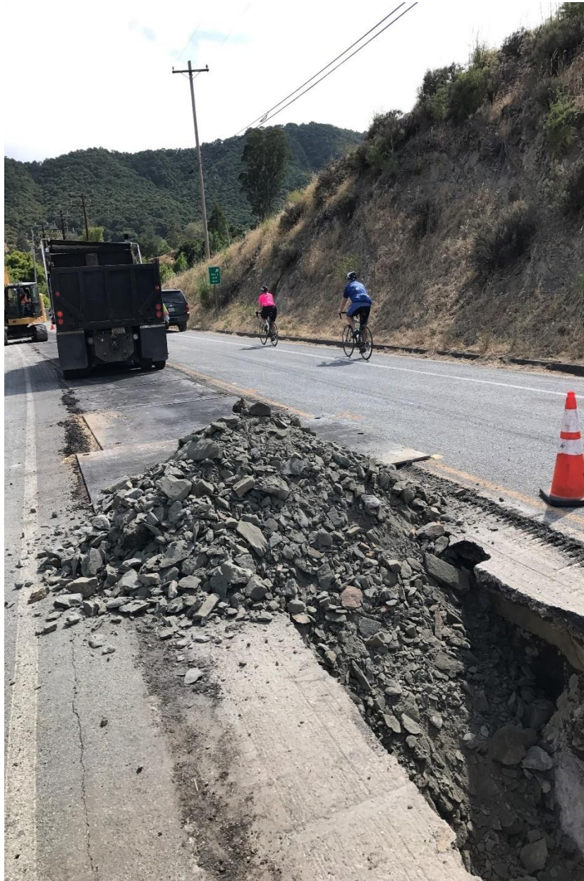
Figure 10: Broken Rock for New Pipe Installation
