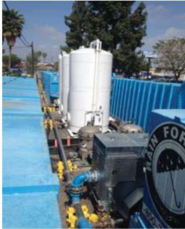
Figure 12: Hydrotest Set Up with Sound Proofing to Minimize Noise Complaints (located behind Baker tank)
