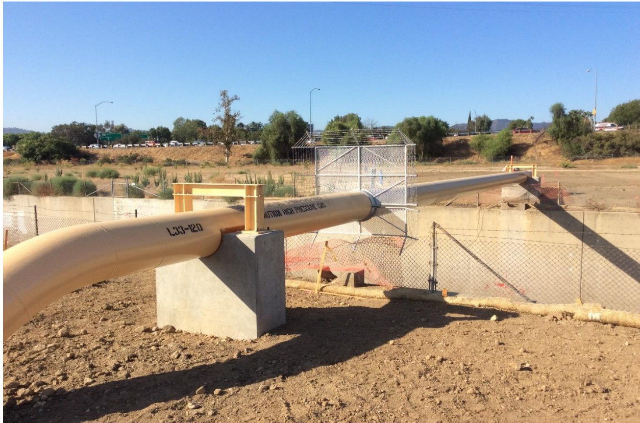
Figure 4: Span Crossing of Replacement Pipeline
