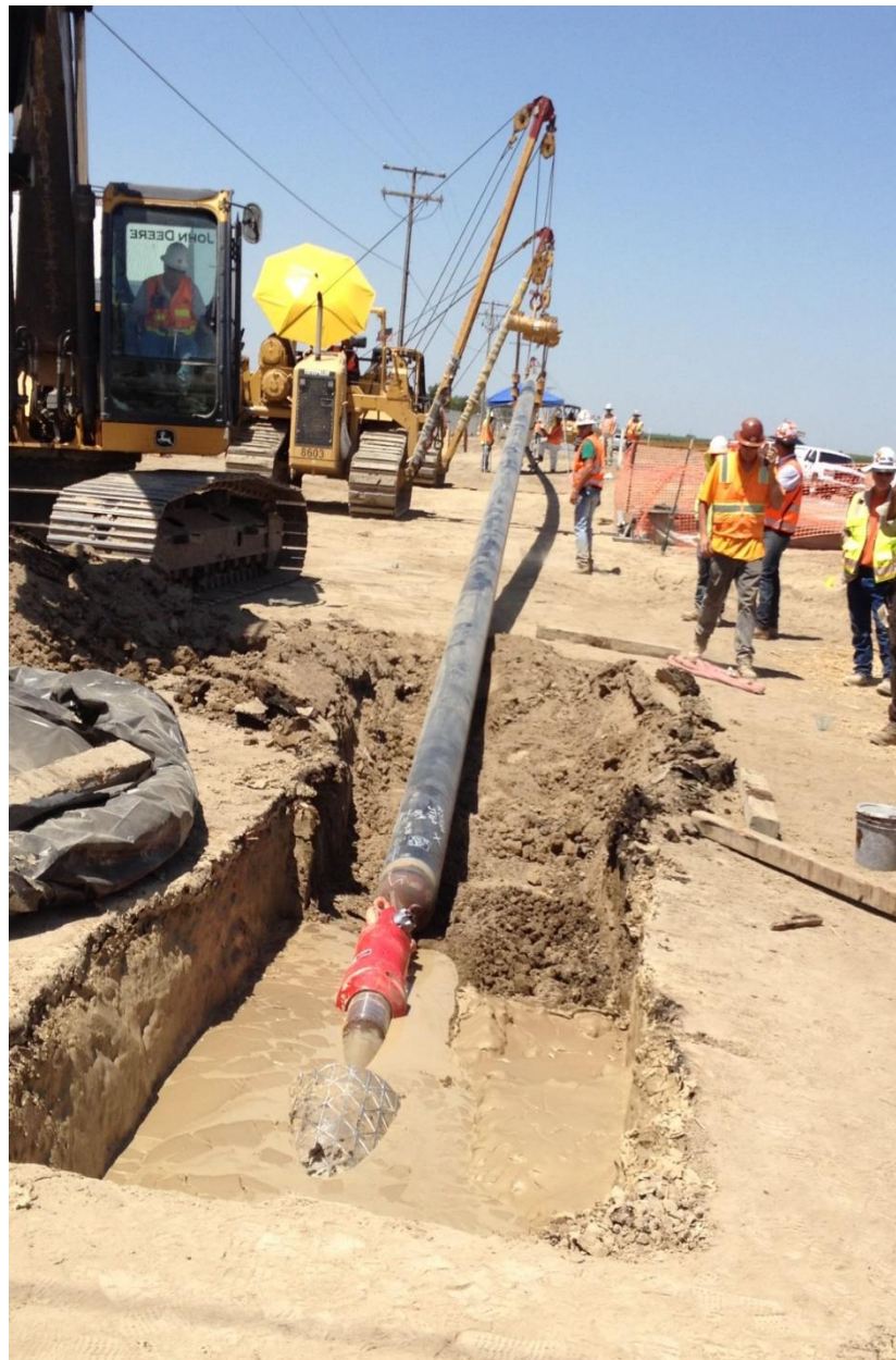
Figure 3: HDD Pullback String Installation
