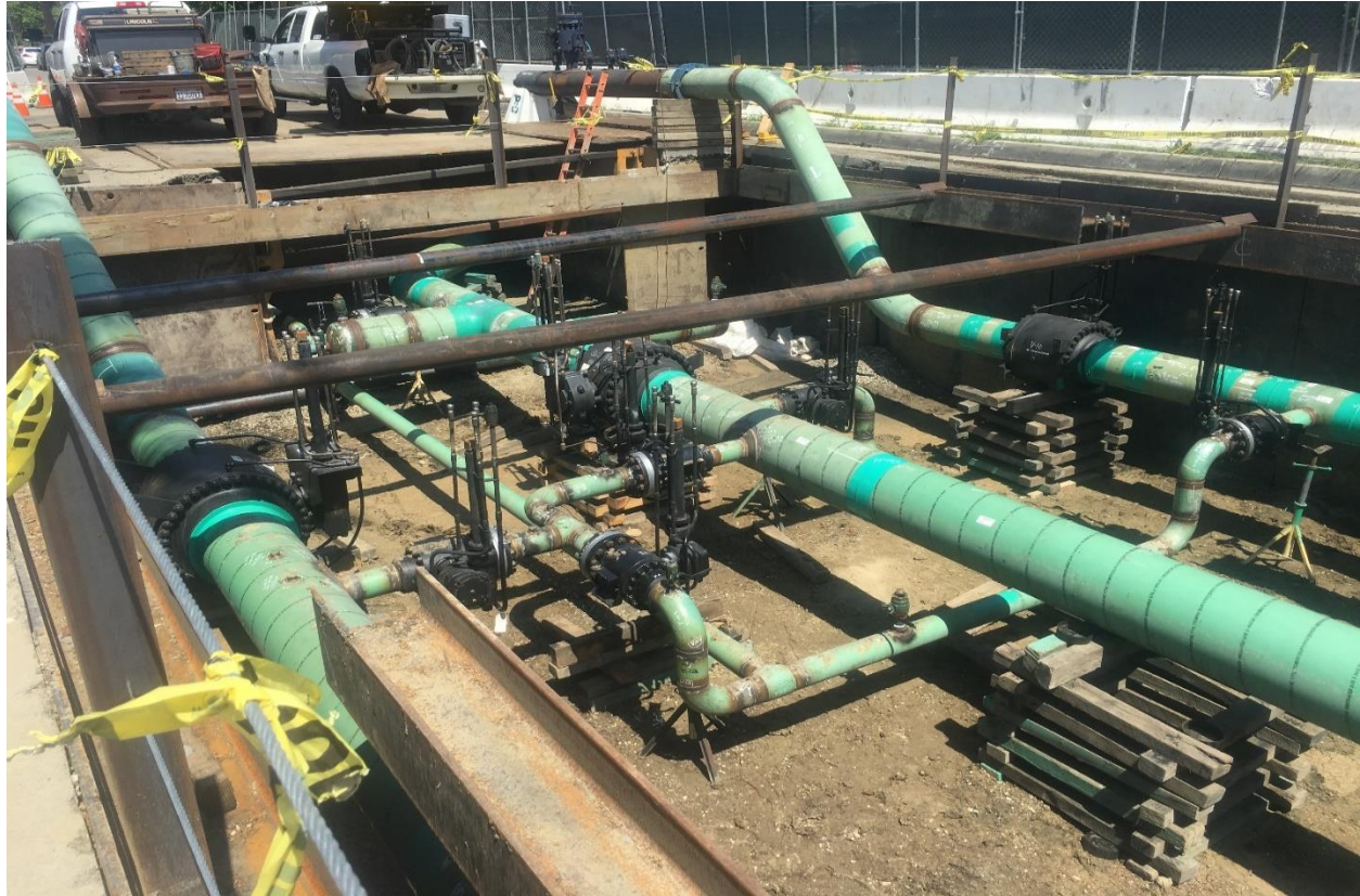
Figure 7: Replacement Bridle Configuration During Construction
