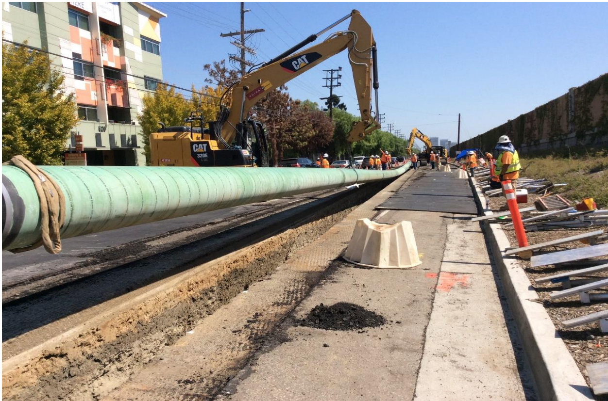
Figure 5: Installing Pipe String into Trench
