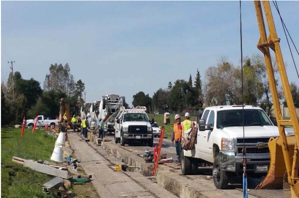
Figure 5: Slurrying New Pipeline
