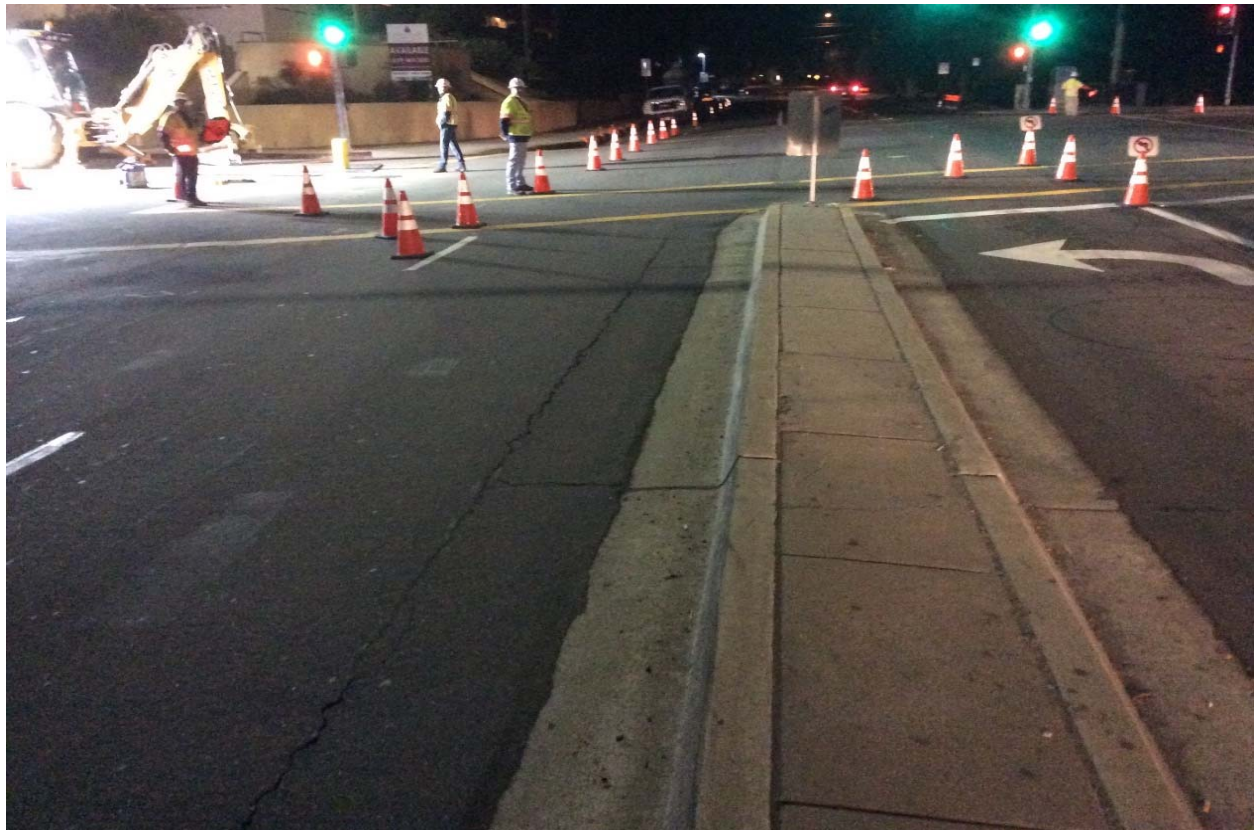
Figure 13: Traffic Control in Place
