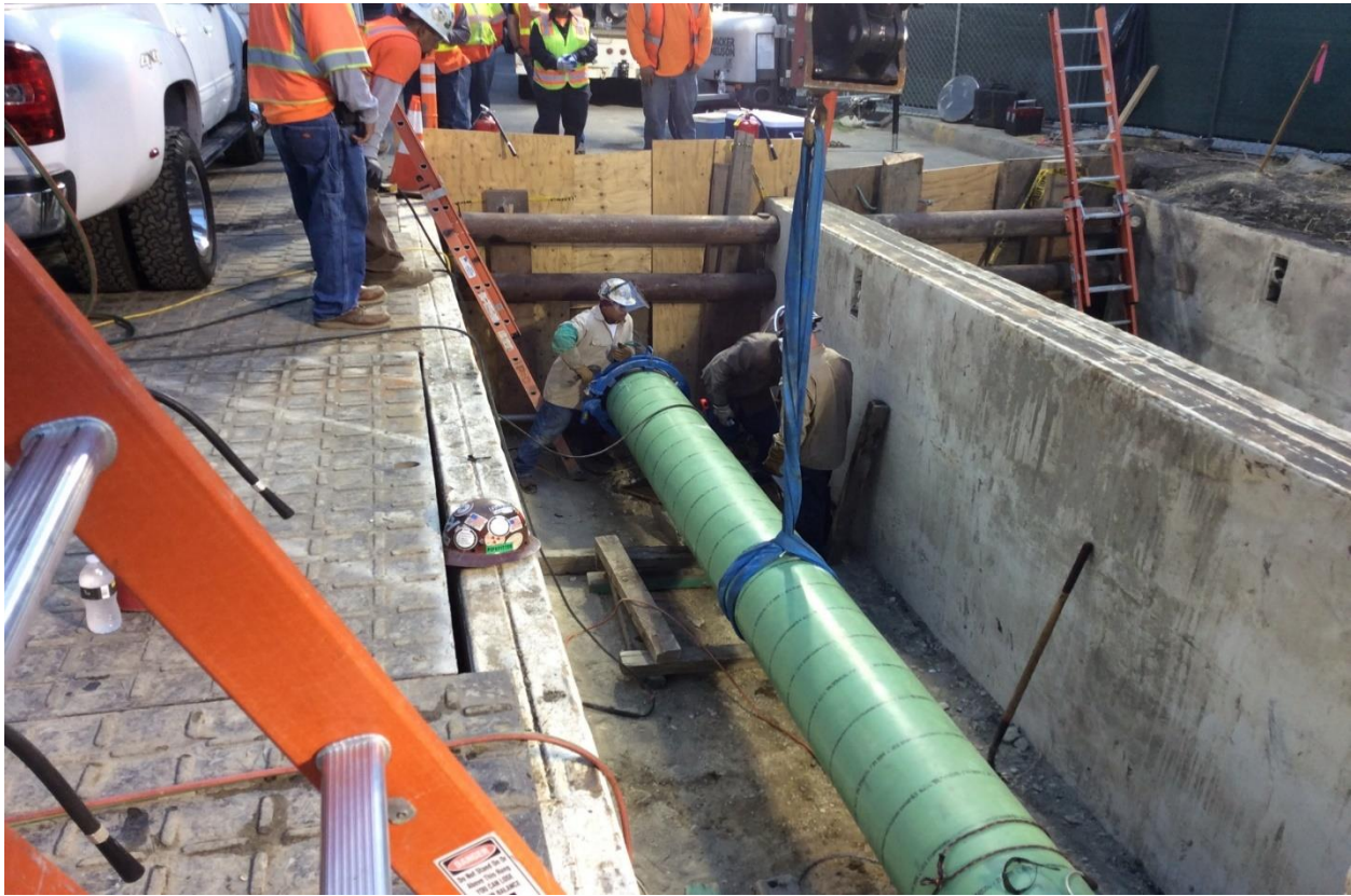
Figure 8: Lowering Tie-in Piece at Burbank Boulevard
