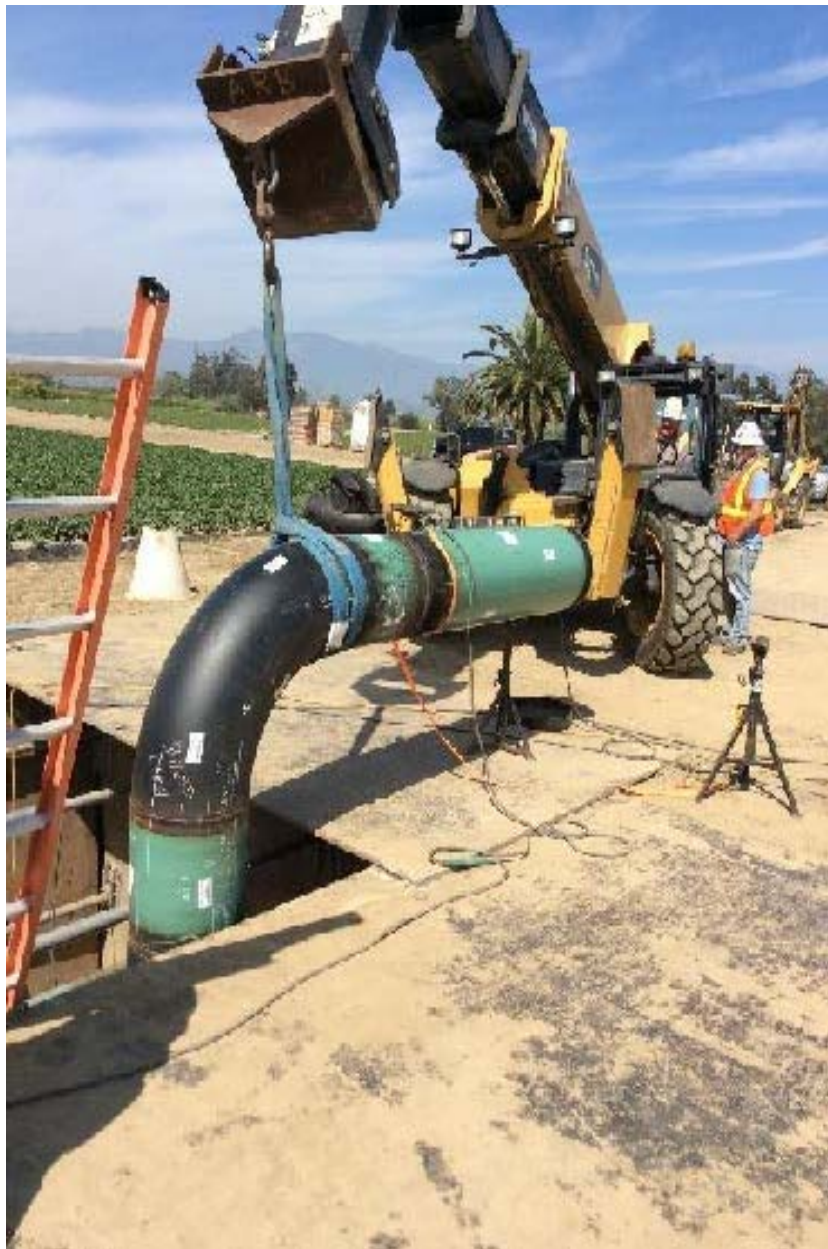
Figure 21: Section 3 Test Head Loop Being Lowered at MLV Site
