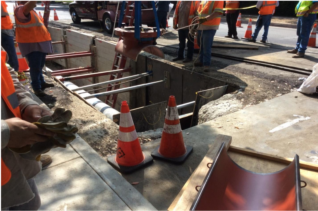
Figure 5: Lowering Top Half of Stopple Fitting at Garfield Avenue
