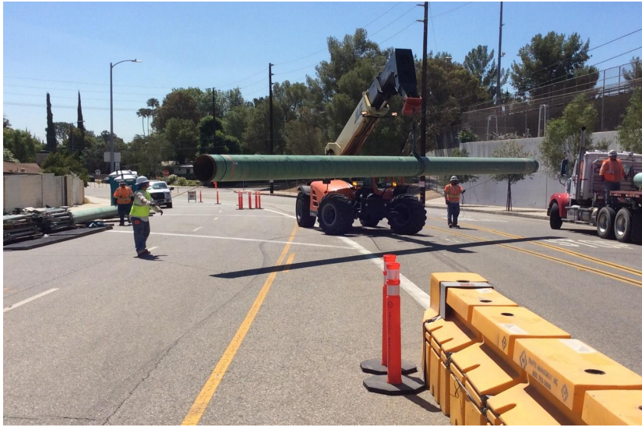
Figure 4: Unloading Pipe at East Laydown Yard
