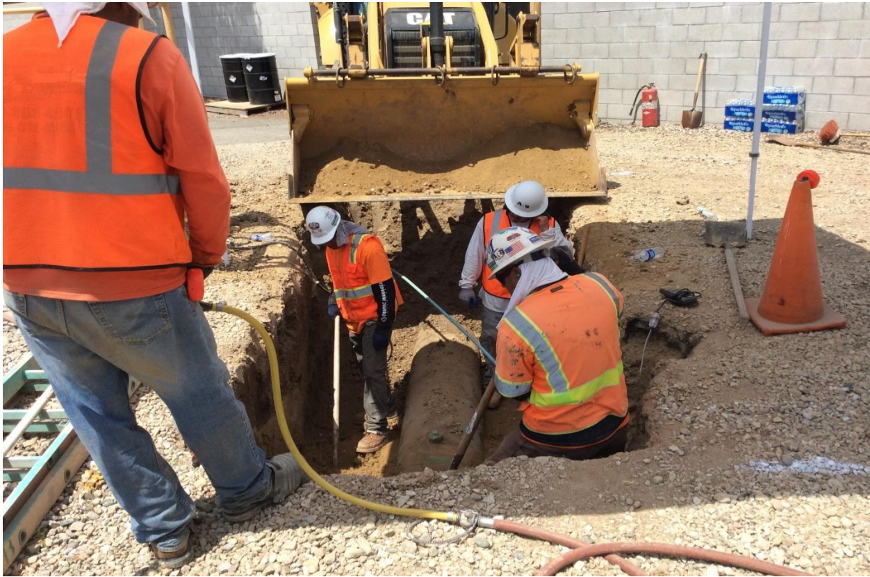
Figure 3: Exposing Line 406 at Westside Station
