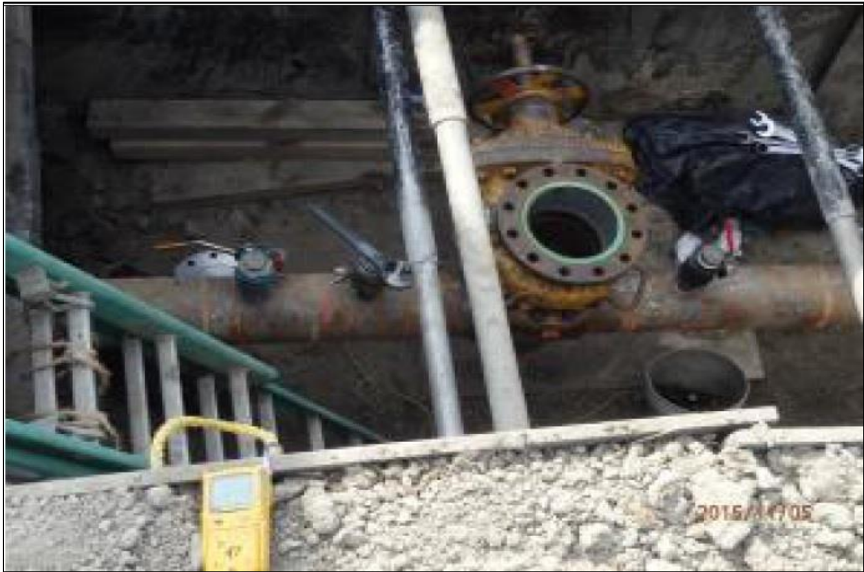
Figure 4: PCF Installation to Complete Abandonment
