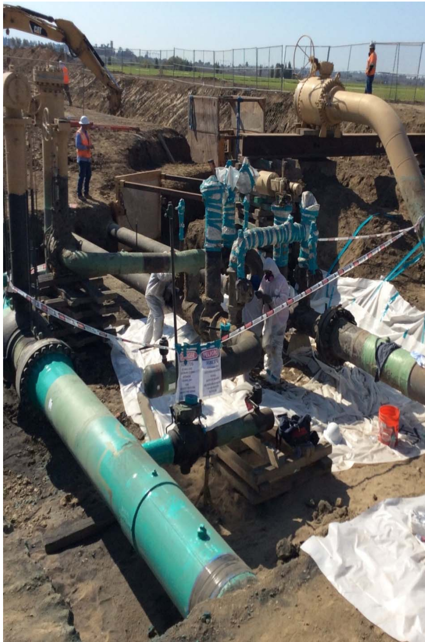
Figure 23: Section 3A Abatement Activities of MLV Removal
