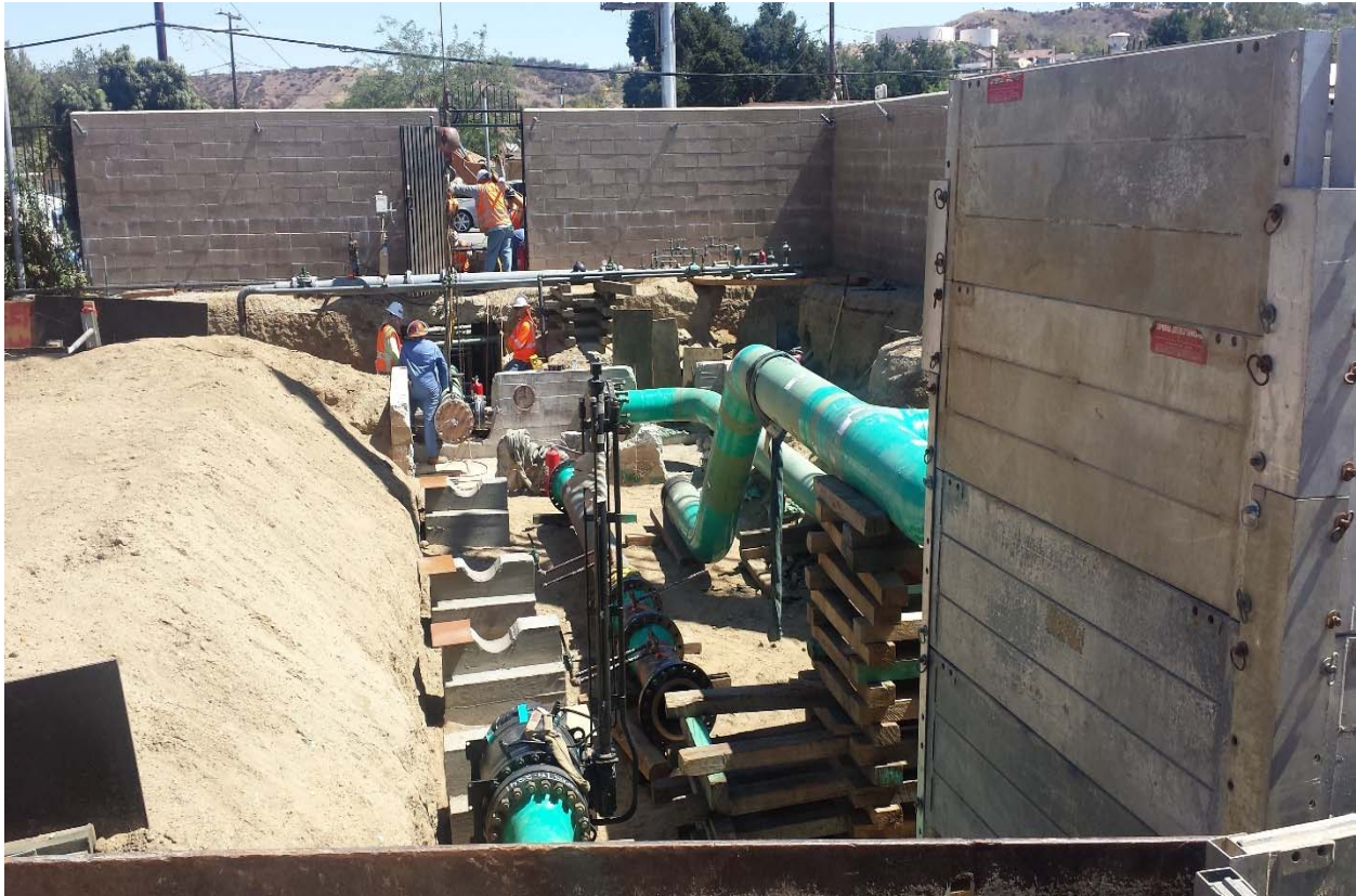
Figure 7: Construction within the Station
