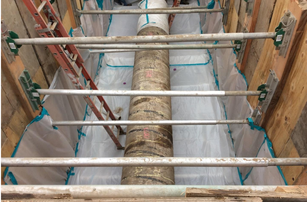
Figure 5: Preparation of Bell Hole for Coating Abatement
