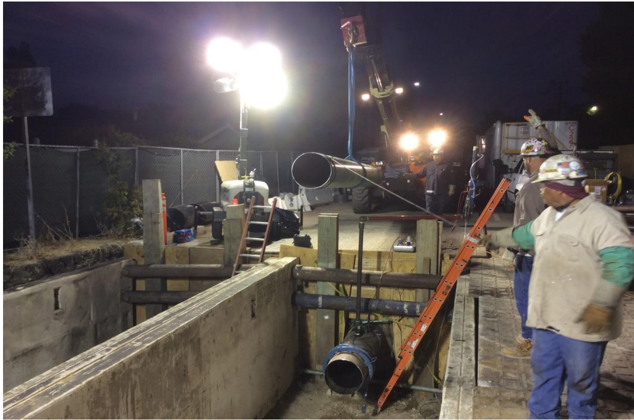
Figure 7: Crew Lowering Tie-in Piece at Burbank Boulevard
