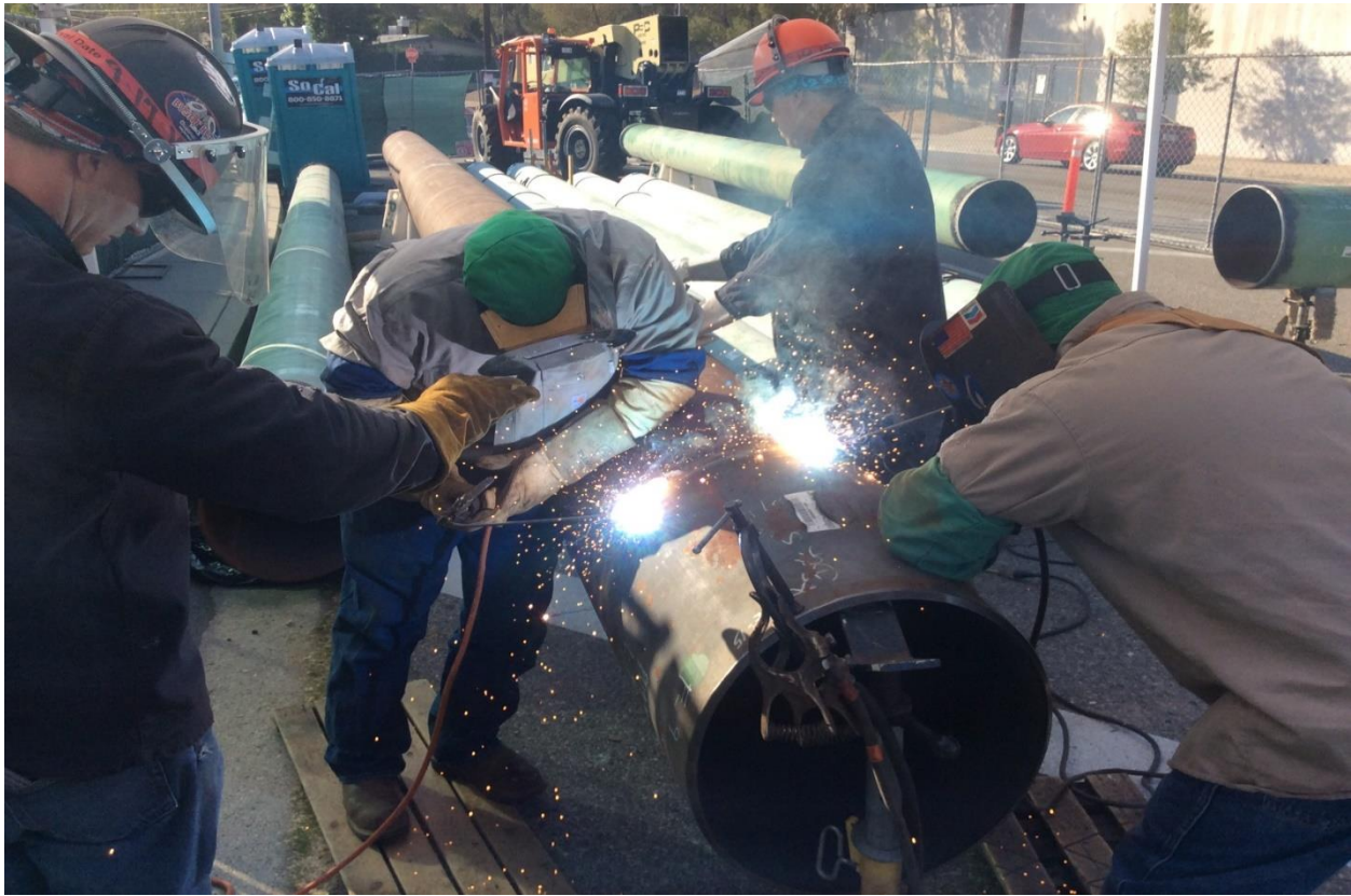
Figure 5: Fabricating Test Loops
