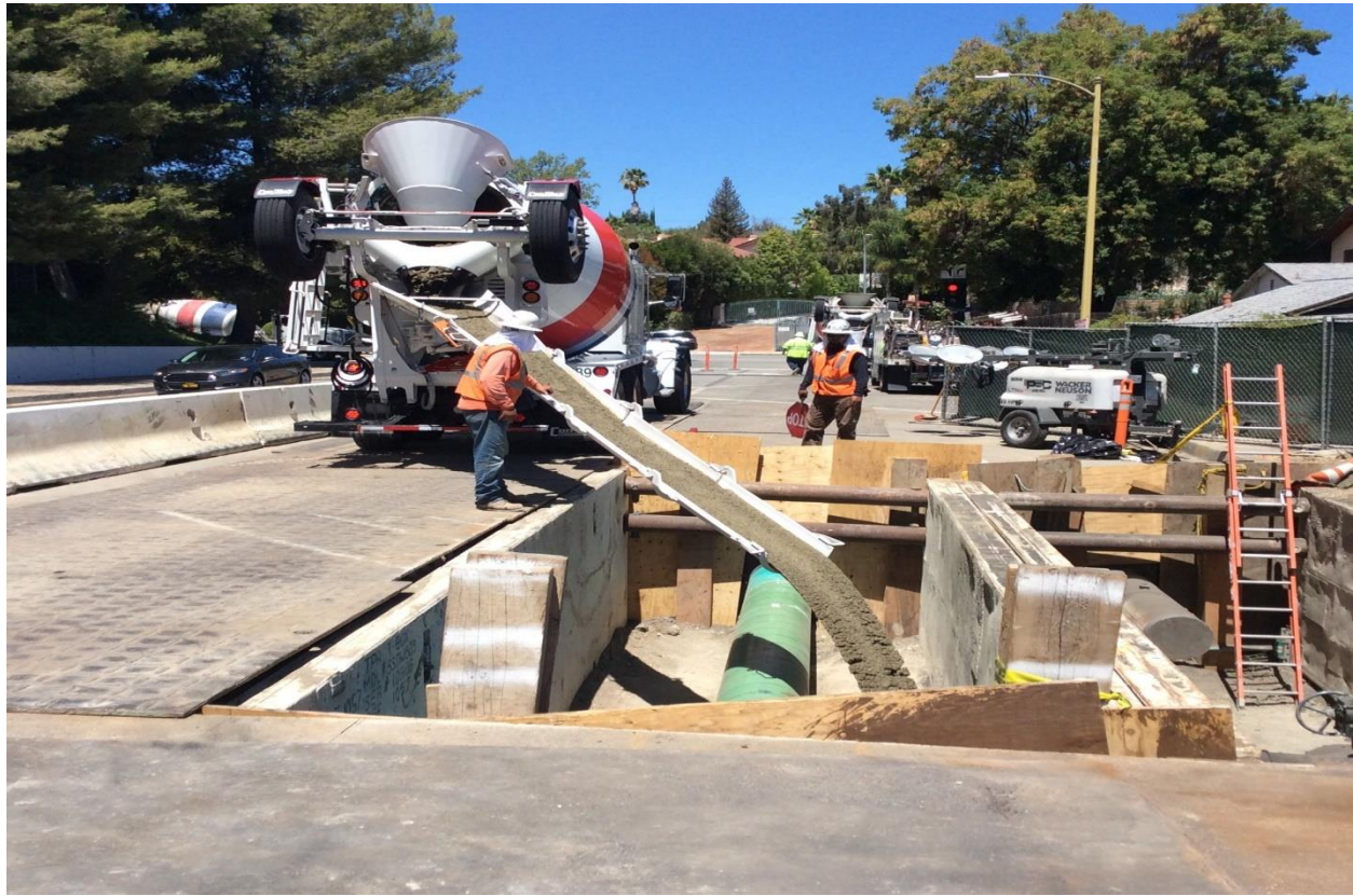
Figure 10: Backfilling Bell Hole Line 406 at Burbank Boulevard
