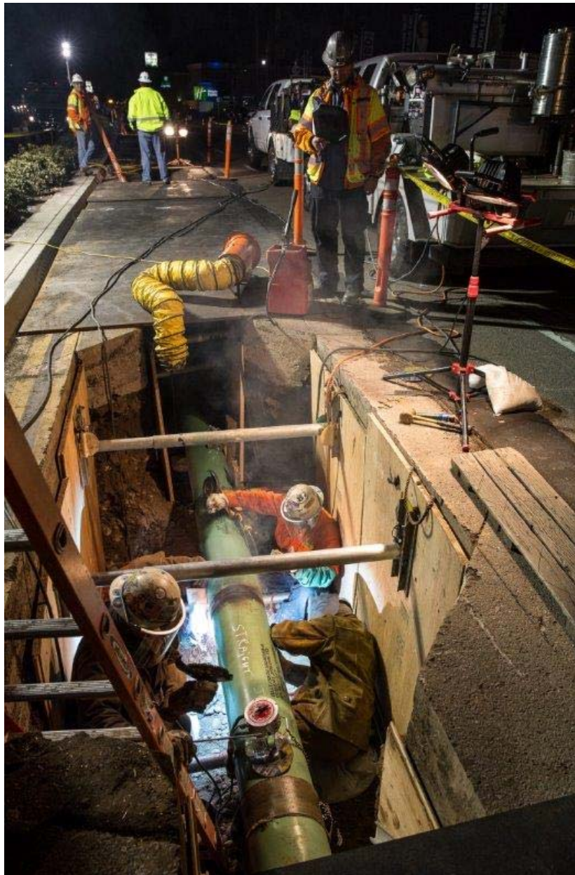
Figure 8: Night Work on Mission Bay Drive
