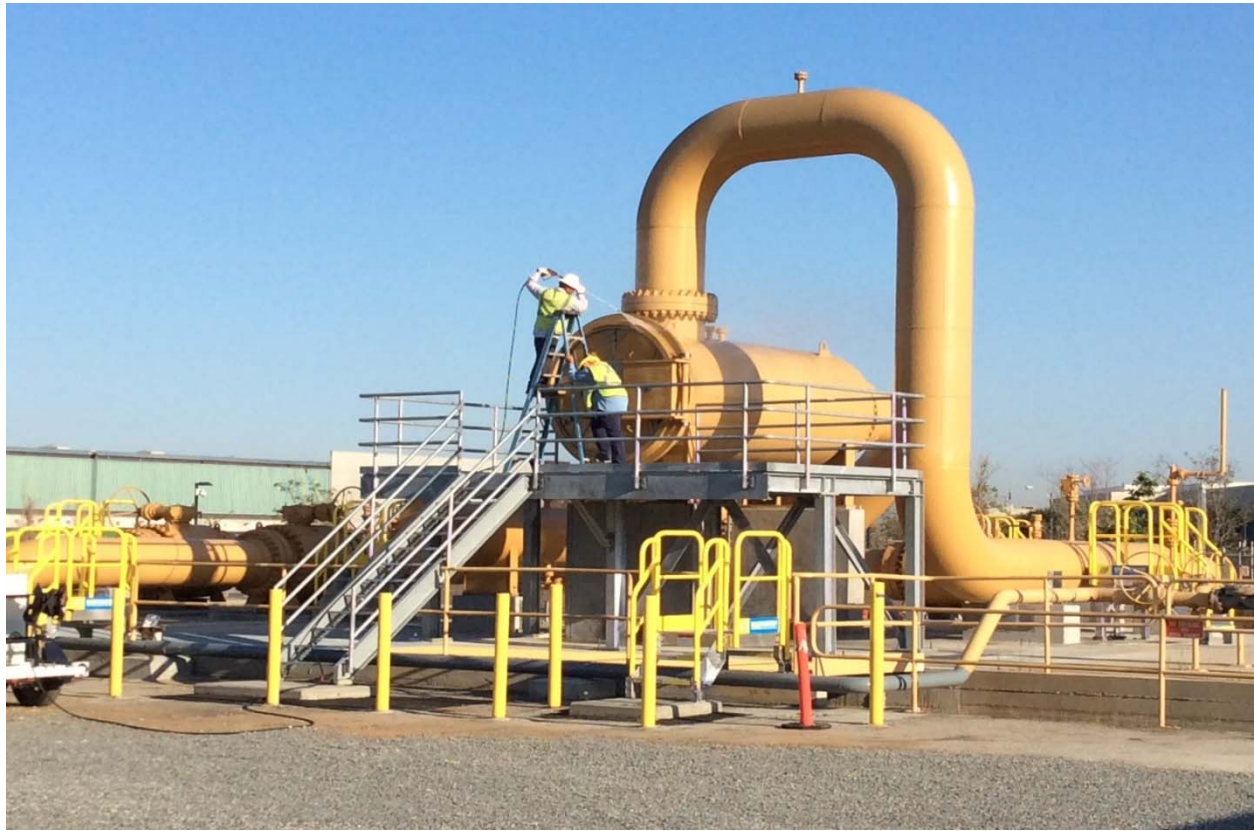
Figure 9: New Filter Separator
