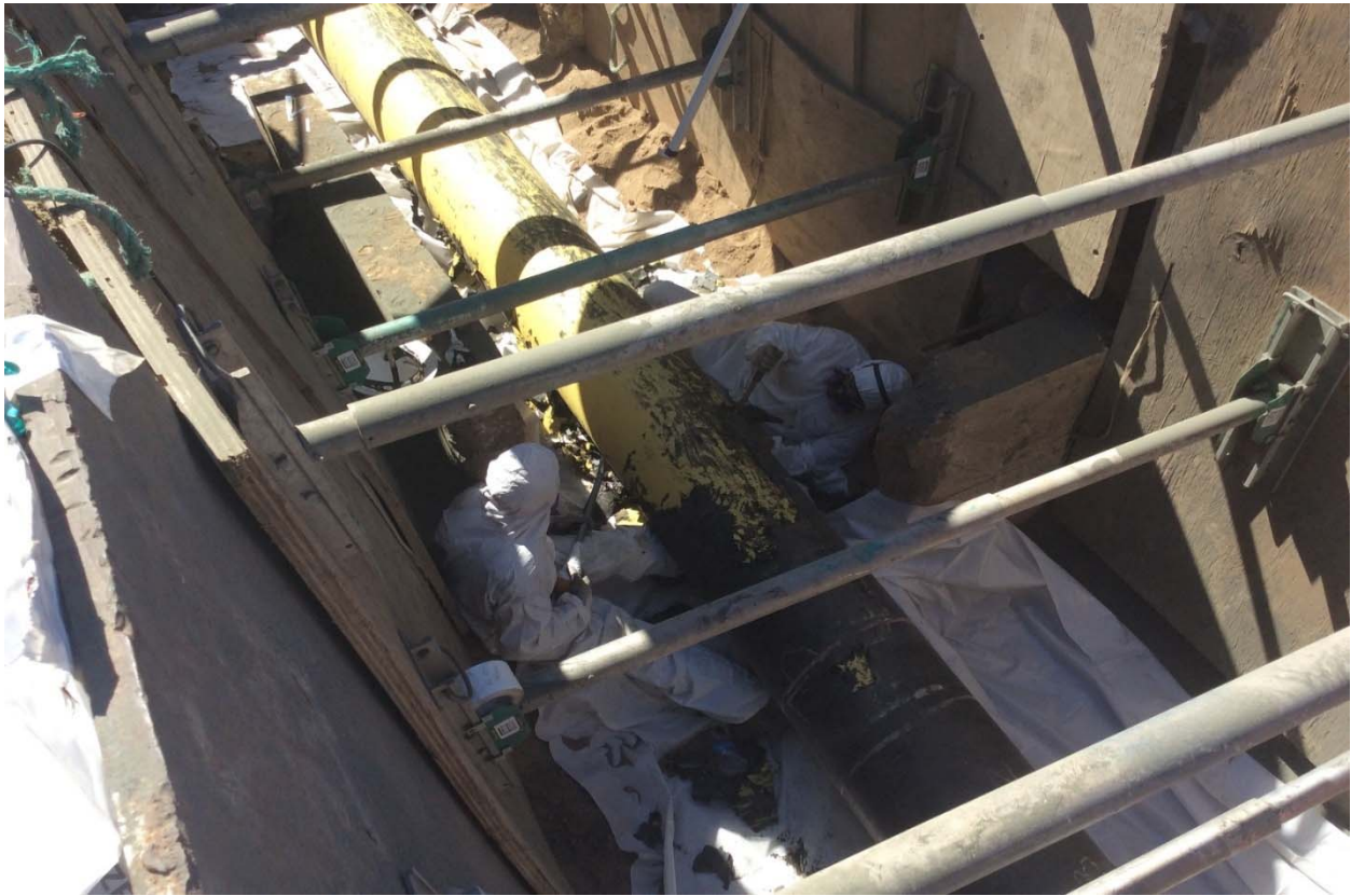
Figure 14: Section 1 Abatement Activities
