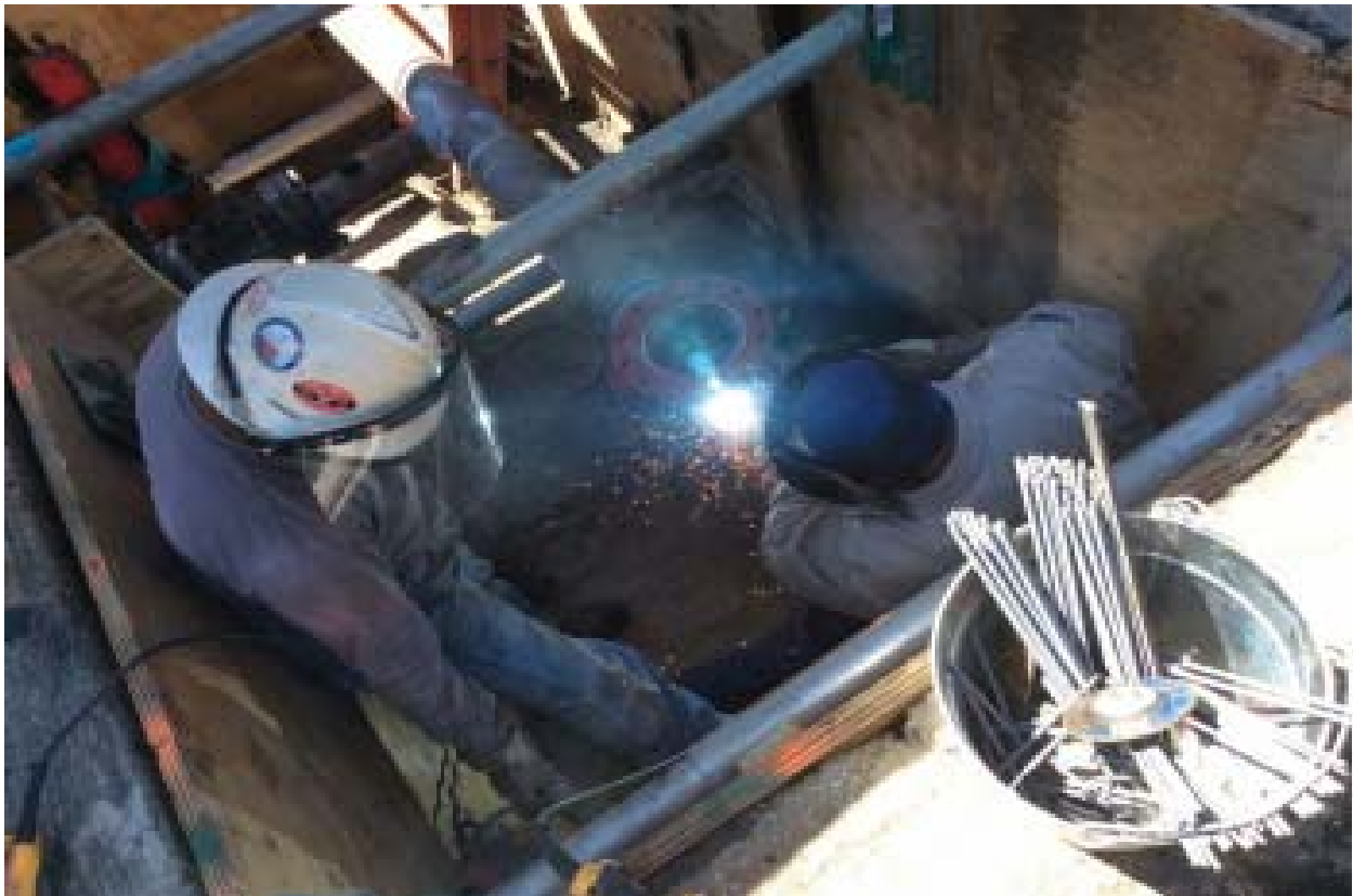
Figure 7: Installation of a Bottom Out Fitting
