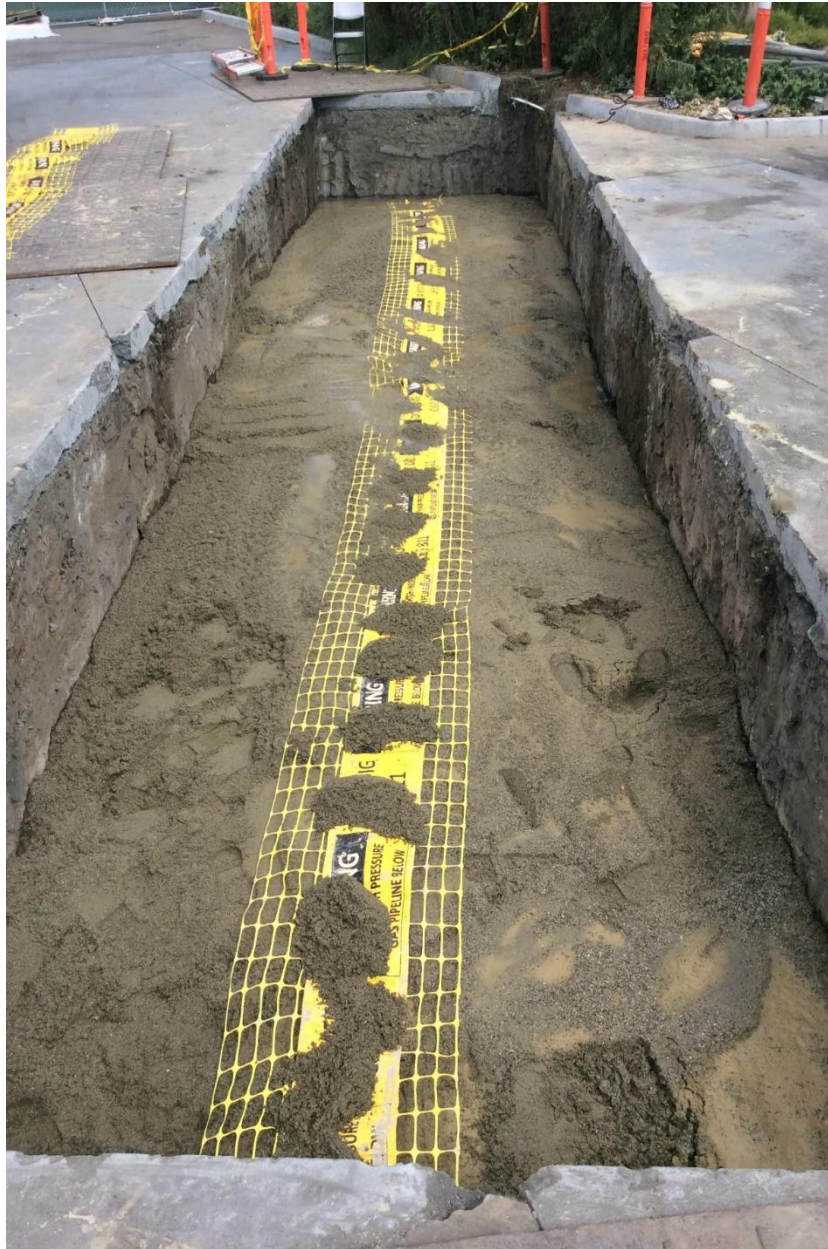
Figure 8: Excavation Backfill with Slurry and Warning Mesh
