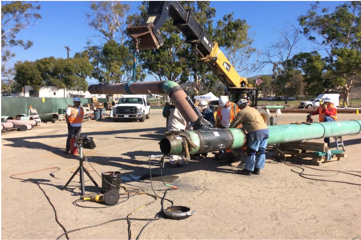
Figure 15: Section 1 Pre-fabrication of Replacement Pipe
