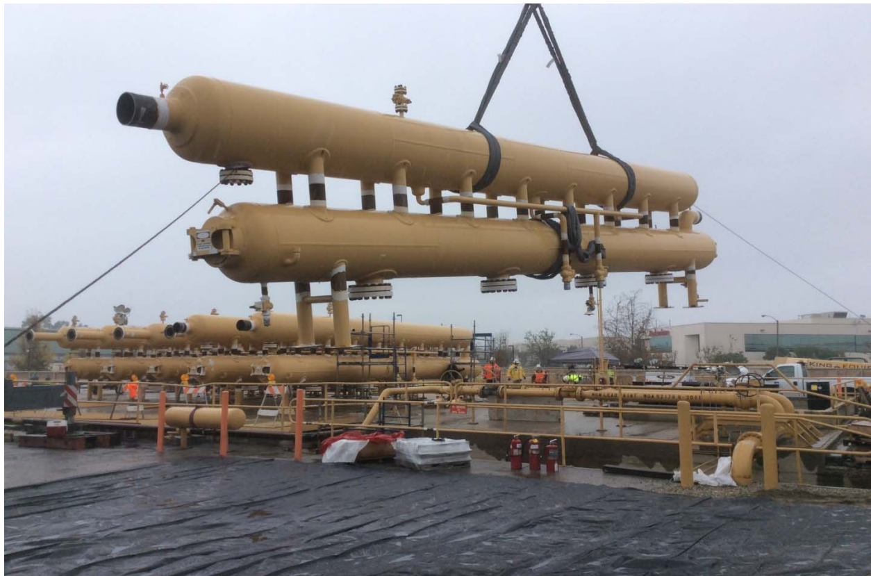
Figure 5: One (of Seven) Scrubber Assemblies Being Removed
