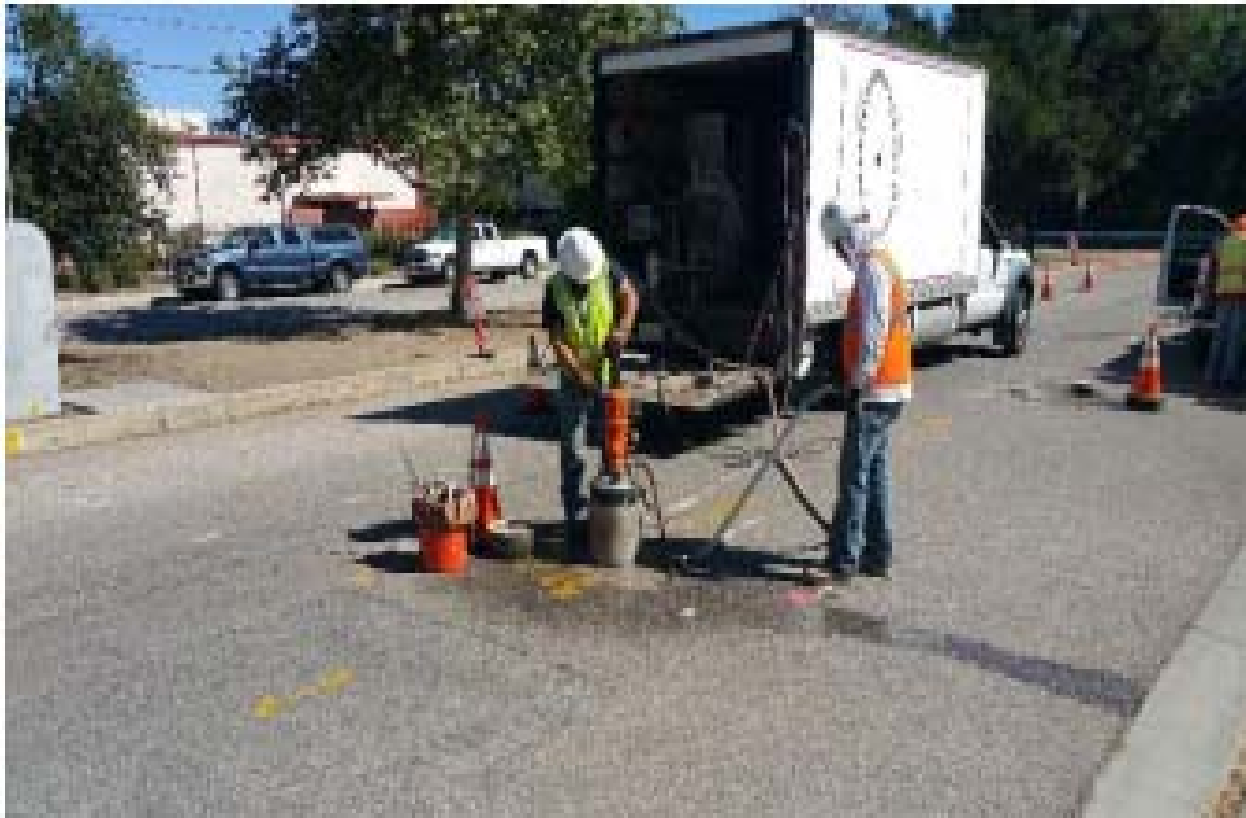
Figure 6: Potholing Operation
