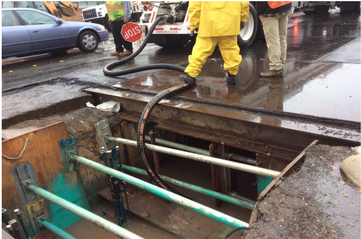
Figure 10: Pumping Water from Bellhole
