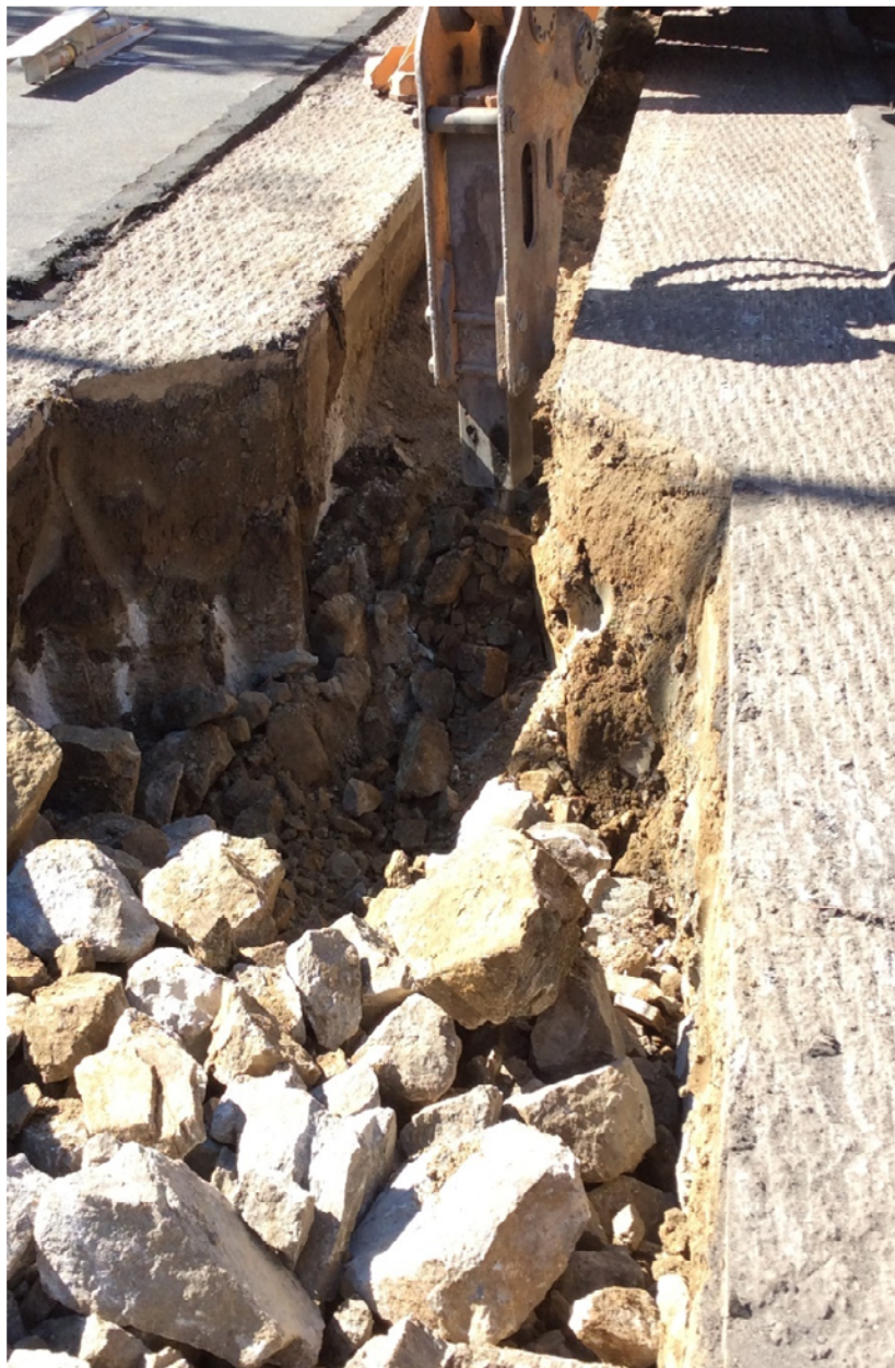
Figure 12: Breaking Rock (Granite)
