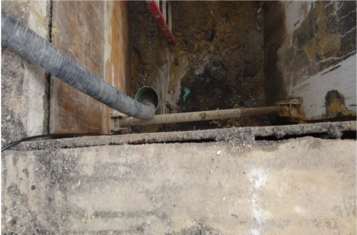
Figure 10: Groundwater Mitigation
