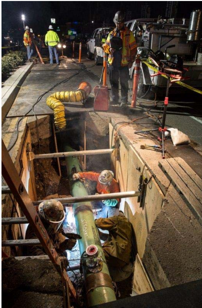
Figure 8: Night Work on Mission Bay Drive
