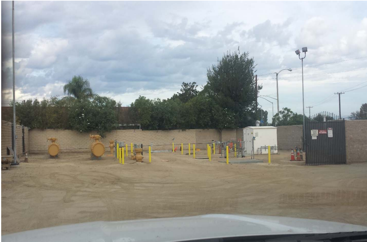
Figure 8: Station after Construction
