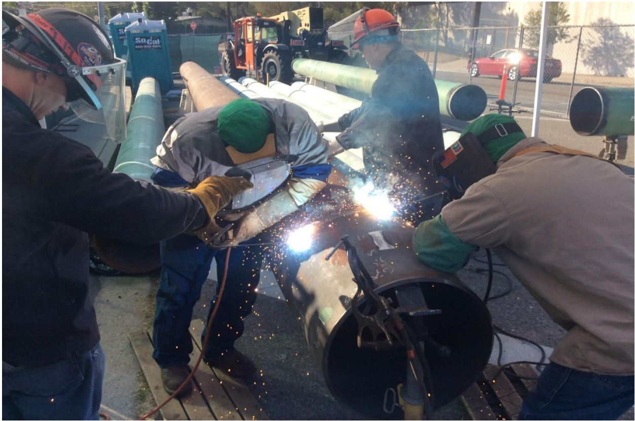
Figure 5: Fabricating Test Loops
