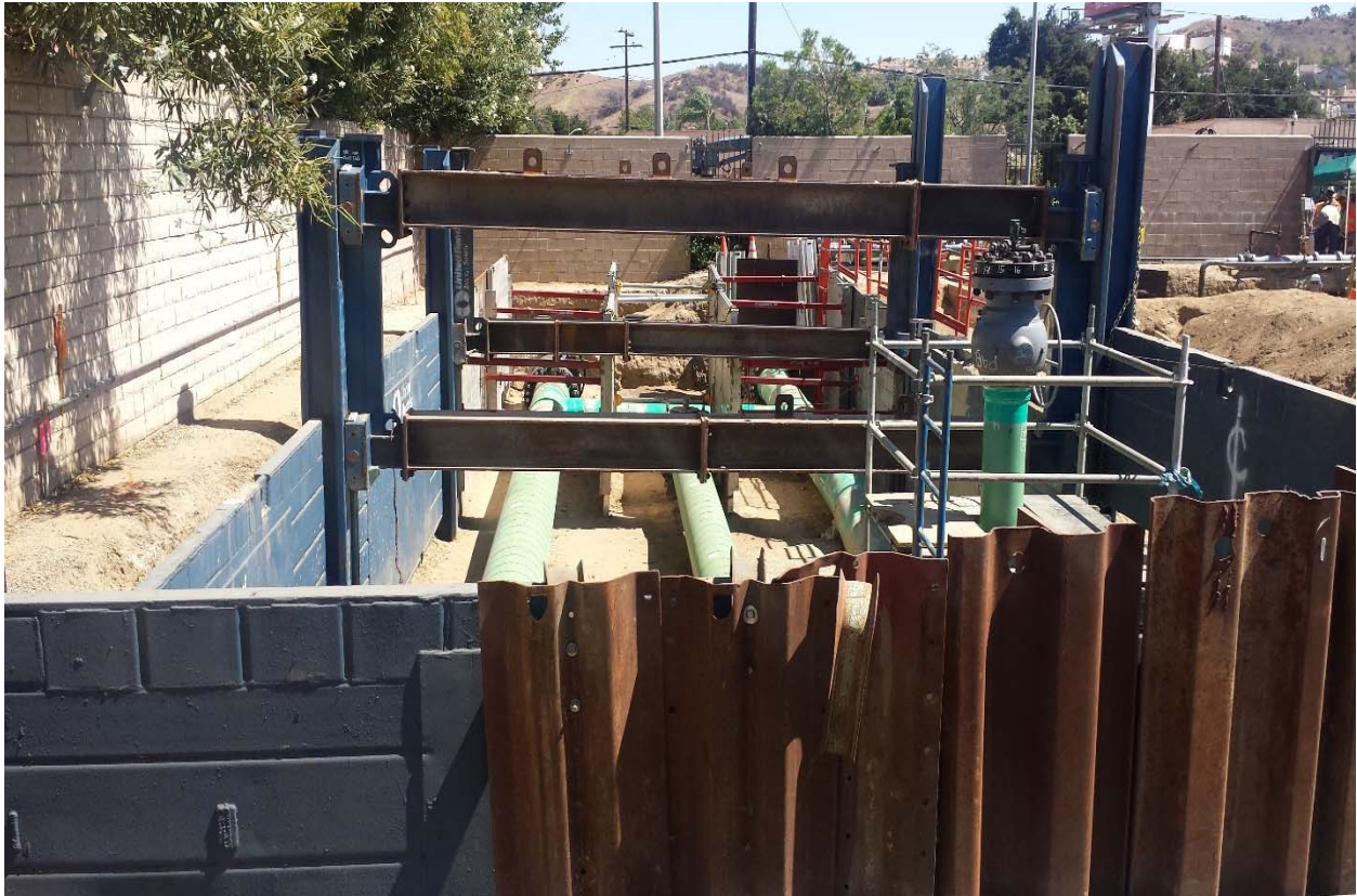
Figure 6: Shoring During Construction within Station
