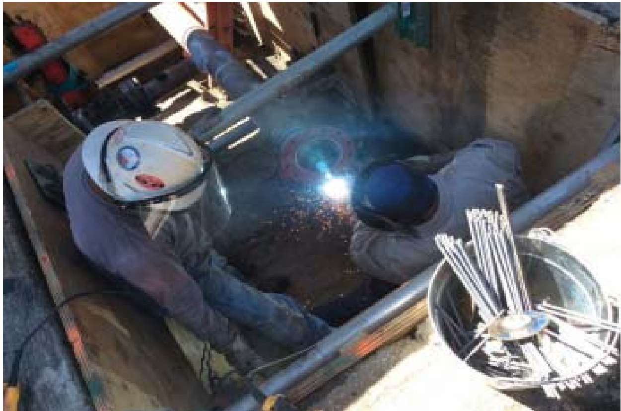
Figure 7: Installation of a Bottom Out Fitting
