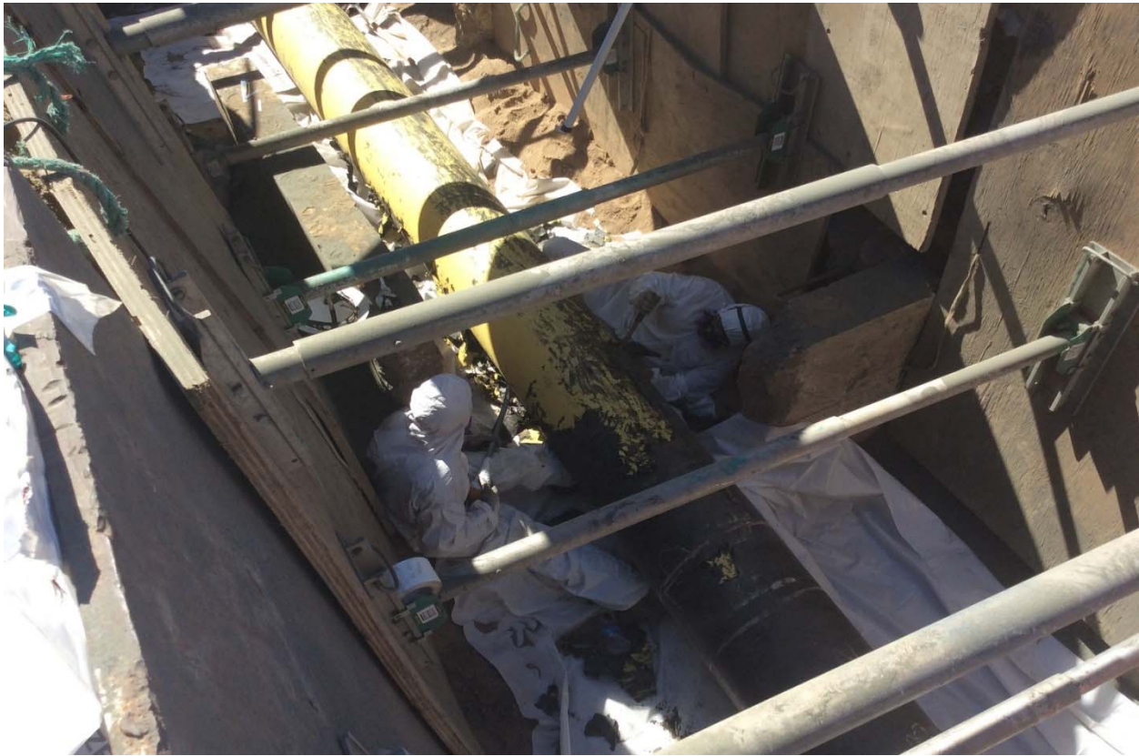
Figure 14: Section 1 Abatement Activities
