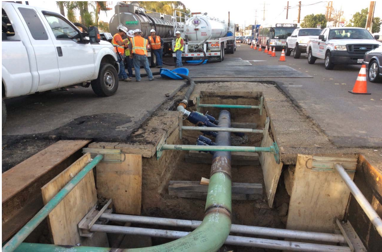
Figure 11: Hydrotest Contractor Setting Fill Pipe
