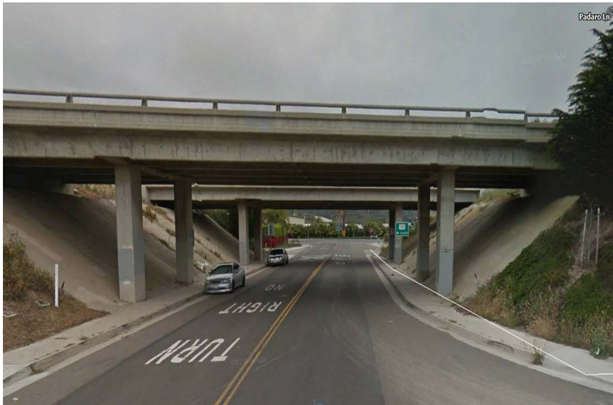
Figure 7: Underpass Site of New Crossover Line 8119
