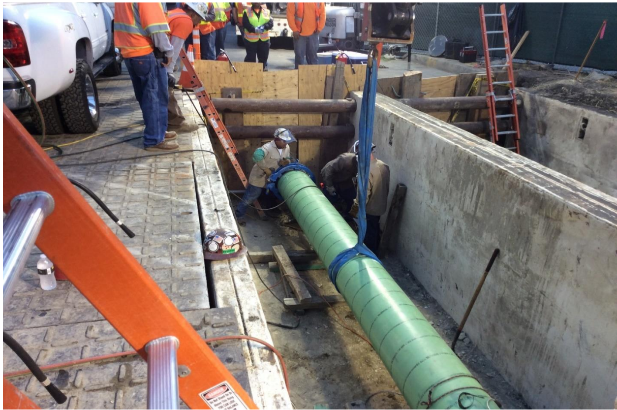
Figure 8: Lowering Tie-in Piece at Burbank Boulevard
