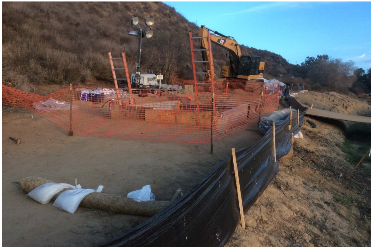
Figure 24: Section 4 and 5 West End Test Head Excavation
