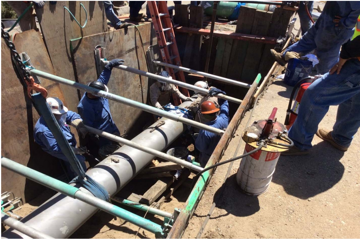
Figure 19: Section 2A Cut and Cap Activities
