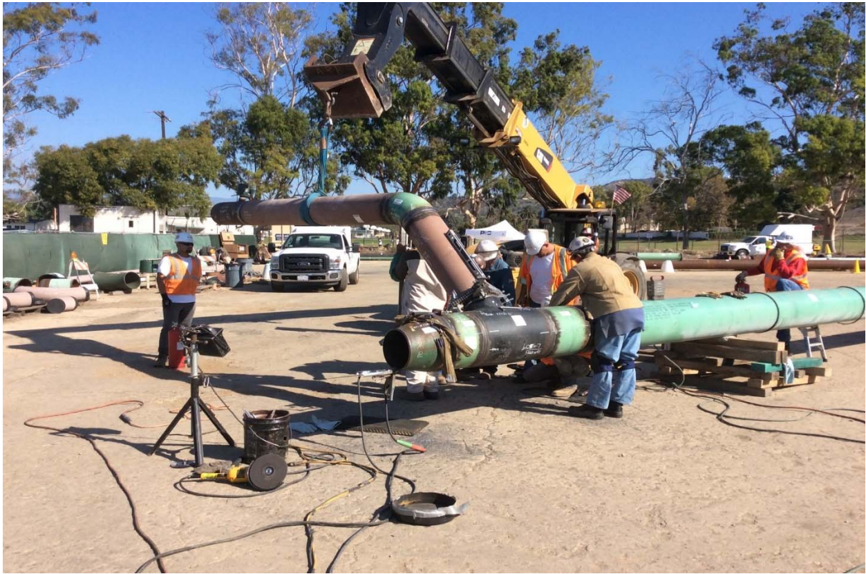
Figure 15: Section 1 Pre-fabrication of Replacement Pipe
