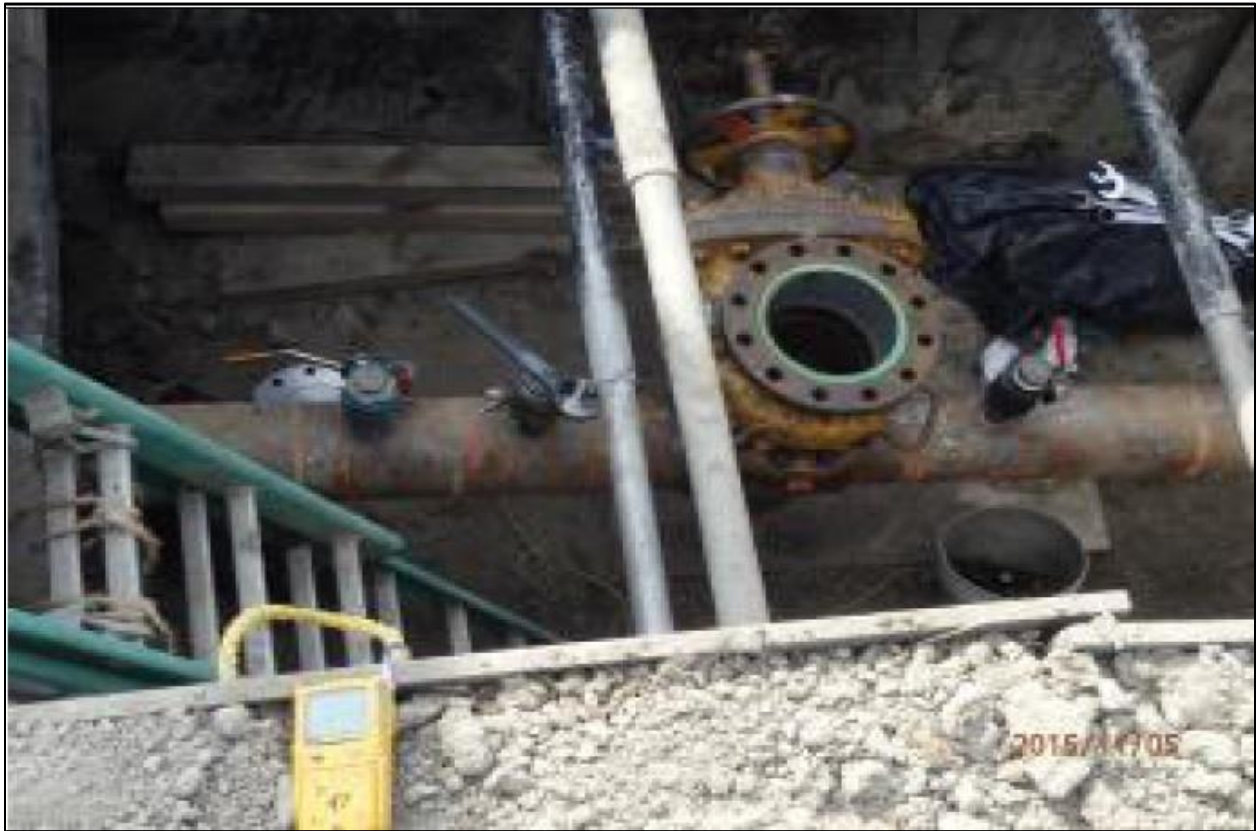
Figure 4: PCF Installation to Complete Abandonment
