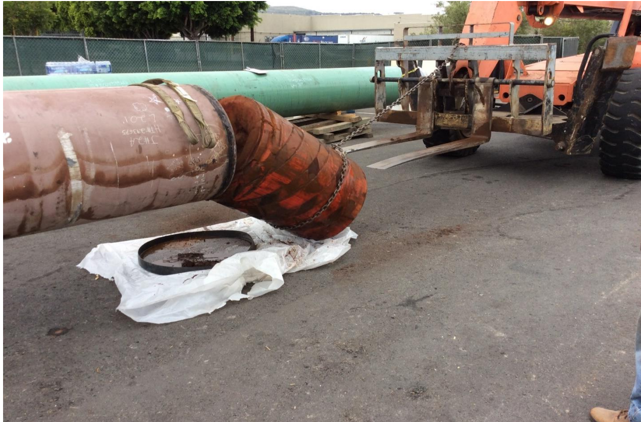
Figure 6: Poly Pig Removal from Test Head
