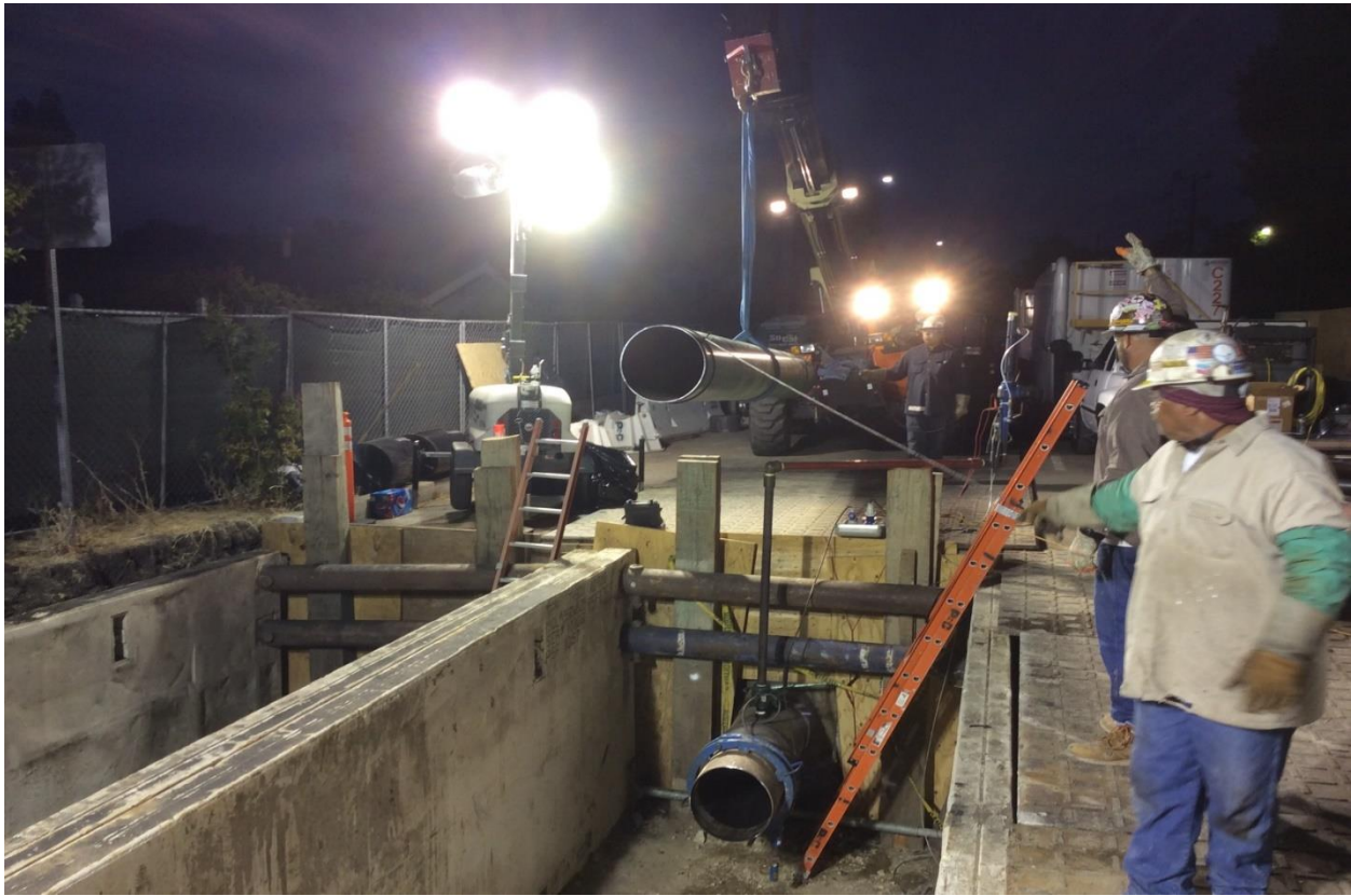
Figure 7: Crew Lowering Tie-in Piece at Burbank Boulevard
