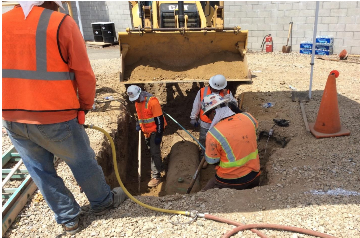
Figure 3: Exposing Line 406 at Westside Station
