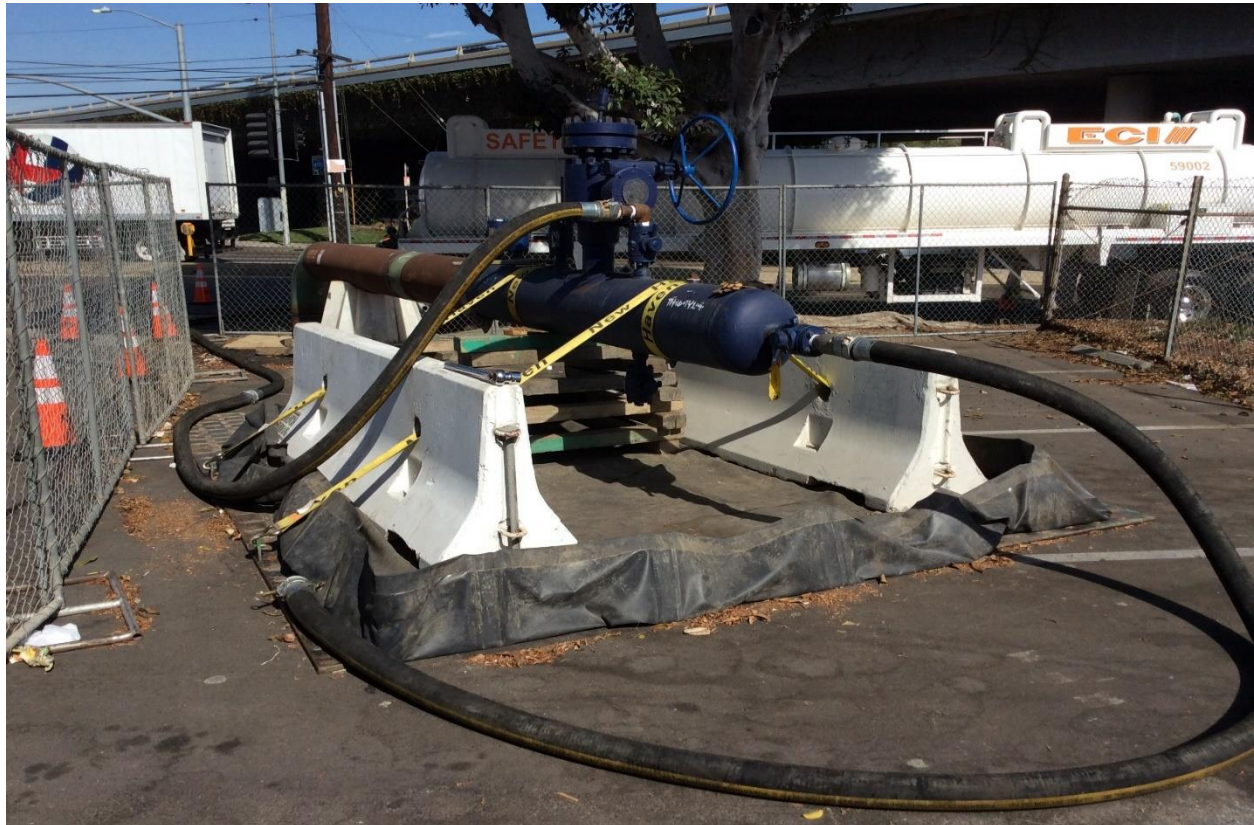
Figure 6: East Test Head Location in Parking Lot During Hydrotest
