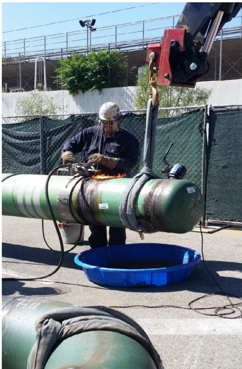
Figure 26: Section 9 Preparation of Isolation Caps
