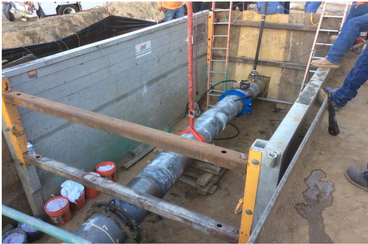
Figure 25: Section 4 and 5 Removal of Existing Pipe Prior to Test Head Installation
