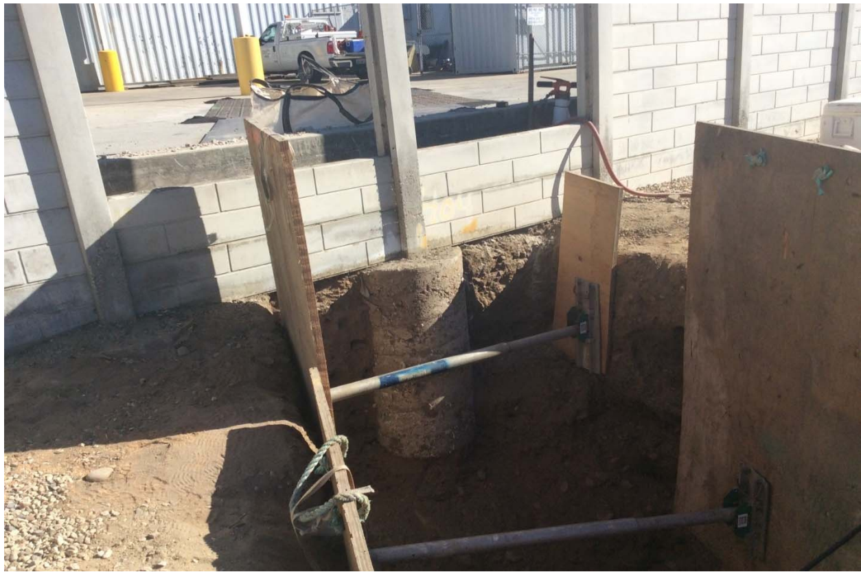
Figure 16: Section 1 Existing Wall Footing Within Trench
