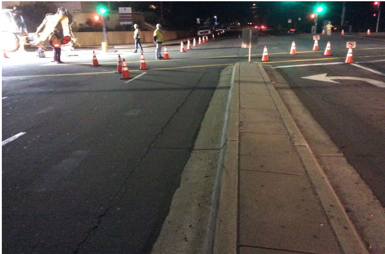
Figure 13: Traffic Control in Place
