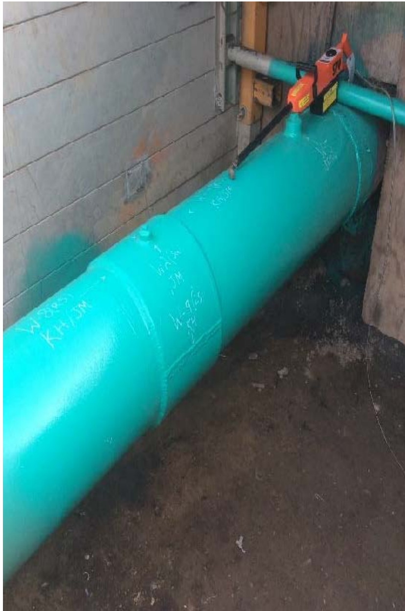
Figure 22: Section 3 Coating Inspection at Tie-in Point
