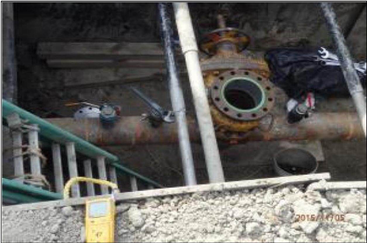
Figure 4: PCF Installation to Complete Abandonment
