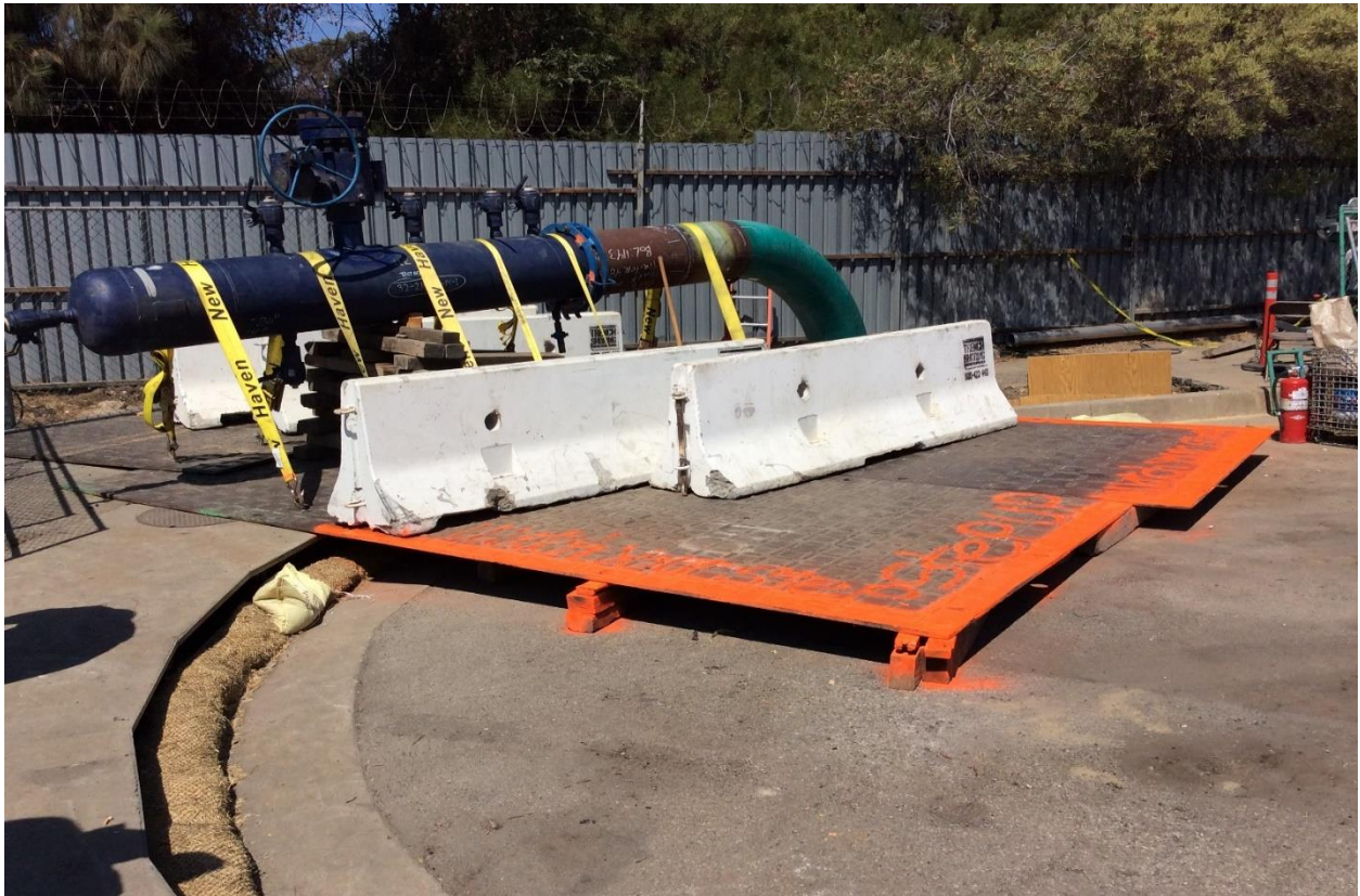
Figure 5: Installed Test Head Configuration
