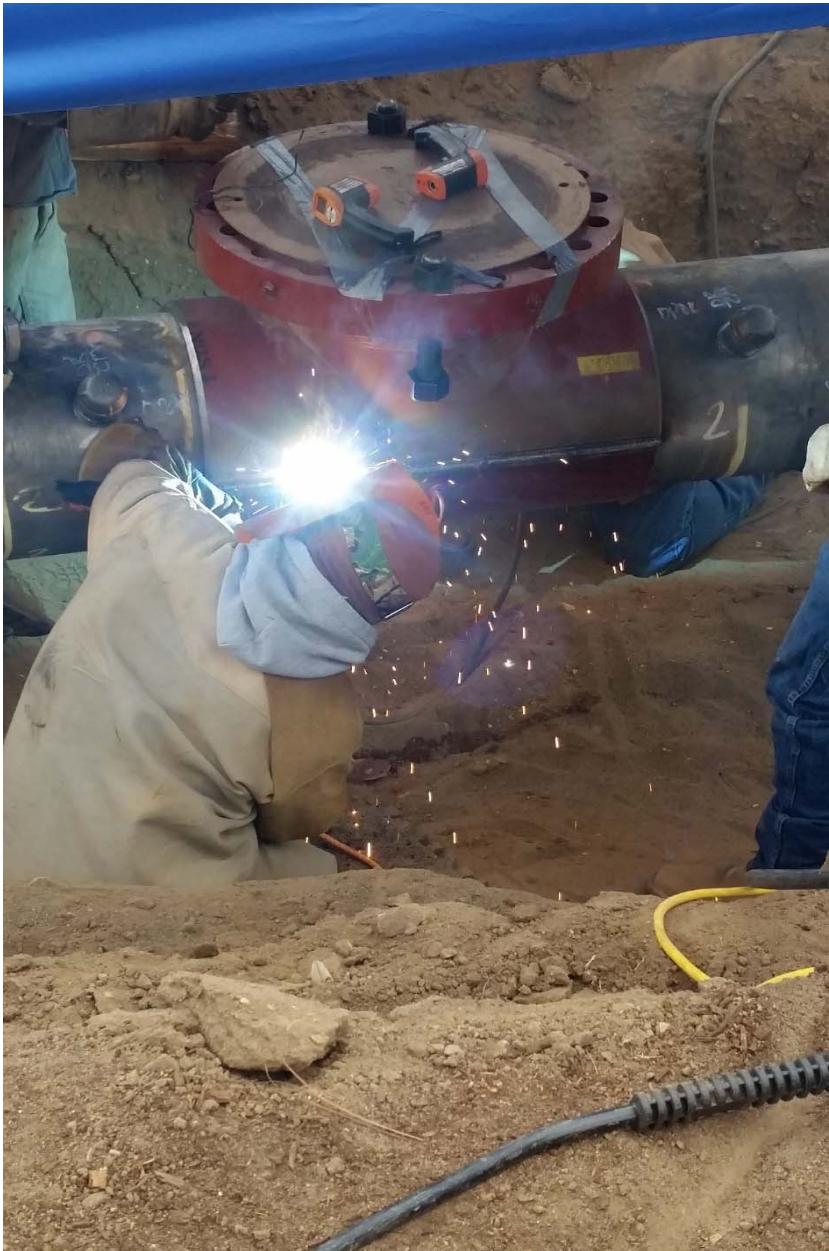
Figure 6: Welding of Stopple Fitting at Battles Road
