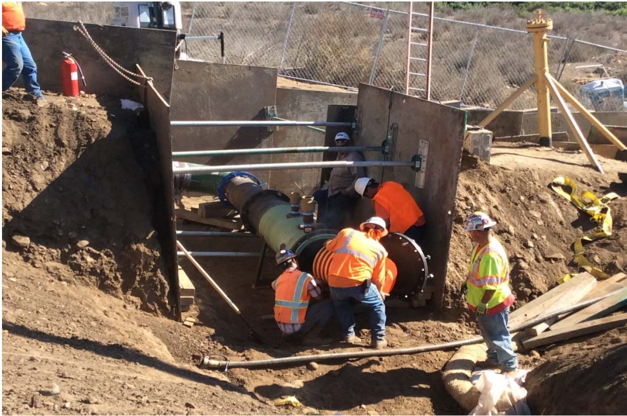
Figure 18: Section 2 Hydrotest Prep at Hall Canyon Site
