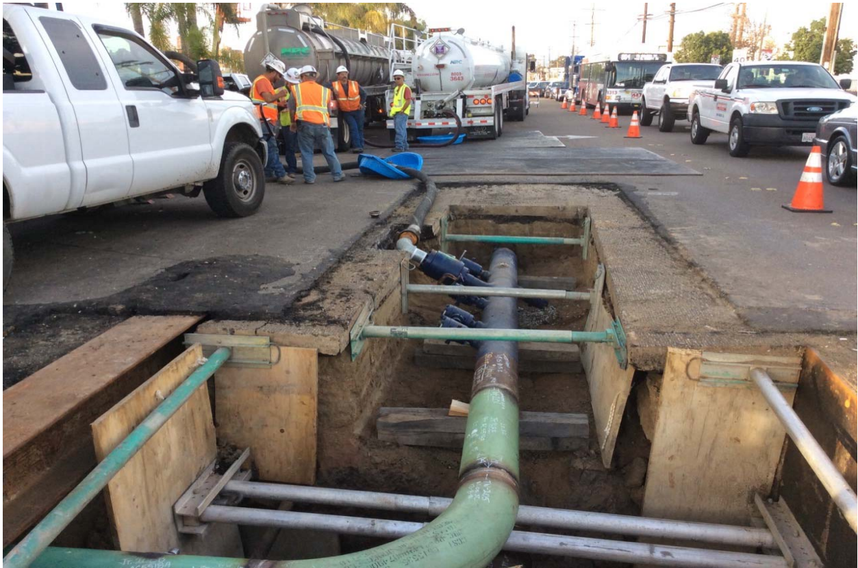
Figure 11: Hydrotest Contractor Setting Fill Pipe
