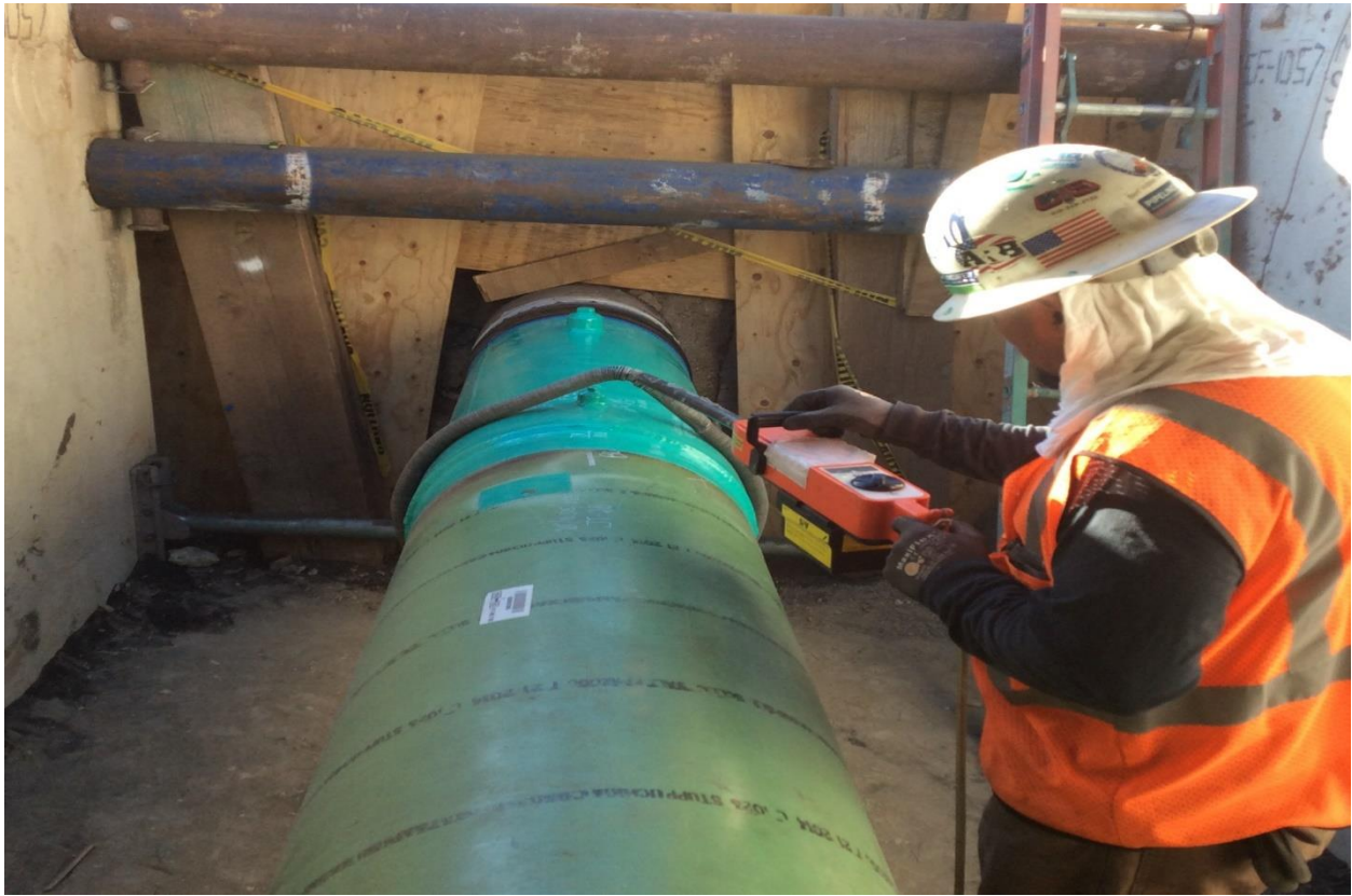
Figure 9: Coating Check Prior to Backfill
