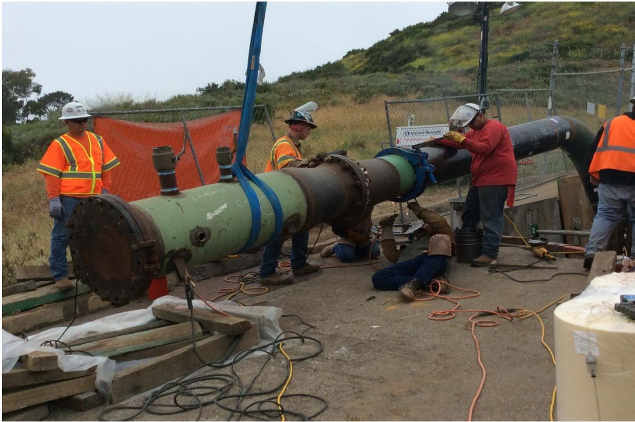
Figure 20: Section 2A Test Head Installation at Hall Canyon Site
