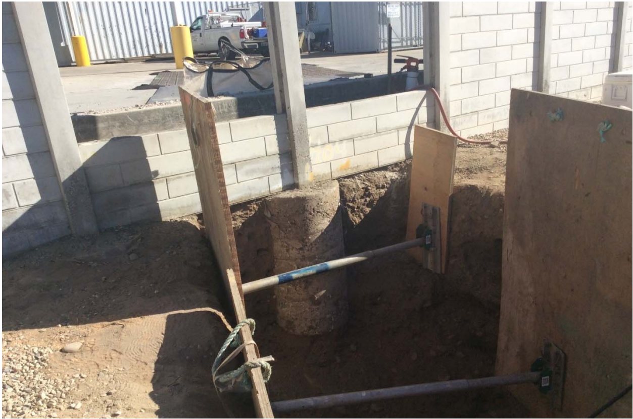
Figure 16: Section 1 Existing Wall Footing Within Trench
