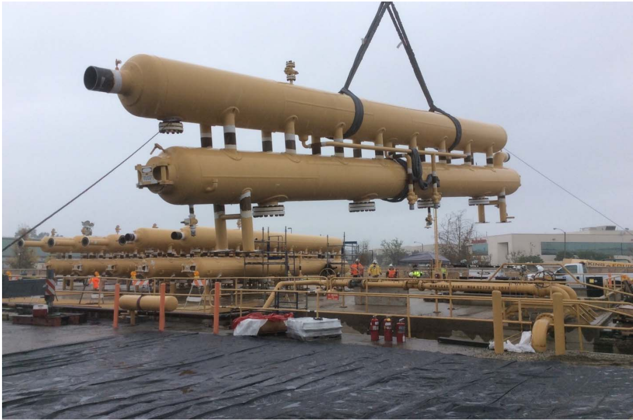
Figure 5: One (of Seven) Scrubber Assemblies Being Removed
