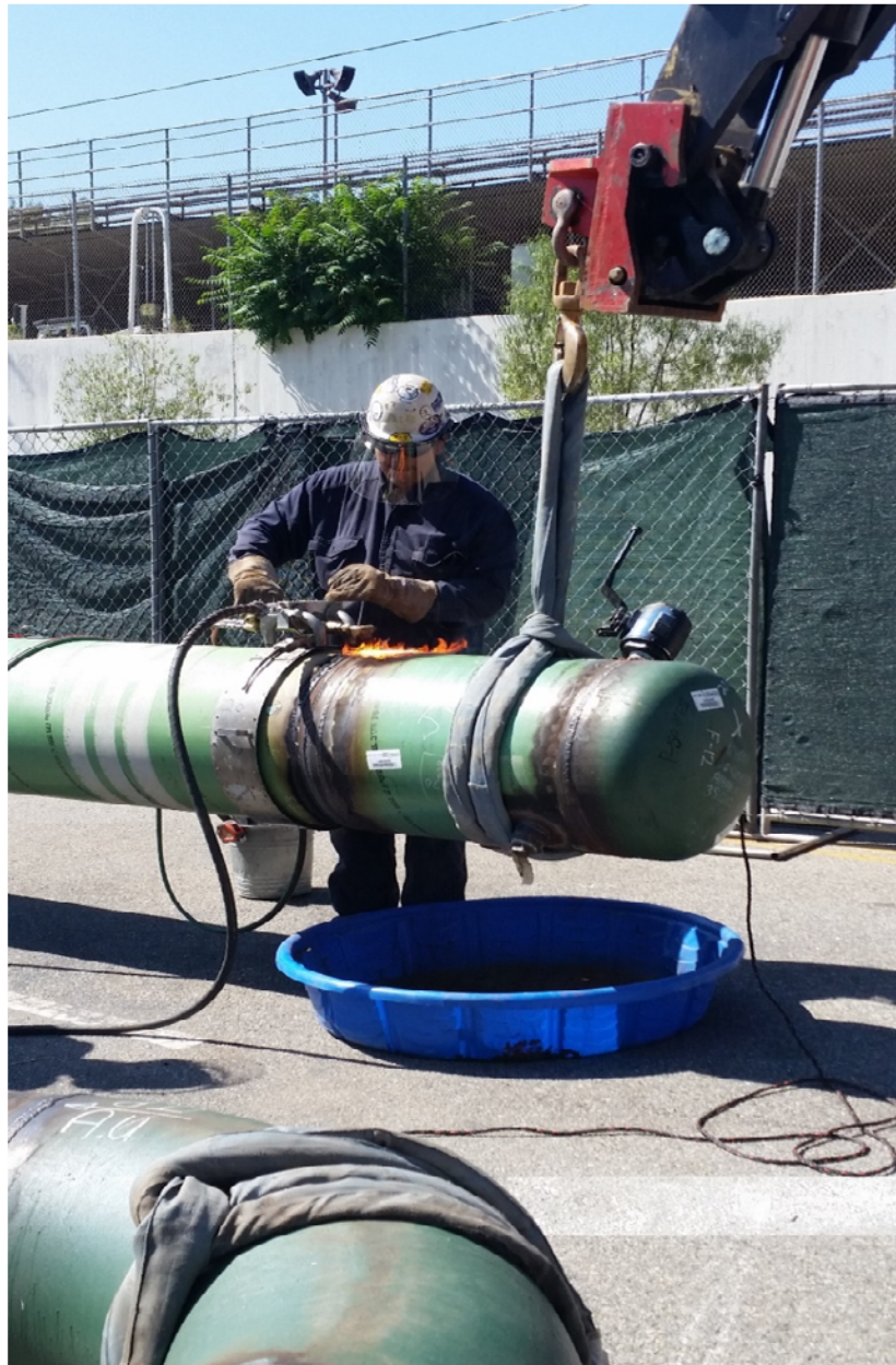
Figure 26: Section 9 Preparation of Isolation Caps
