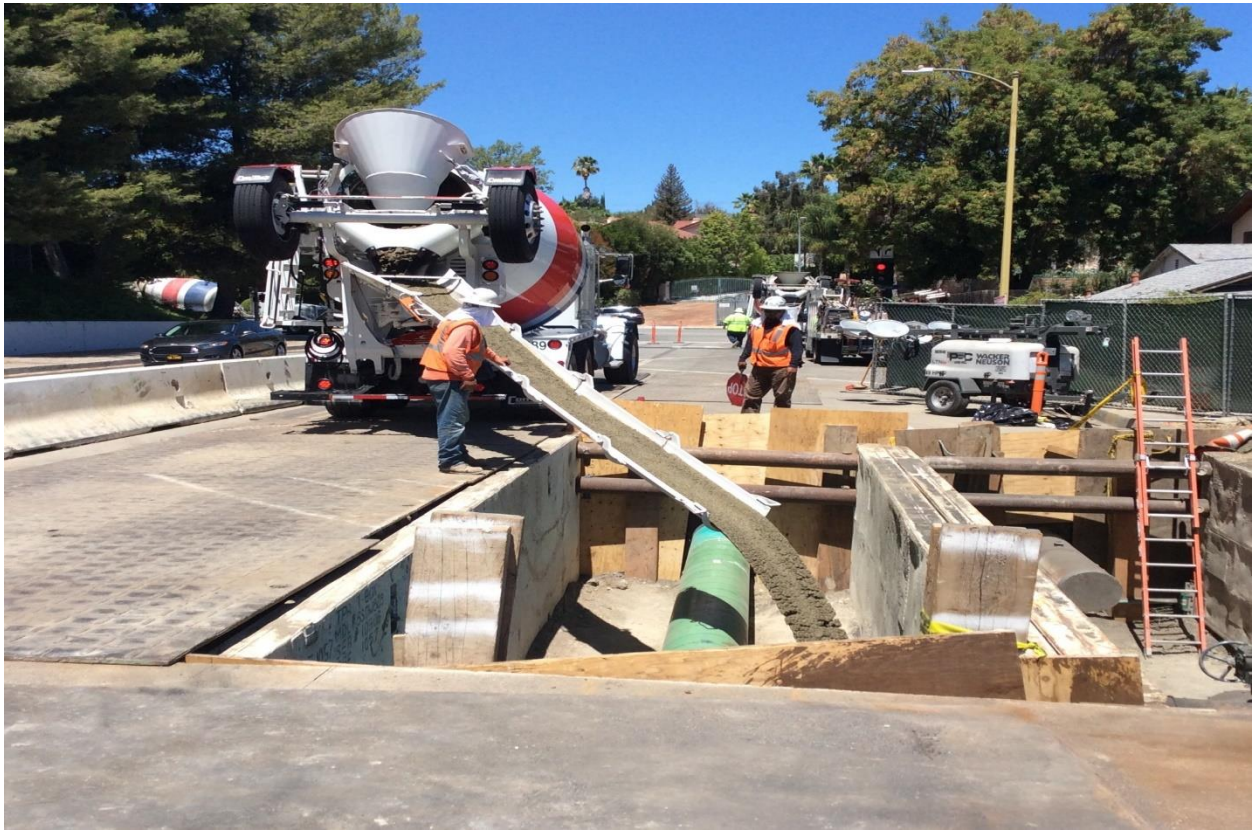
Figure 10: Backfilling Bell Hole Line 406 at Burbank Boulevard
