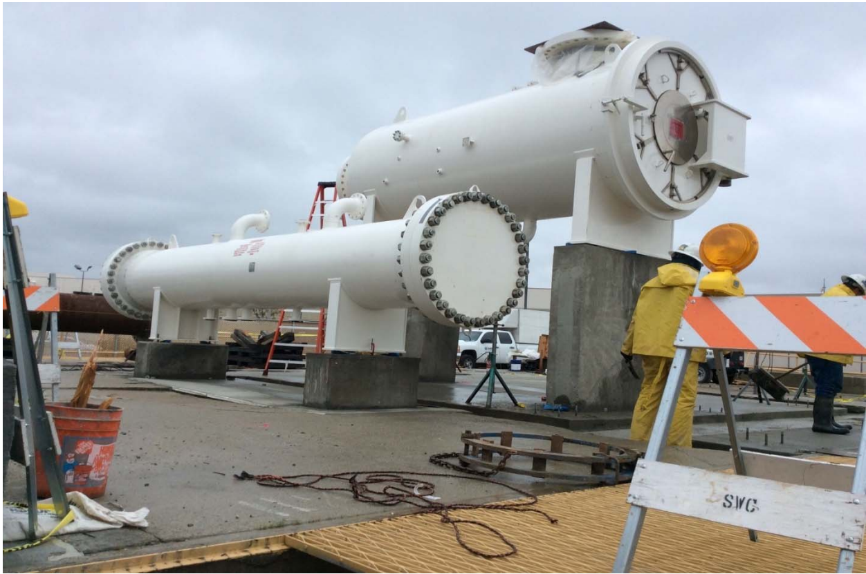
Figure 8: New Filter Separator Vessels
