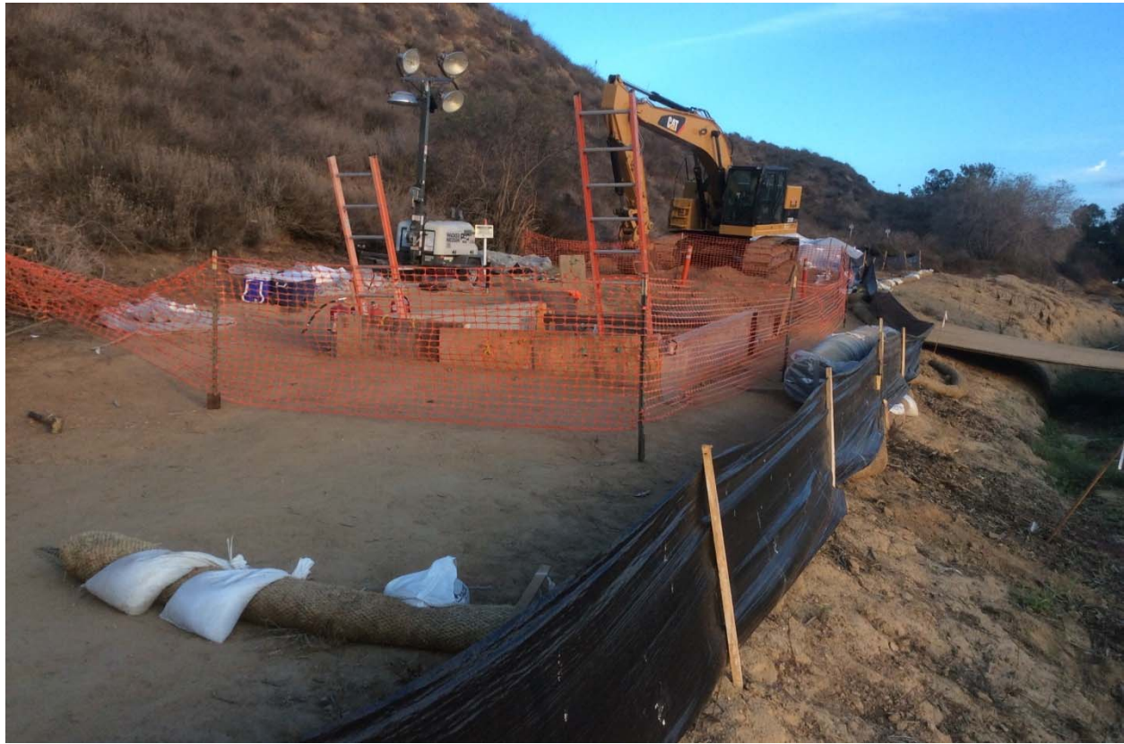
Figure 24: Section 4 and 5 West End Test Head Excavation
