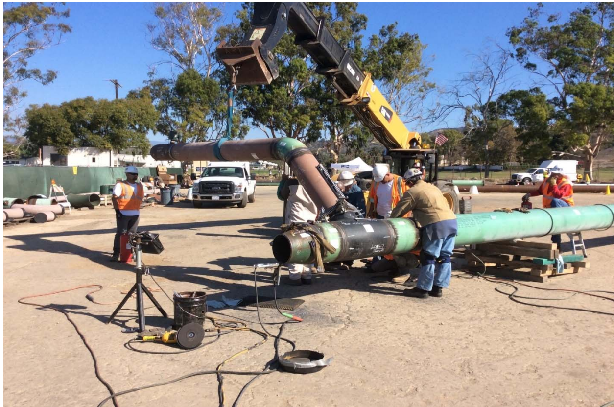
Figure 15: Section 1 Pre-fabrication of Replacement Pipe
