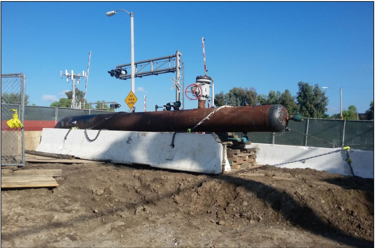
Figure 5: South End Test Head
