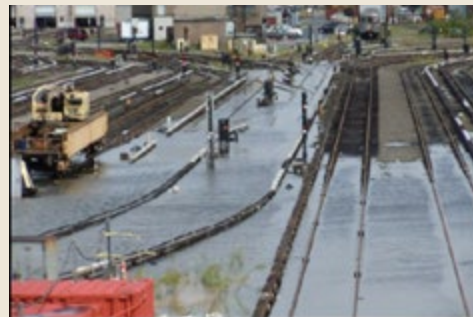
Figure 16.6. Flooded subway tracks in Coney Island after Hurricane Irene. (Photo credit: Metropolitan Transportation Authority of the State of New York 2011).
