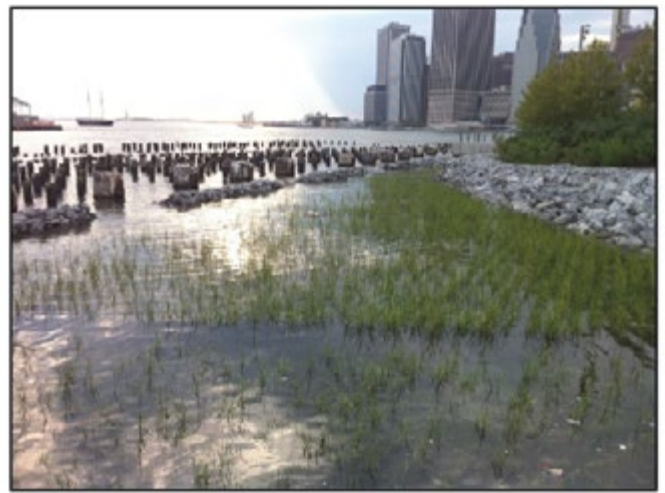
Figure 25.6. A coastal ecosystem restoration project in New York City integrates revegetation (a form of green infrastructure) with bulkheads and riprap (gray or built infrastructure). Investments in coastal ecosystem conservation and restoration can protect coastal waterfronts and infrastructure, while providing additional benefits, such as habitat for commercial and recreational fish, birds, and other animal and plant species, that are not offered by built infrastructure. (Photo credit: Department of City Planning, New York City, reprinted with permission).
