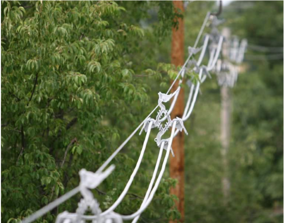
Figure 3. An example of spacer cable CC construction. Photo from Hendrix Aerial Cable Systems [Trager].
