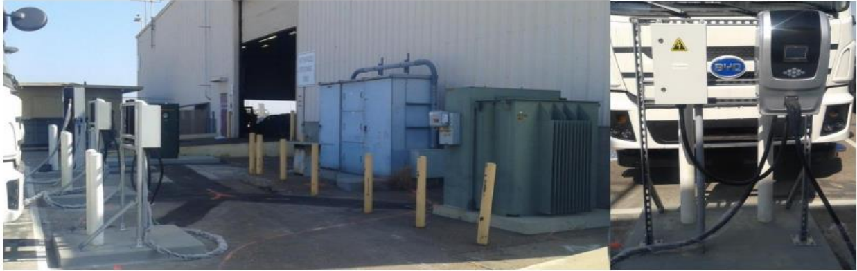
Figure 4. Equipment Installation at Pasha
