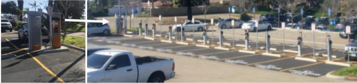
Figure 15. Electrify Local Highways Equipment Installation
