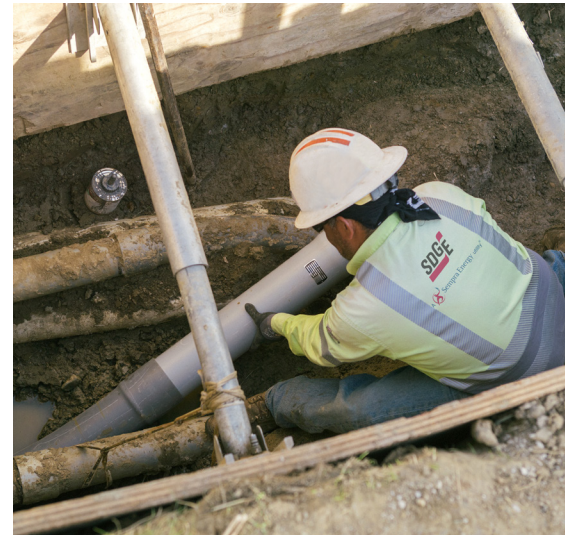
Julian undergrounding project
