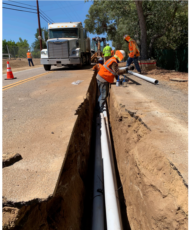
Valley Center undergrounding project
