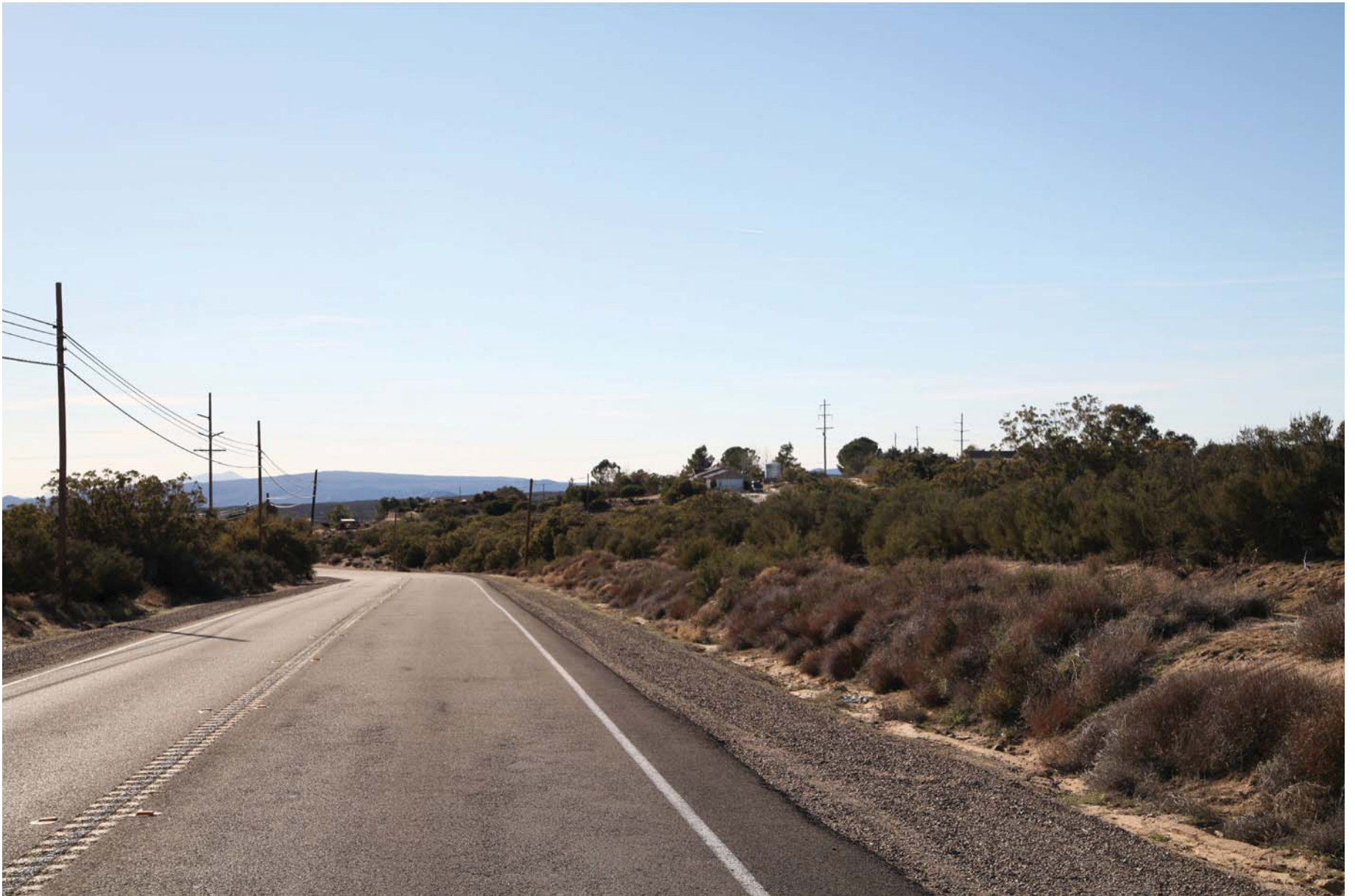
Existing View from SR-94 looking west (VP 4)
