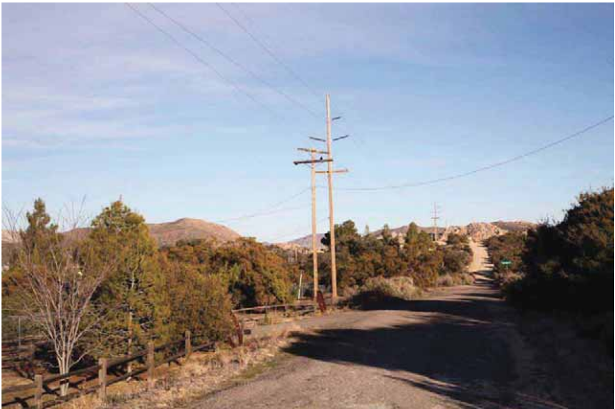
8. Ross Avenue at McCain Lane looking east
