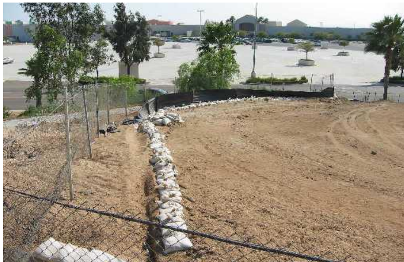
Gravel bags used as perimeter control.
