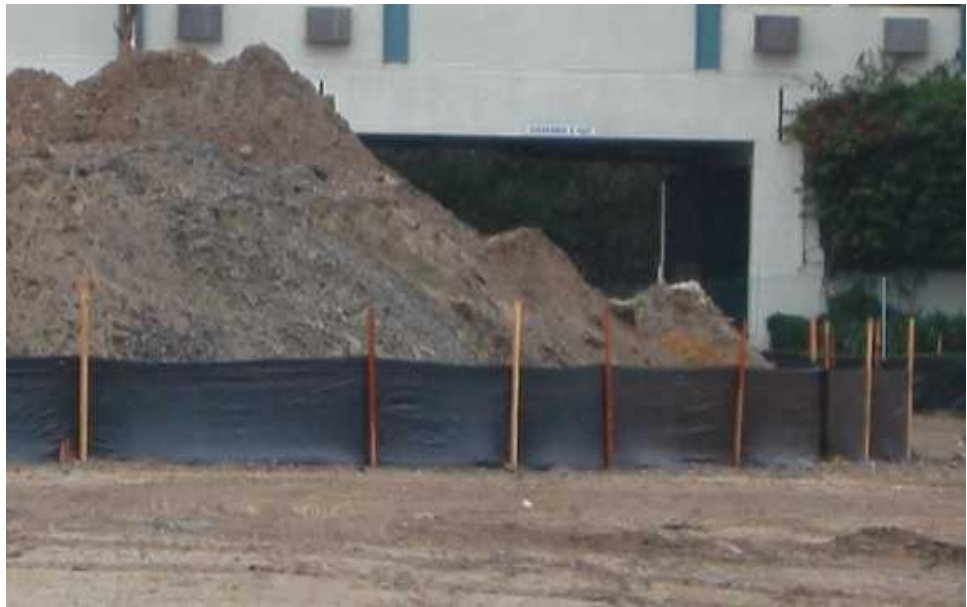
Silt fence used for stockpile perimeter control.
