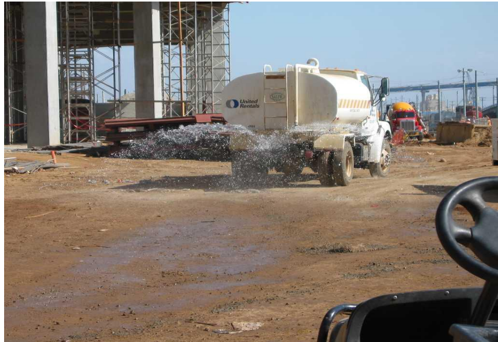
Water being applied for dust control.
