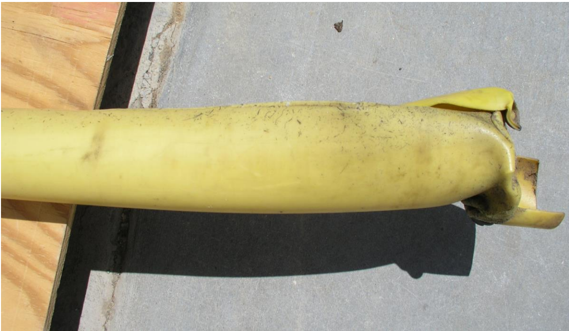
Figure 5. Close-ups of distortion and melting from fire in west guard (top) and east guard (bottom)
