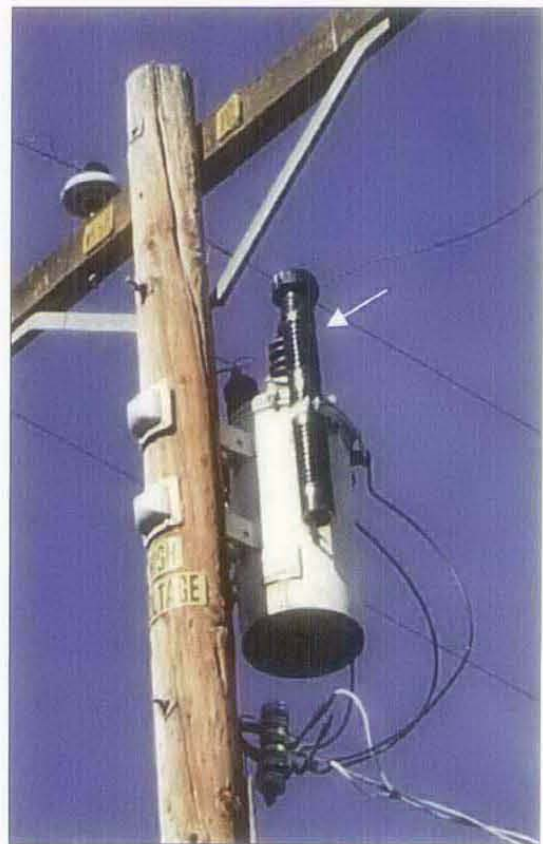
Figure 2-25 Lightning Arrester
