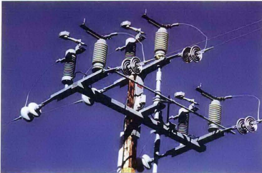
Figure 3-20 S&C Omni-Ruptor Switch, Triangular Construction (open position)
