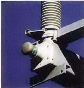
Open Position Indicator Green Letter "O" visible
