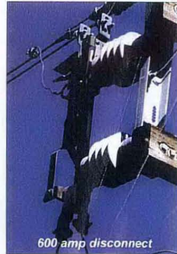
Figure 2-10 Solid Blade Disconnects
