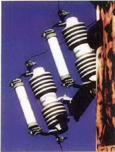
Figure 3-1 Arm Mounted Cutout with Non-Expulsion Fuse
