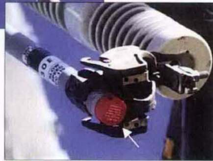
Figure 3-9 SMU-20 Fuse - Detail
