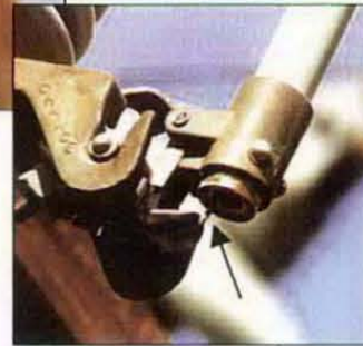
Figure 2-2 Universal Fuse, Fuse link, Expulsion end of fuse
