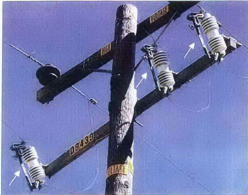
Figure 2-9 Arm Mounted Cutout with Solid Blade Disconnect (open position)
