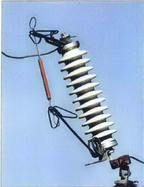
Figure 2-5 Bushing Mounted Cutout with Open Link Fuses
