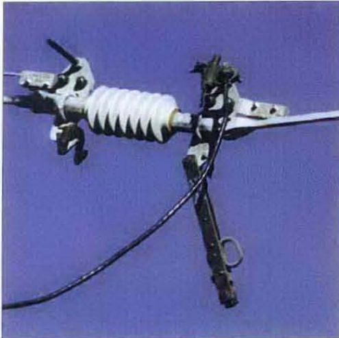
Figure 2-14 In-Line Disconnect (open position)
