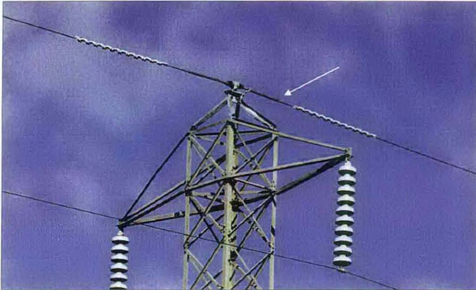
Figure 4-27 Tangent Transmission Tower with Static Line
