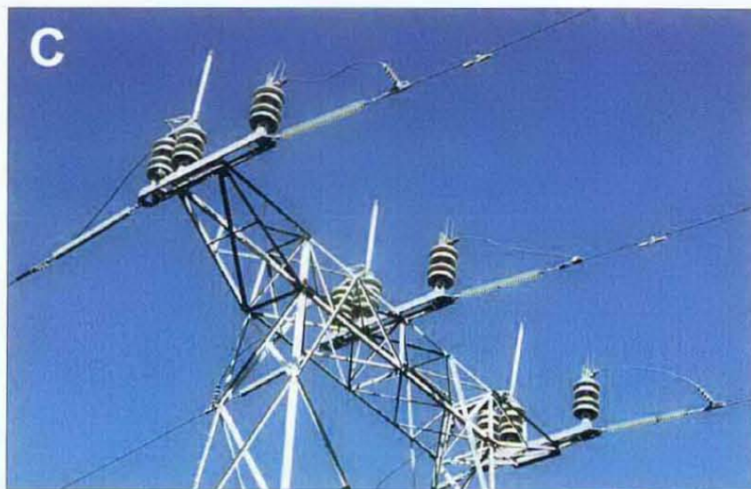
Figure 2-34 Transmission Air Switches A. Tower Mounted (closed position) B. Pole Mounted (closed position) C. Tower Mounted (open position)
