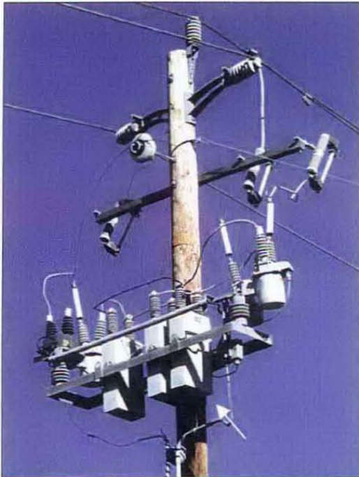
Figure 3-29 Capacitor Bank
