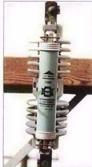
Figure 3-2 Arm Mounted Cutout with Non-Expulsion Fuse
