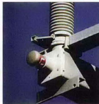
Closed Position Indicator Red Letter "C" visible
