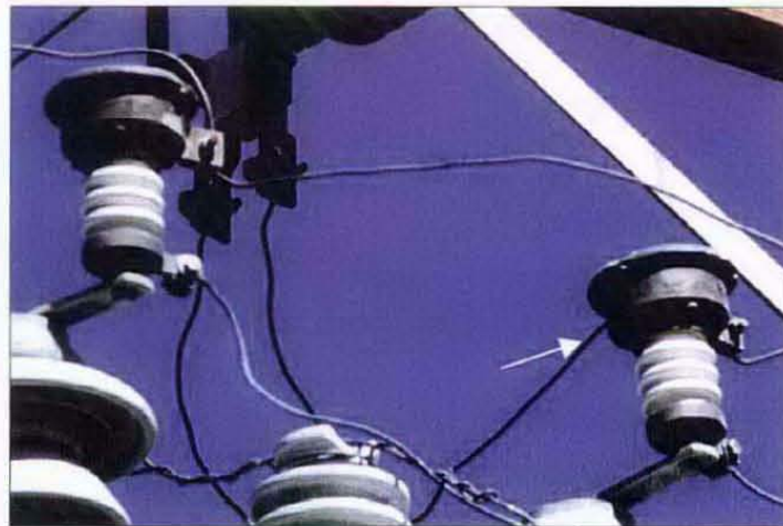
Figure 2-19 Lightning Arrester
