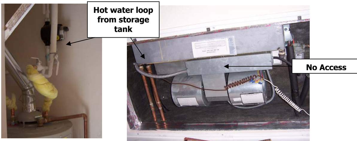
Figure 65: Hydronic Fan Coil Unit
