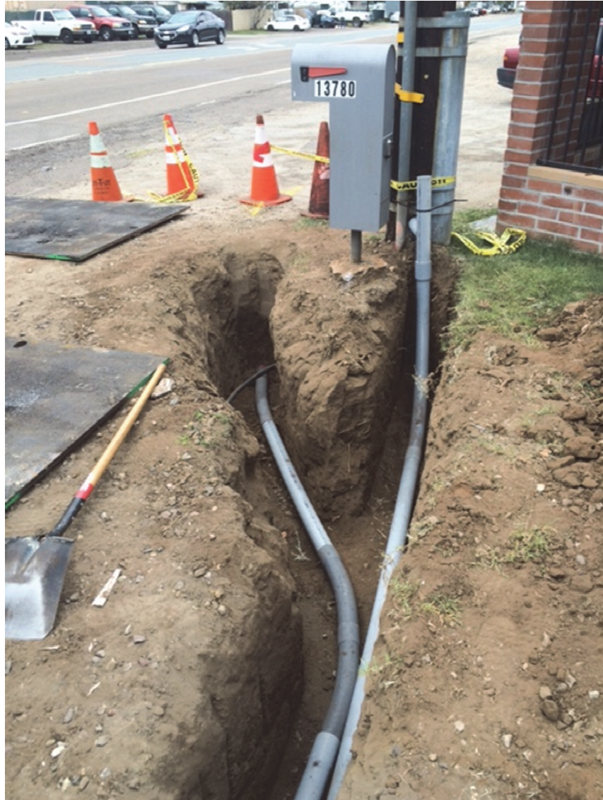
Fig. 3: Laying conduit in the trench
