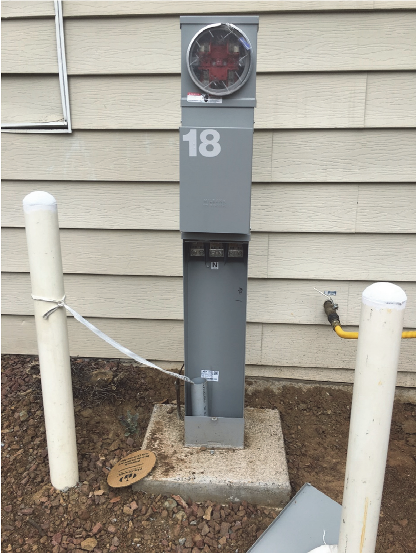
Figure 8: Pulling cable up to the electric pedestal
