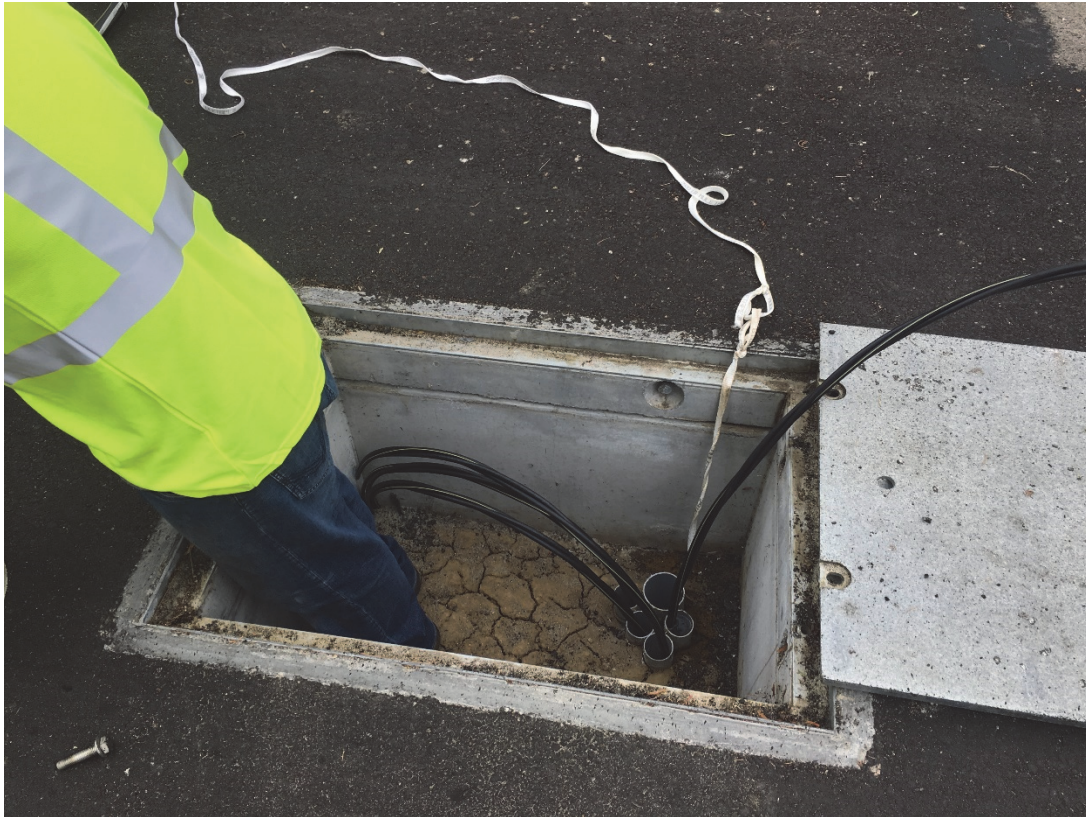
Fig. 7: Pulling cable after civil construction
