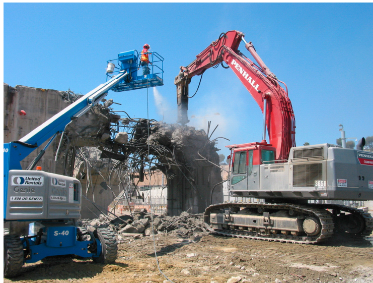
Figure III-4 Demolition of Turbine Building
