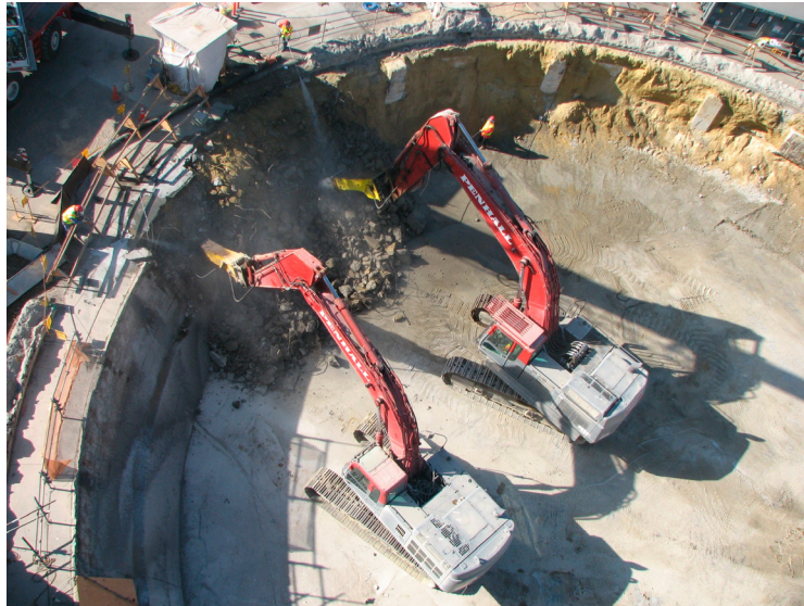
Figure III-17 Demolition of Containment Cradle and Sphere Enclosure Building Foundations above Elevation 8' 6"
