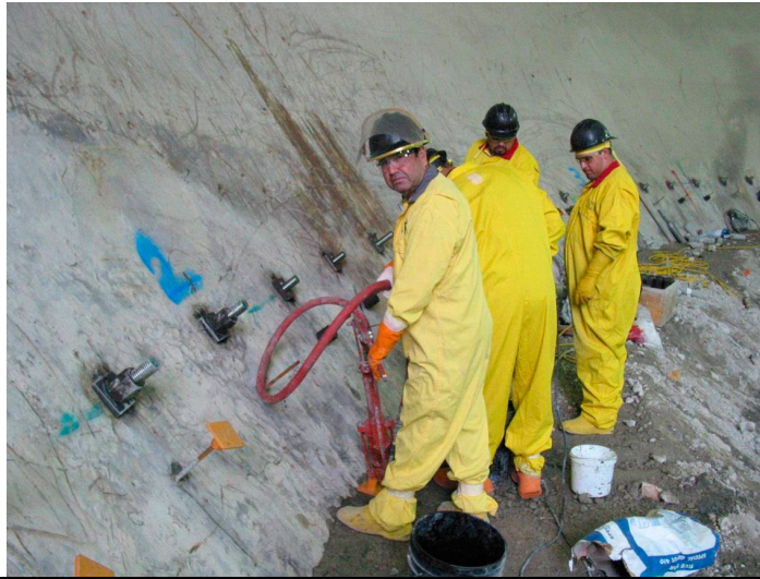
Figure III-8 Anchoring SONGS 1 Containment Sphere to Concrete Foundation
