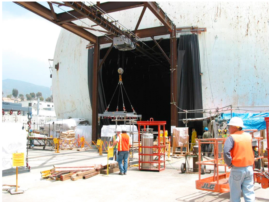
Figure III-7 Removing Debris from Inside SONGS 1 Containment Sphere
