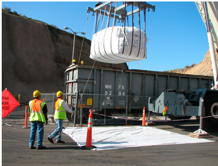
Figure III-22 Placing Lift Liner Containing Concrete Rubble into Gondola Rail Car
