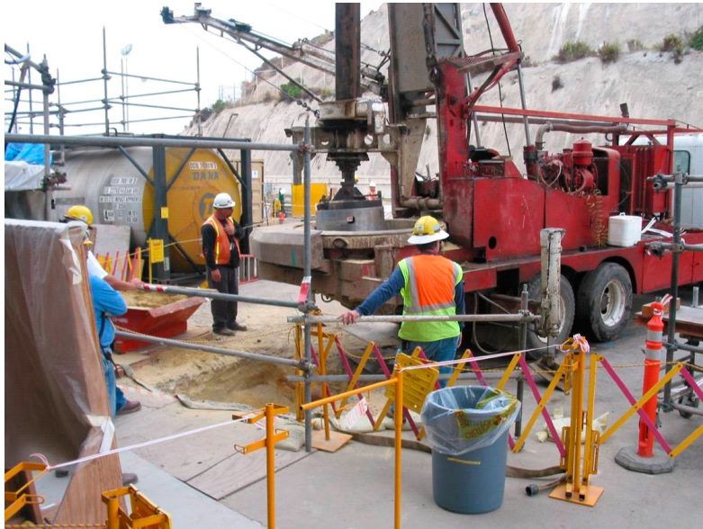
Figure III-10 Installation of Dewatering Well Prior to Containment Demolition
