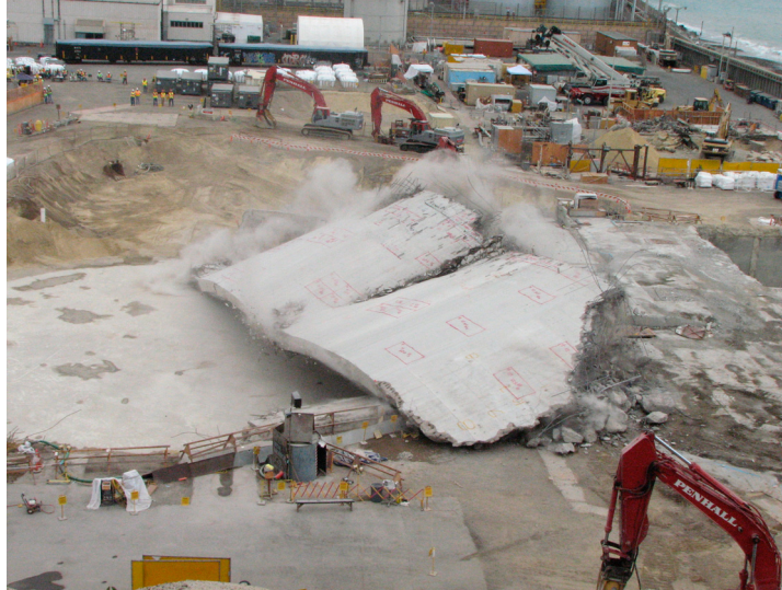
Figure III-17 Demolition of Containment Cradle and Sphere Enclosure Building Foundations above Elevation 8' 6"
