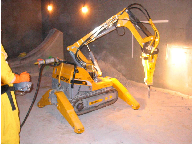
Figure III-20 Cleanup of Contaminated Debris from Lower Radwaste Building
