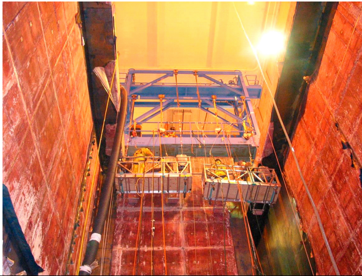
Figure III-26 Removal of Spent Fuel Pool Stainless Steel Liner
