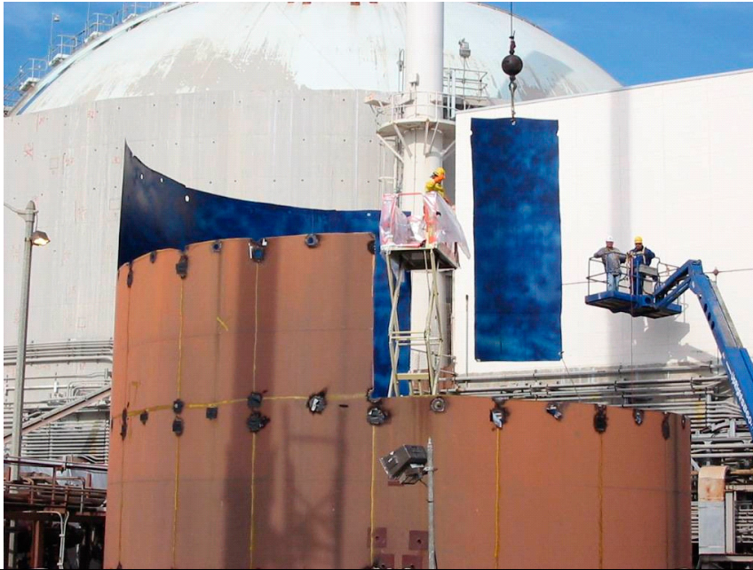
Figure III-24 Demolition of Refueling Water Storage Tank
