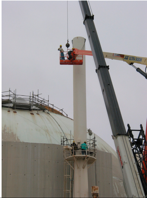
Figure III-26 Removal of Spent Fuel Pool Stainless Steel Liner
