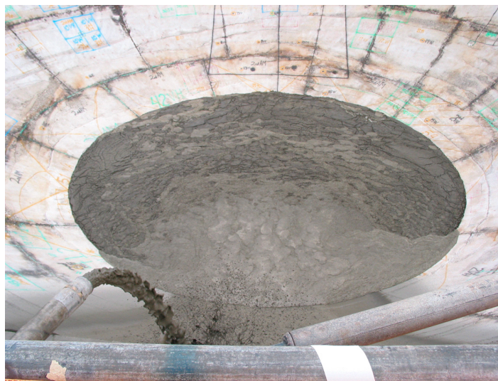
Figure III-14 Filling SONGS 1 Containment Concrete Foundation with Low Density Grout
