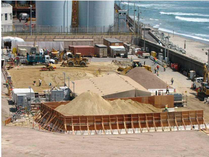
Figure III-33 Excavation and Removal of Improvements in SONGS 1 Southwest Quadrant
