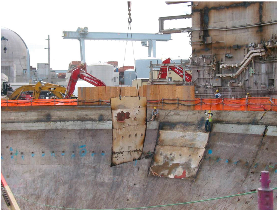
Figure III-12 Removal of Torch Cut Piece of SONGS 1 Containment Sphere
