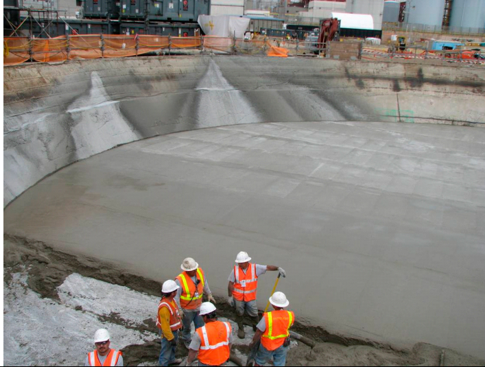
Figure III-15 Installing Concrete Cap over Grout in SONGS 1 Containment Foundation
