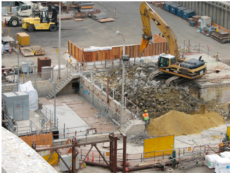
Figure III-23 Demolition of Intake Structure Above Elevation 8'6"
