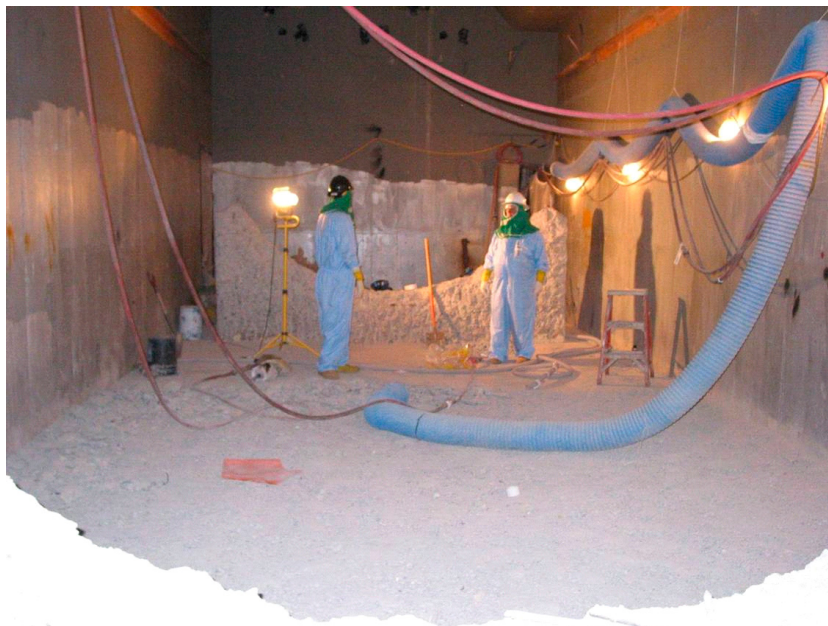
Figure III-20 Cleanup of Contaminated Debris from Lower Radwaste Building
