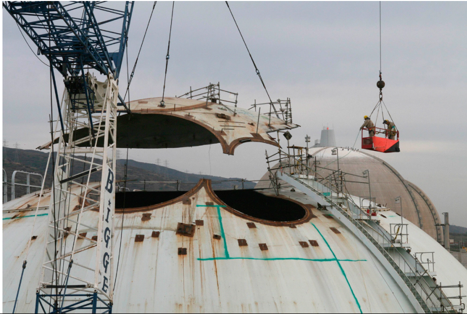
Figure III-12 Removal of Torch Cut Piece of SONGS 1 Containment Sphere
