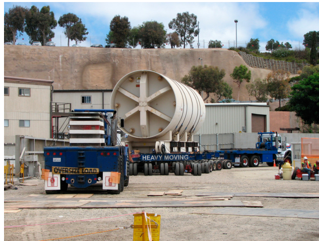
Figure III-39 SONGS 1 Reactor Pressure Vessel Package on Interim Storage Pad
