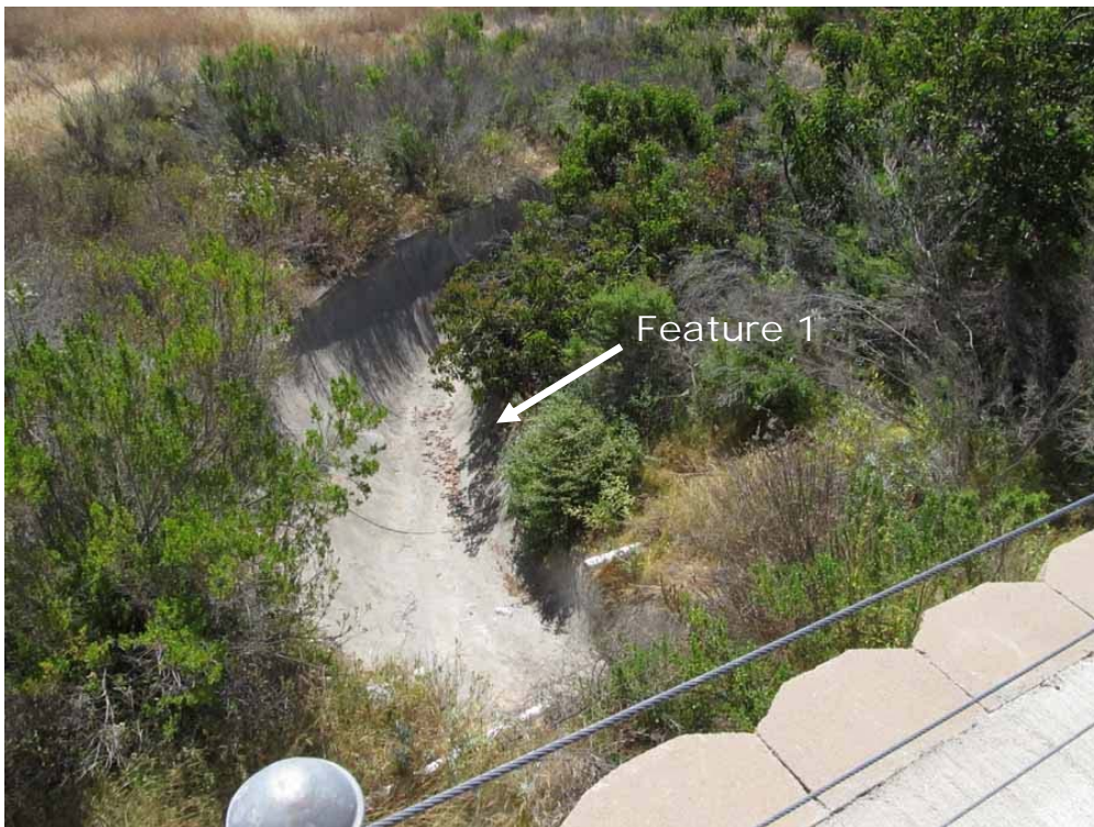
Photograph 2 (East of Talega Substation, Mapbook Pages 2 and 3): Feature 1, concrete channel east of Talega Substation. View east.
