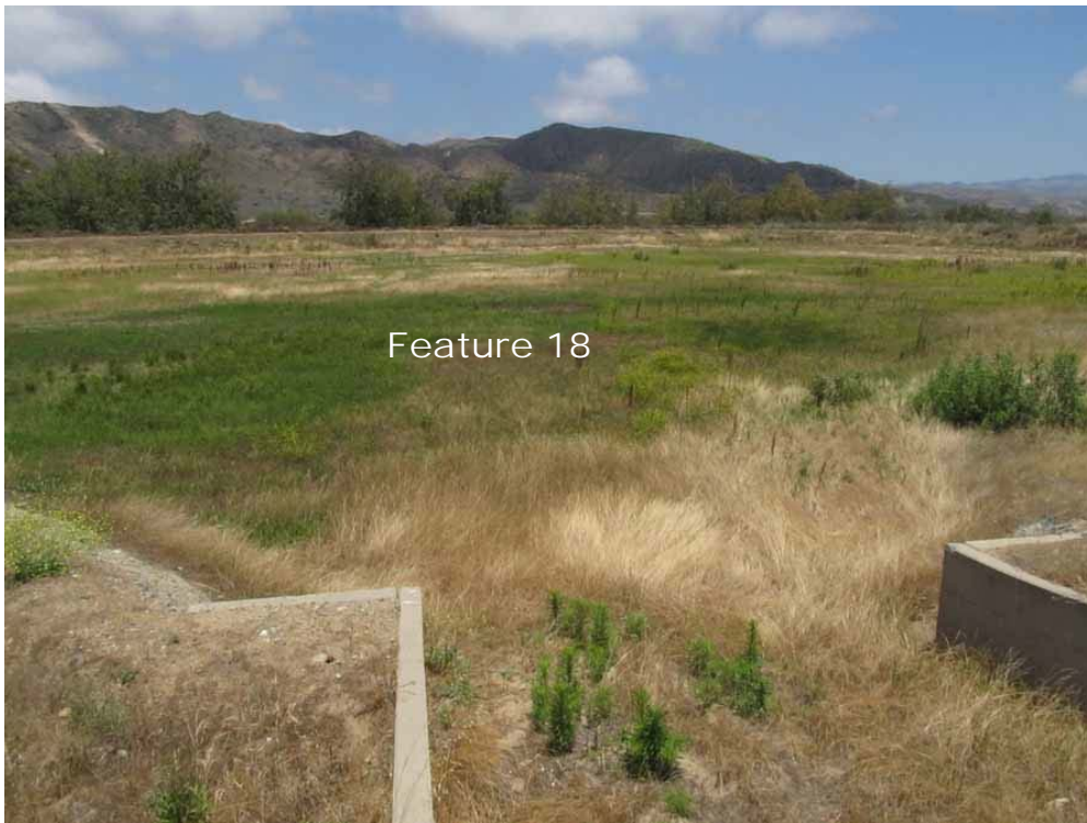
Photograph 36 (Between Poles 65 and 67, Mapbook Page 35): Feature 18, overflow basin. View east.
