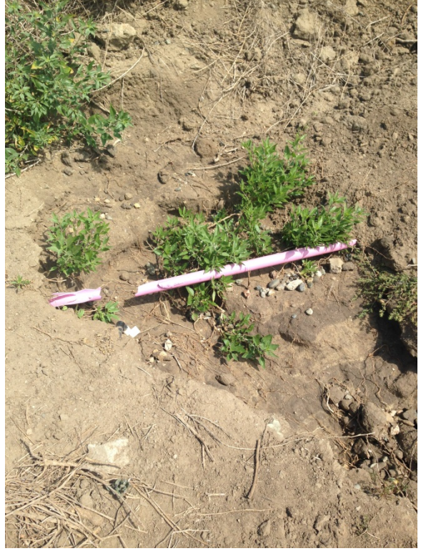
Burst irrigation pipe upslope and northwest of Basin 21-1. Photo by RCS, 9 Sep 2015.
