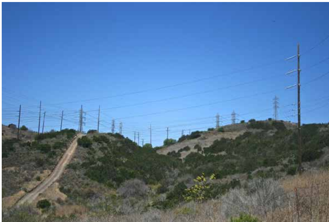
Viewpoint 8: Existing view looking southwest from SDG&E access road at power line.
