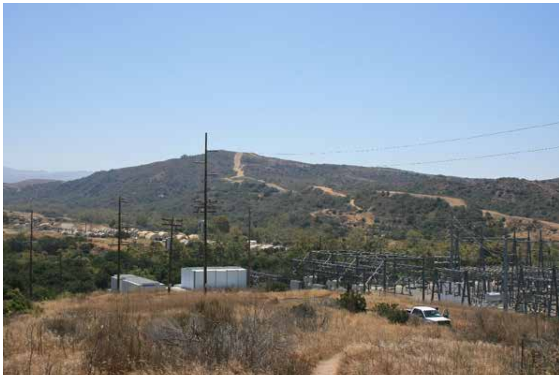
Viewpoint 7: Existing view looking southeast from SDG&E access road at Talega Substation.
