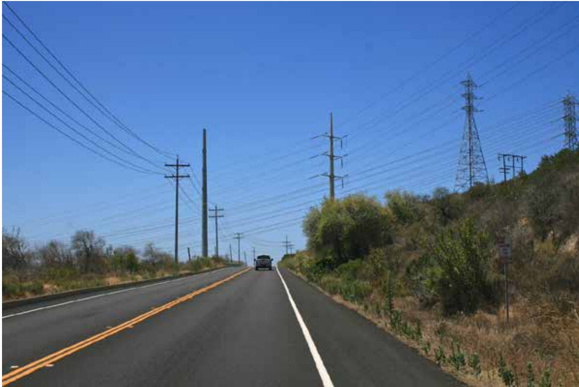
Viewpoint 15: Existing view looking southwest from Cristianitos Road, south of bend in large wash.
