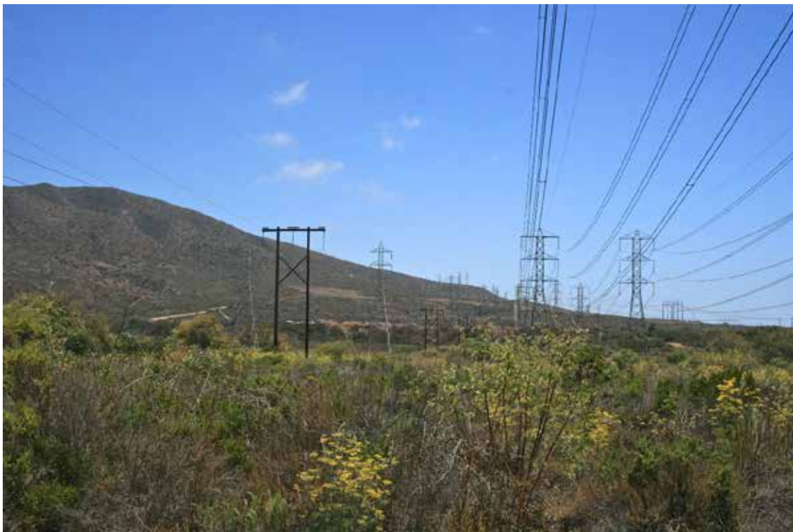
Viewpoint 24: Existing view looking southeast from the edge of Basilone Road at existing lattice tower structure. (A simulation of Viewpoint 24 is included in Appendix 4.1-B: Visual Simulations.)
