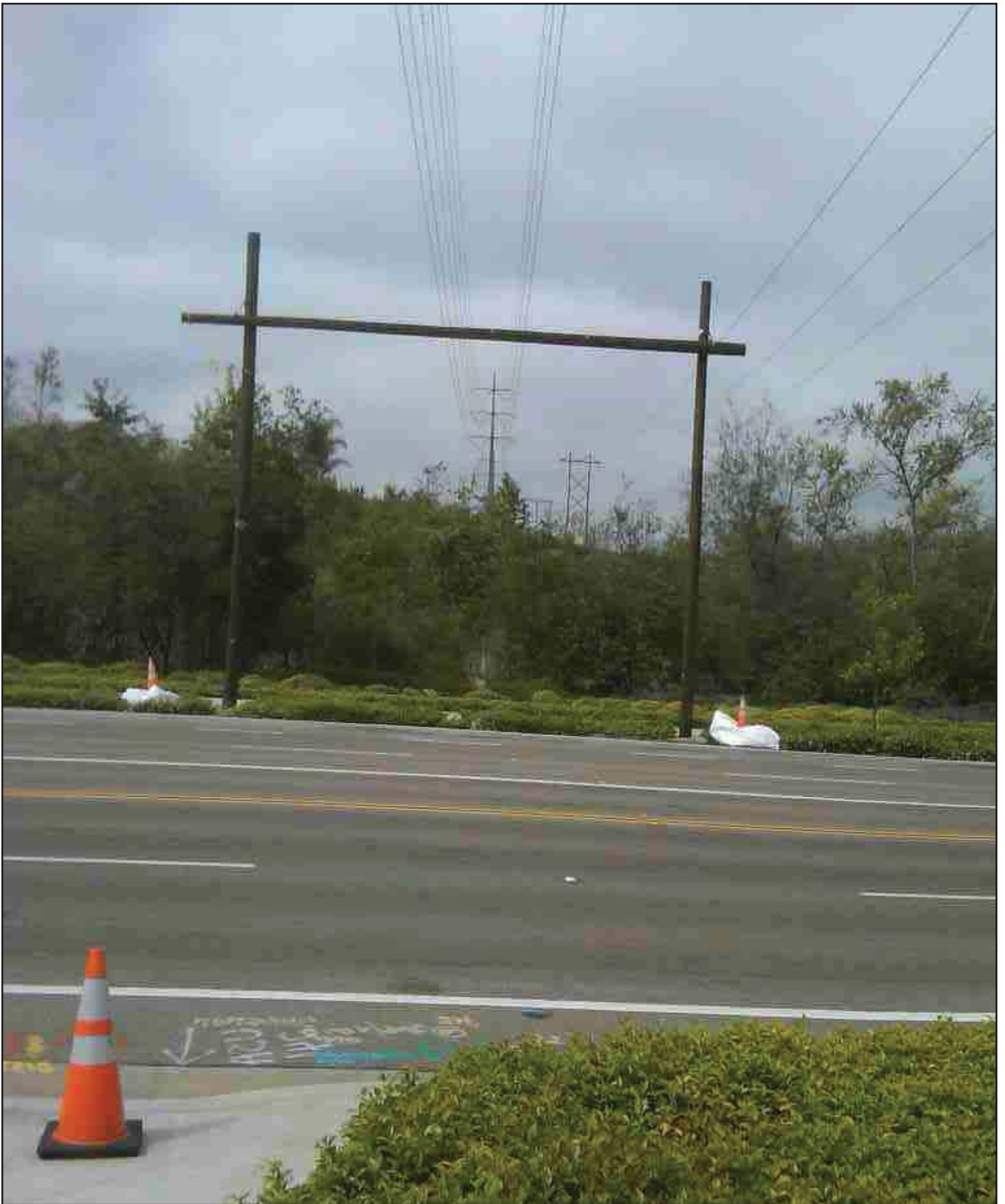
Figure 3C-17 Typical Guard Structure - 1
