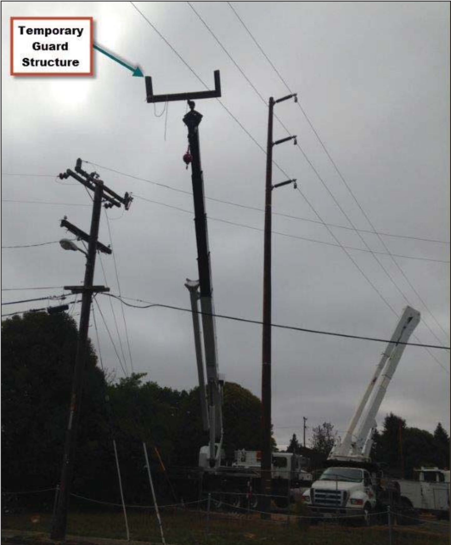
Figure 3C-18 Typical Guard Structure - 2
