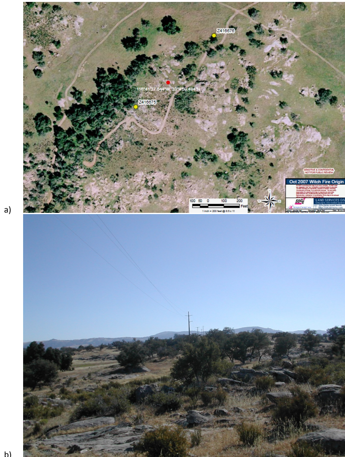
Appendix 4. a) Witch fire site plan view produced by SDGE; red dot is fire ignition location; yellow dots are pole locations. b) photo taken by Peterka at Witch site looking northeast along the power line. Note the foliage height is significantly below line height, and the density of trees is scattered.
