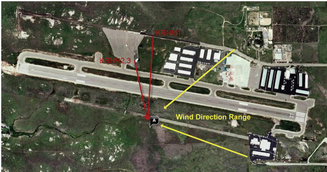
Exhibit 12b. Ramona Airport ASOS station and location of photographs KRNM1 and KRNM3; "A" is the anemometer site.
