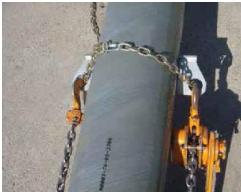
FIGURE 11 JACKING LUG SAFETY STRAP/CHAIN INSTALLATION
