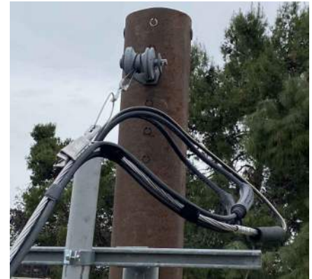
FIGURE 4 STORM SAFE FLEXIBLE BAIL ASSEMBLY
