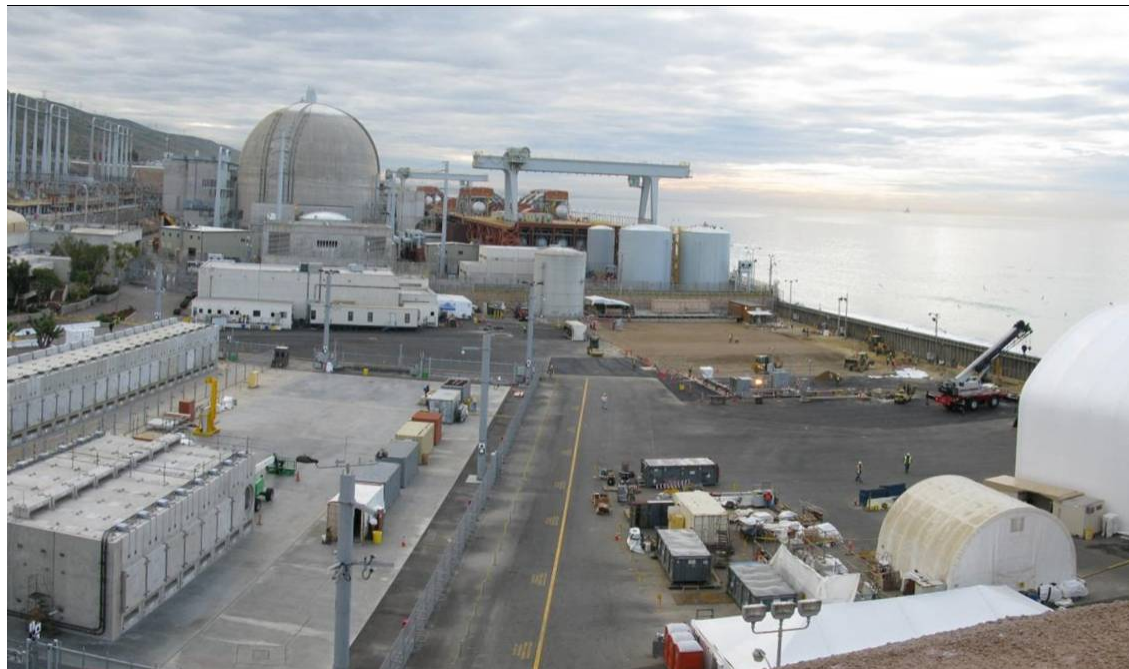
Figure II-2 SONGS 1 Decommissioning Site in December 2012
