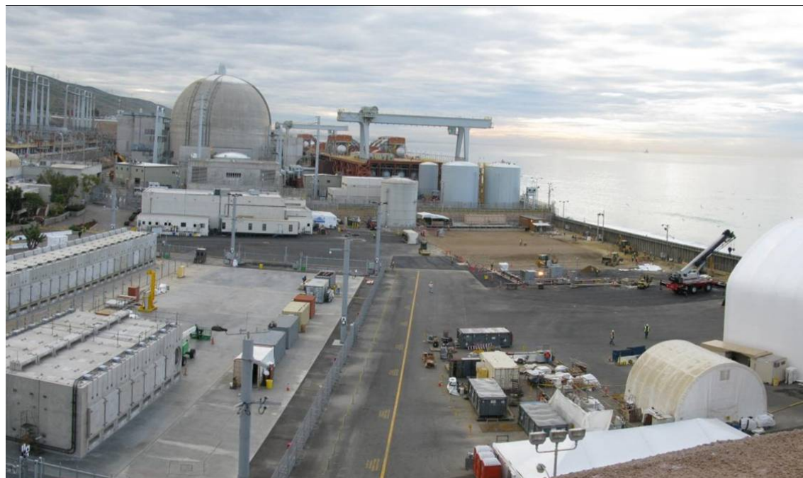
Figure II-1 SONGS 1 Decommissioning Site in December 2008
