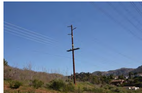
Sample steel pole with reflective tape and climbing pegs.
