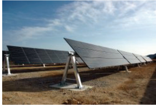
Wattsun HZ-Series Linear Axis Tracker in South Korea. These trackers use a horizontal axis.
