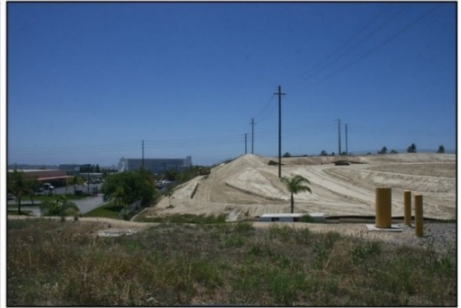
Northwest corner of Project Site, looking Northwest
