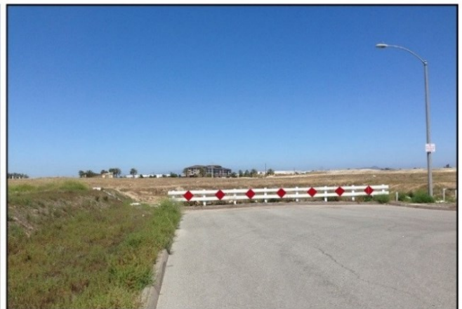
Senior Center Drive, looking East
