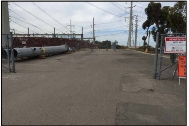
San Luis Rey staging yard at northwest corner, looking West
