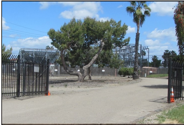
Melrose staging yard from Melrose Drive, looking Southwest
