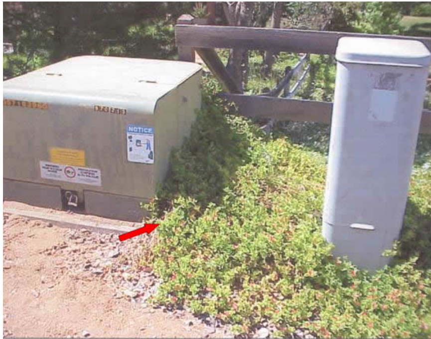
Weeds, Trees, Bushes, Dirt Or Obstacle Outside Unit (Clear On Site) Code 47
