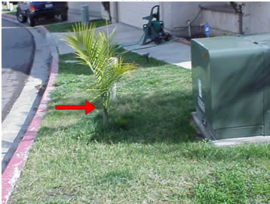
External Working Space Caused By Tree / Vegetation Code 330
