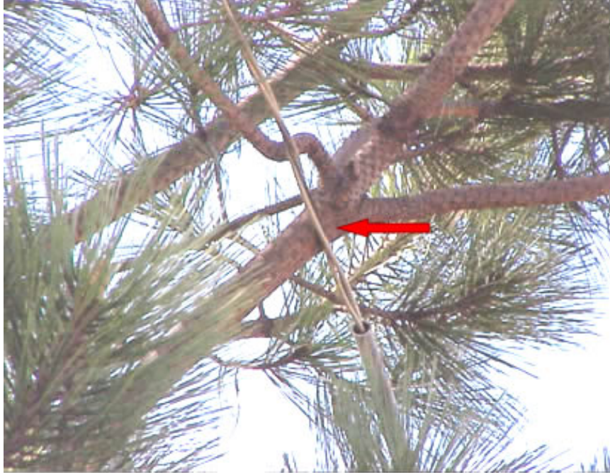
Need Tree Guard (Slipped Down) Code 323
