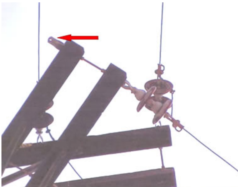
Idle Equipment – Code 239 This Condition No Longer an Infraction as Long as The Clevis is backing up Strain
