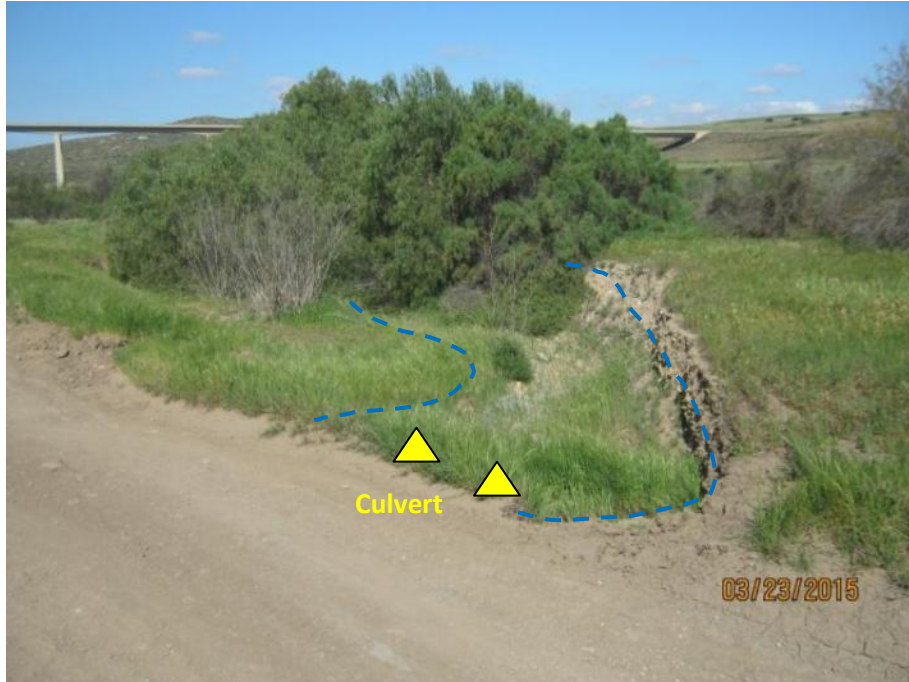
Photograph 21: Feature 21 is an un-vegetated ephemeral drainage located in between Location 57 and Location 58. Project activity includes vehicular access through the drainage as it crosses the road. Photograph taken facing north.
