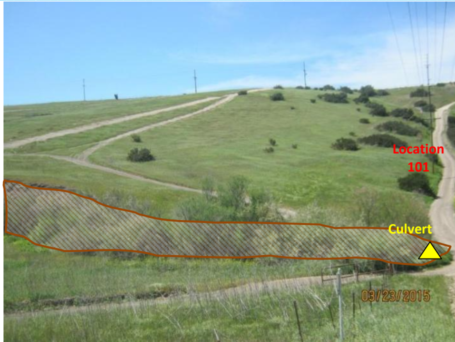
Photograph 31: Feature 31 is an ephemeral drainage with CDFW riparian scrub habitat located west of Location 100. Project activity includes vehicular access through the drainage as it crosses the road. Photograph taken facing southwest.
