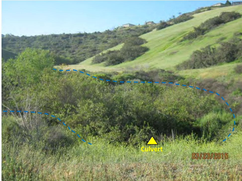
Photograph 5: Feature 5 is a vegetated drainage located southeast of location 14. As this feature is outside of proposed work areas, no impacts are anticipated. Photograph taken facing north.
