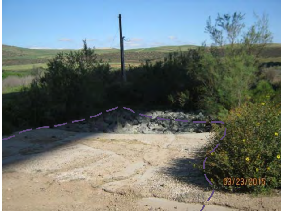
Photograph 17: Feature 17 is a non-jurisdictional concrete brow ditch and energy dissipater east of Locations 50.1 and 50.2. Feature 17 sheet flows across a maintained, concrete Arizona crossing on an existing project access road. Photograph taken facing north.
