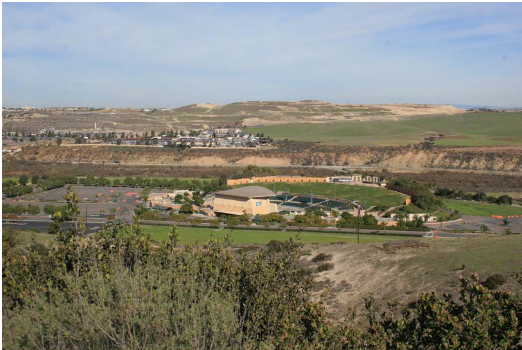
Viewpoint 7: Existing view looking north from the northwest corner of Vista Pacifica Community Park in a residential neighborhood near Dennery Canyon. (A simulation of Viewpoint 7 is included in Attachment 4.1-B: Visual Simulations.)
