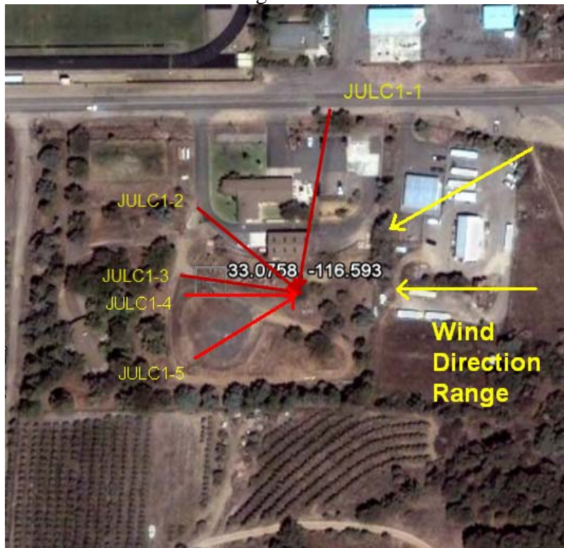
Appendix 13b. Julian anemometer location and location of photographs JULC1-1, JULC1-2, JULC1-3, JULC1-4, and JULC1-5 with wind direction range during the Santa Ana event; note sheltering trees and structures upwind of anemometer.
