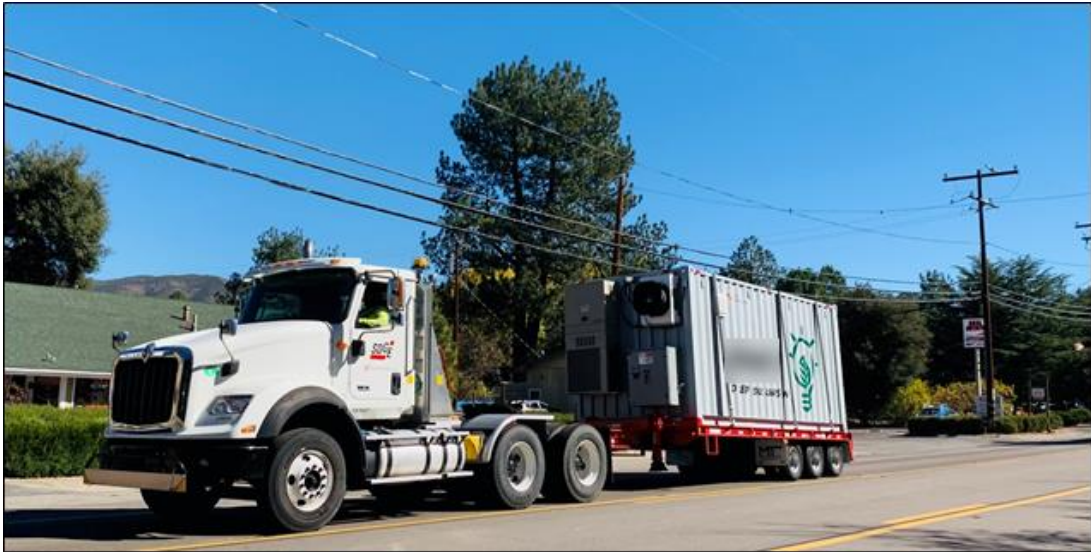
Figure 5-13. Photo of MBESS on the Road during Transportation from CRC 1 to CRC 2
