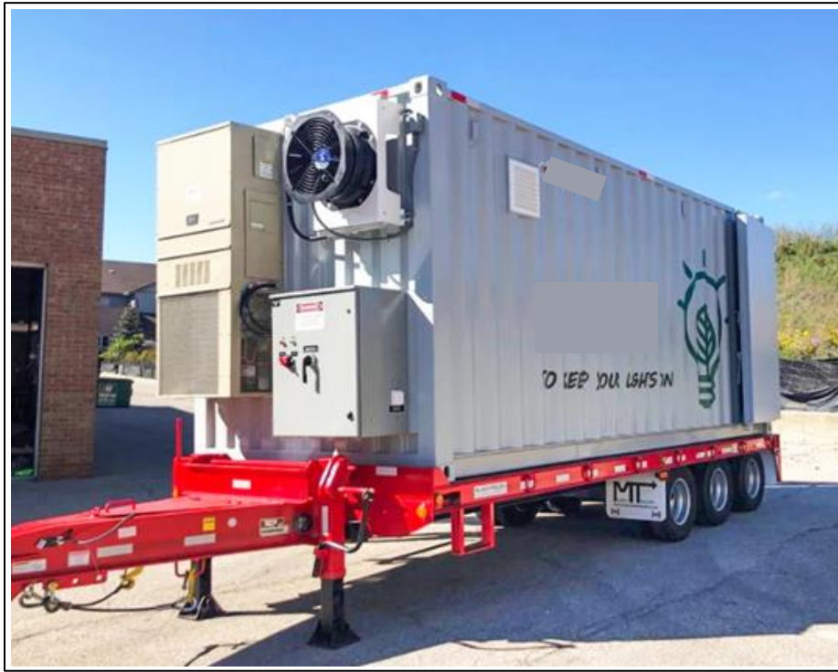
Figure 3-2. MBESS Container used in the project
