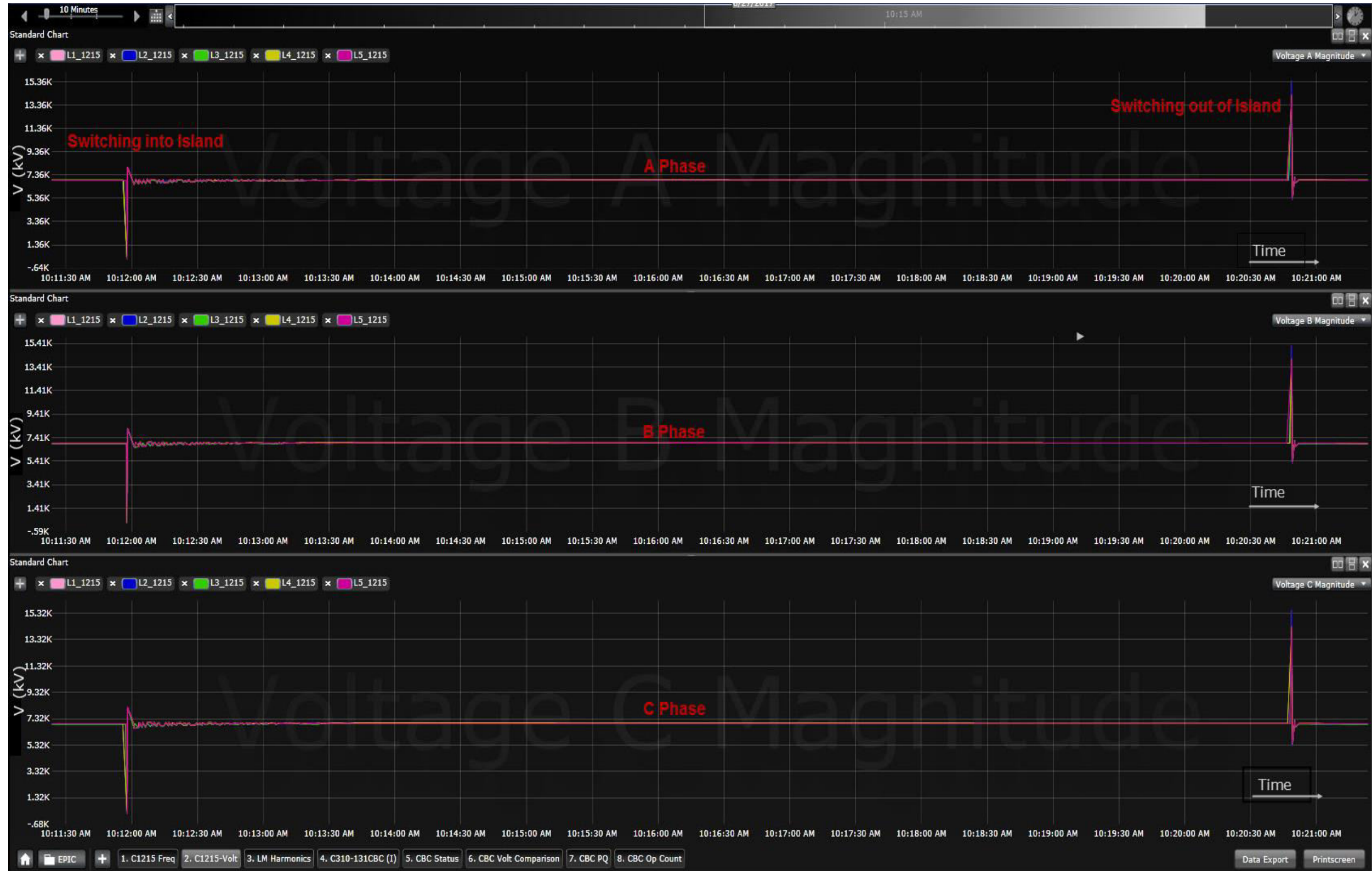
Figure 9.7: Voltage Monitoring in Island 3
