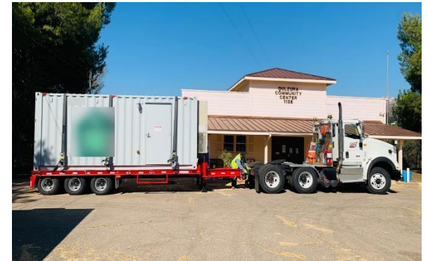
MBESS at community resource center
