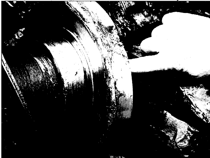
Figure 5. Arc mark on C Phase 230 kV bushing bottom plate which connects the draw lead sleeve to the shield assembly
