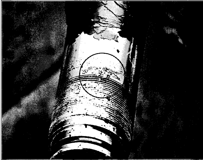
Figure 8. Arc mark on the C Phase 230 kV bushing draw-lead conduit above the bottom plate threading
