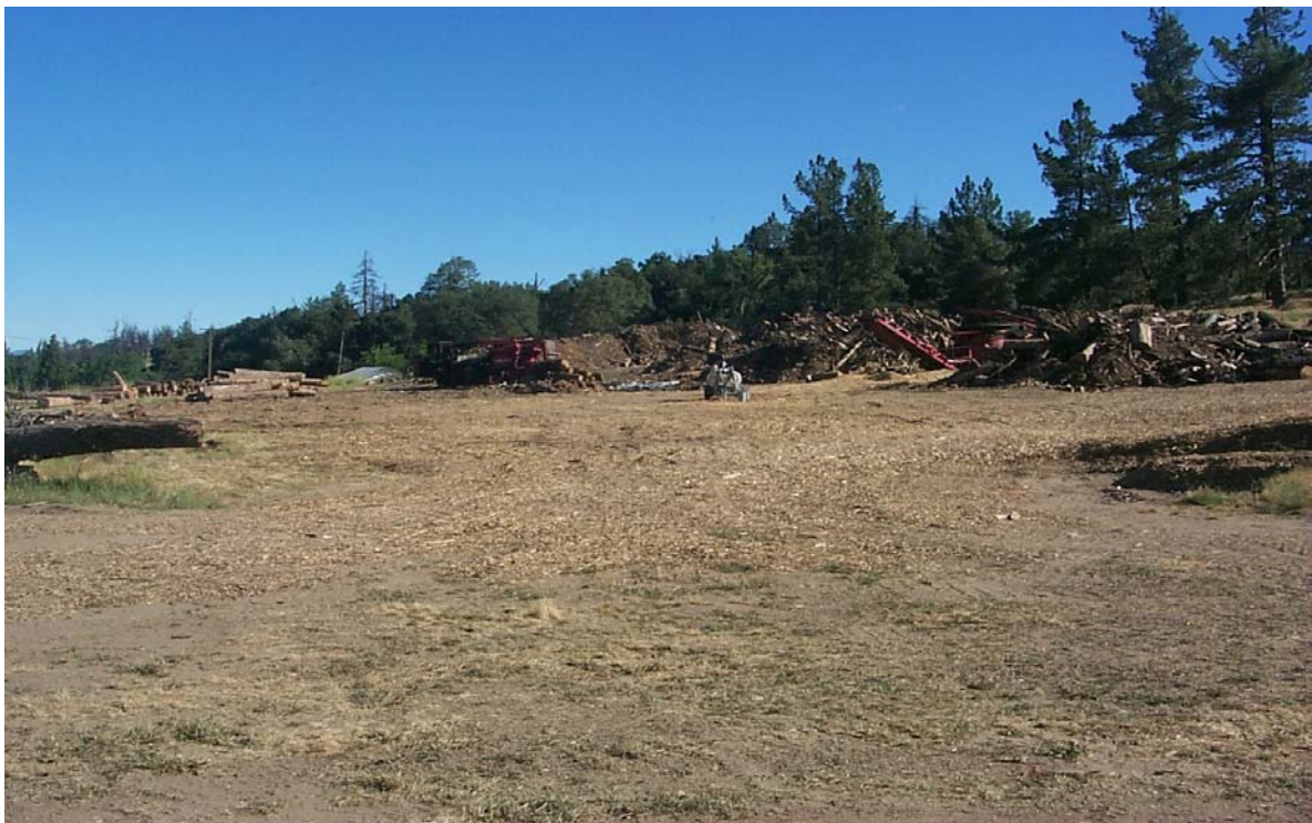
Figure 4.0 Dead Tree Grinding Operations
