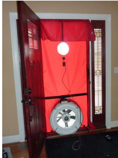
Blower door testing of units
