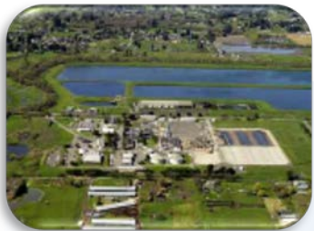
Waste Water Treatment Plant
