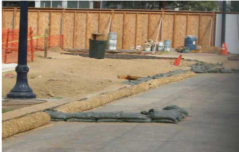
Gravel bags and fiber rolls used as perimeter sediment controls.
