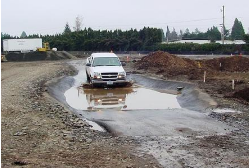
Drive through wheel wash before exiting a site.
