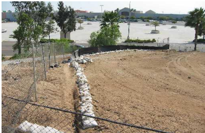
Gravel bags used as perimeter control.
