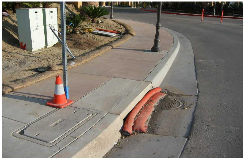
Inlet protection that blocks flow, preventing non-storm water discharges from entering drain.
