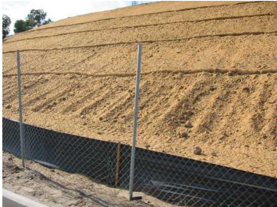
Silt fence installed with at least a 3 foot setback from the toe of an erodible slope. Note that use is combined with fiber rolls and serves as perimeter control.
