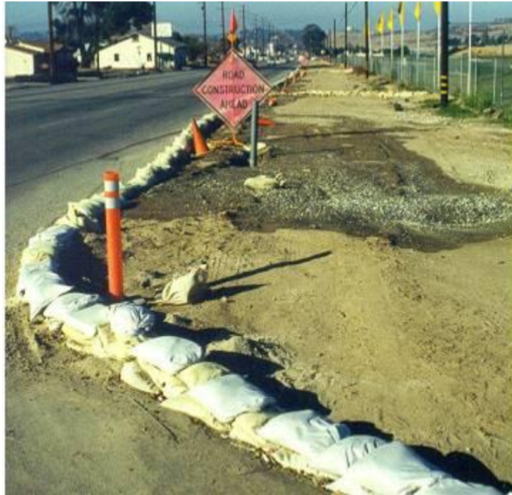
Sand bags used as perimeter control.
