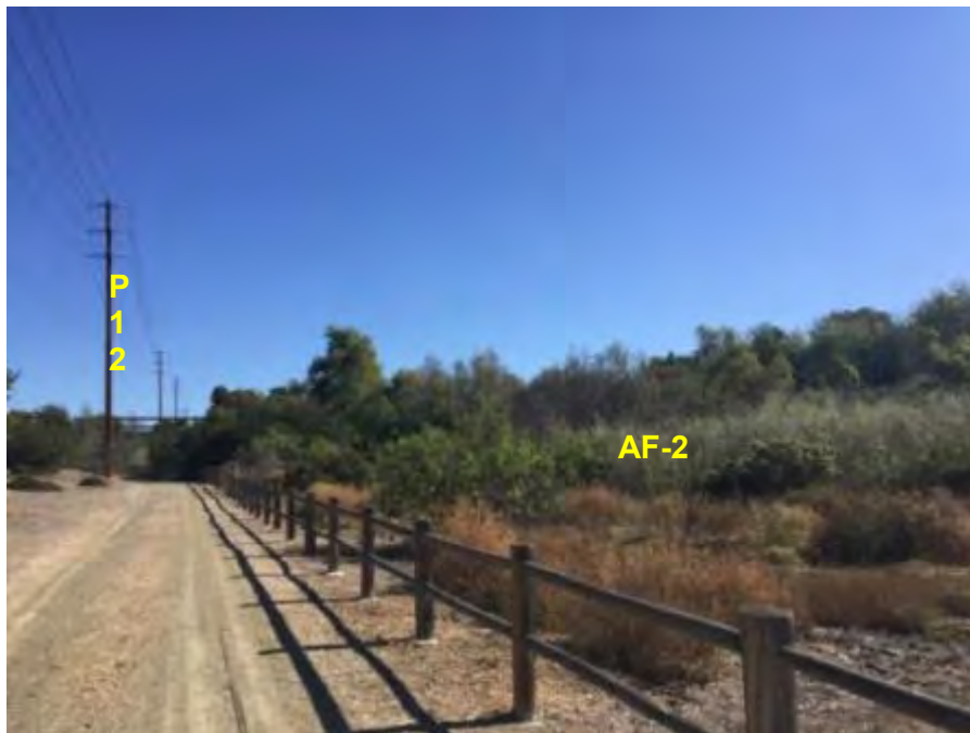
Photograph 10. View of pole P12, located north of arroyo willow-mule fat woodland and spiny rush marsh within AF-2. Access to P12 will be from an existing dirt access road, located between AF-2 and P12. No impacts to AF-2 are anticipated. Photo taken November 13, 2015 facing southeast.
