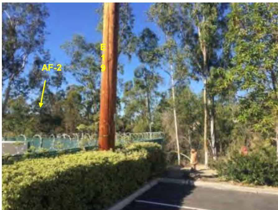
Photograph 28. View of pole E19, located south of arroyo willow-mule fat woodland and cattail marshes within AF-2. Access to pole will be from an existing paved parking lot. No impacts to AF-2 are anticipated. Photo taken November 13, 2015 facing northeast.
