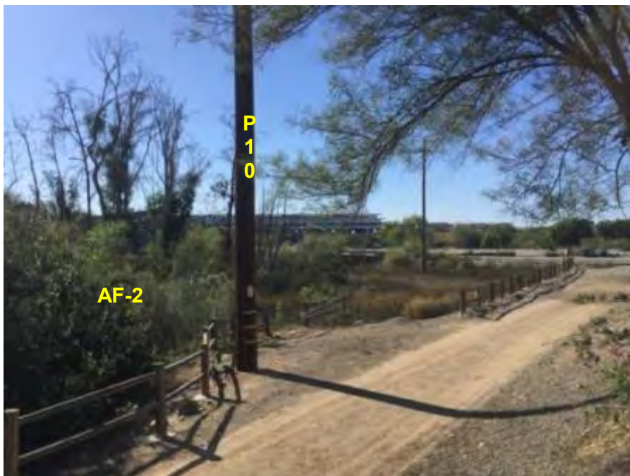
Photograph 8. View of pole P10, located north of arroyo willow-mule fat woodland and spiny rush marsh within AF-2. Access to P10 will be from an existing dirt access road immediately north of the pole. No impacts to AF-2 are anticipated. Photo taken November 13, 2015 facing southwest.
