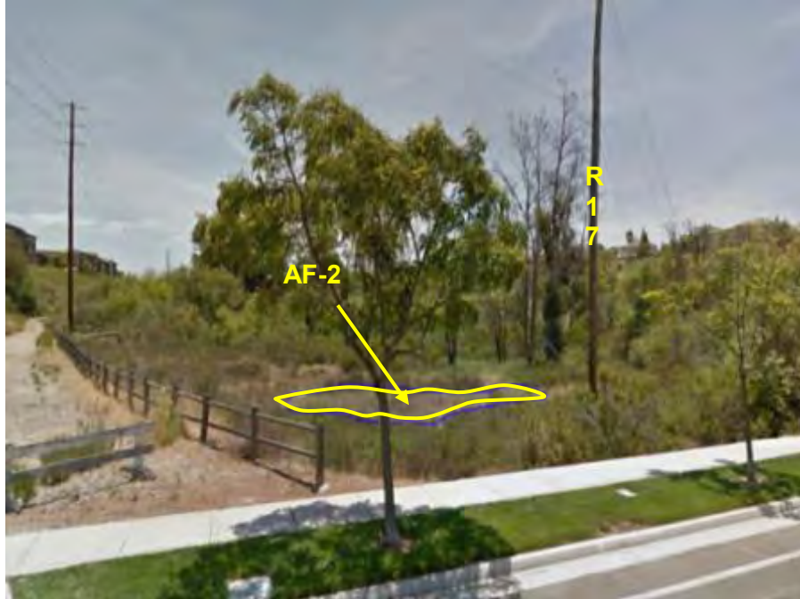
Photograph 5. View of stub pole R17 which is to be removed from service, is located in upland vegetation west of salt grass flats (in yellow) within AF-2. R17 will be accessed by foot travel from the access road and no impacts to AF-2 are anticipated. Photo taken September 9, 2015 facing southeast.
