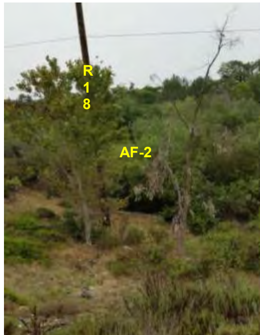
Photograph 12. Another view of pole R18, located within AF-2. This pole will be removed from service and will be accessed by foot travel. The crew will park along the existing access road, walk in, cut pole, and remove. No impacts to AF-2 are anticipated. Photo taken November 13, 2015 facing south from access road to pole.
