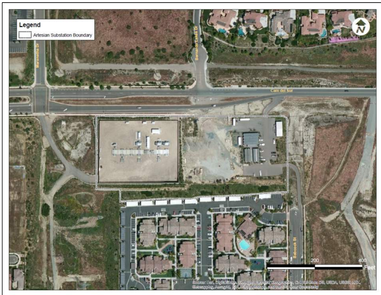
Figure 1-1 Aerial view of the existing Substation and adjacent properties.
