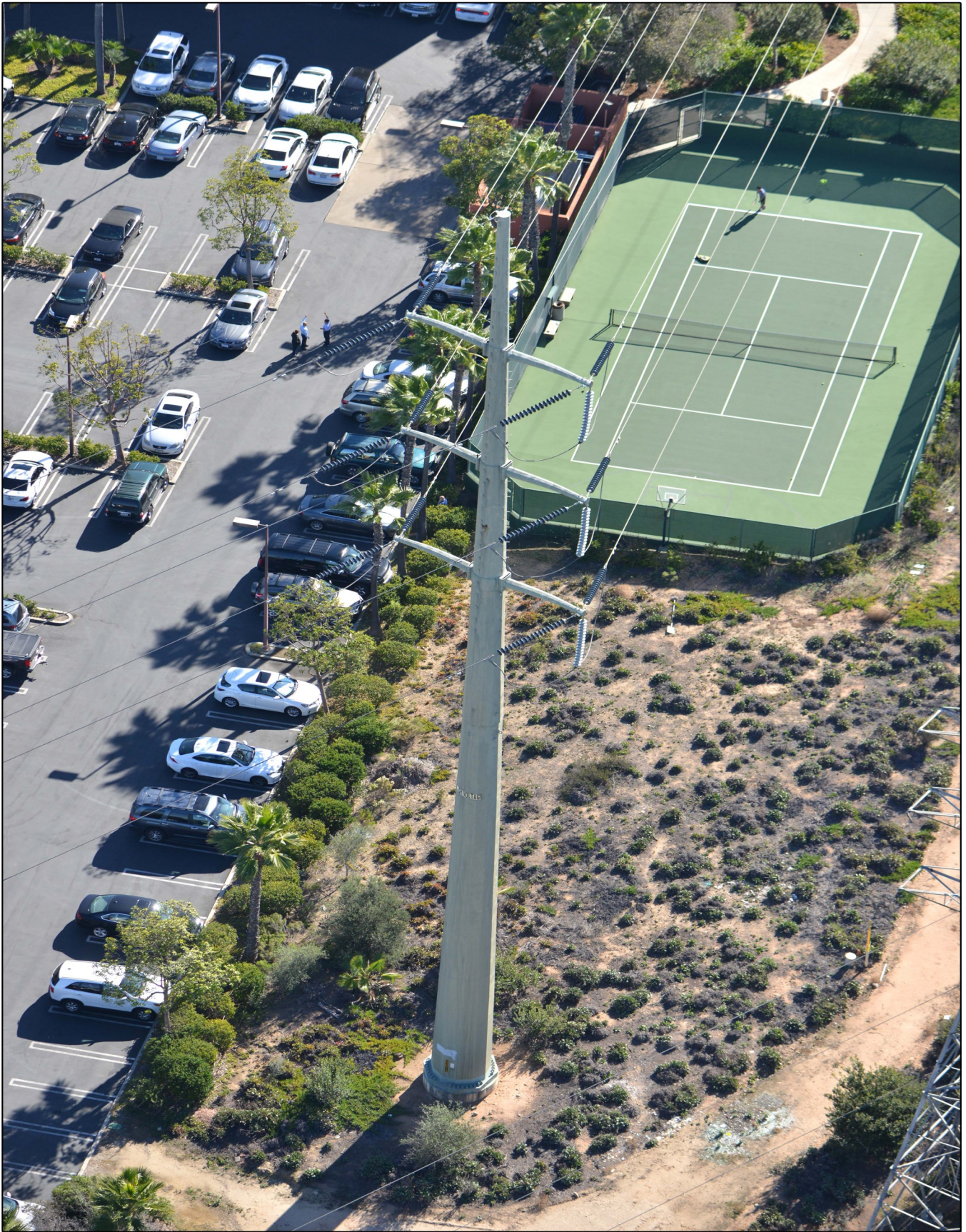
Typical 230kV Double-Circuit Dead-end Dull Galvanized Steel Tubular Pole
